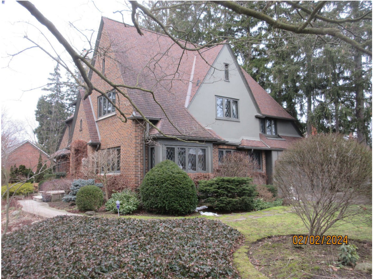
Image 7: View of the south (left) and east (right) facades of the house at 244 Base Line Road East.
