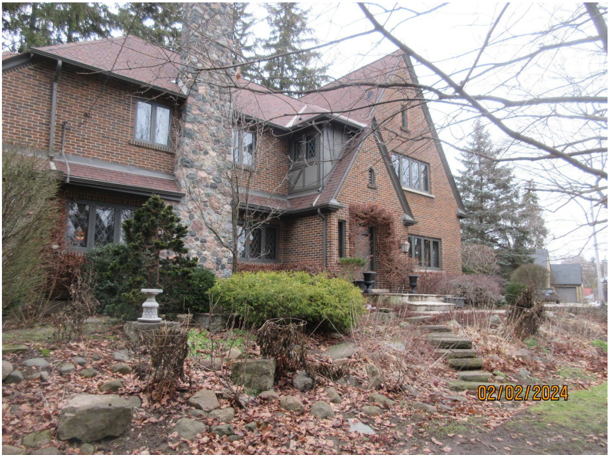
Image 4: View looking northeast towards the house at 244 Base Line Road East.
