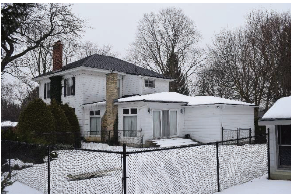
Plate 27: Hip roof addition, looking northeast
