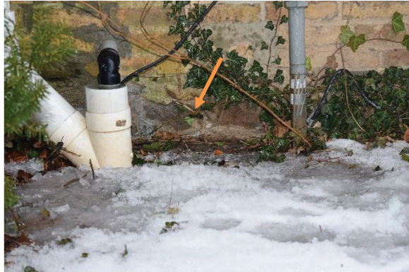
Plate 16: Visible stone section of foundation (denoted by arrow), looking west
