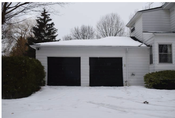
Plate 30: Garage and shed roof addition, looking east
