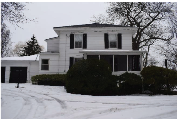
Plate 29: East elevation, looking west
