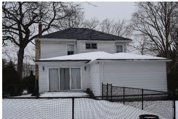
Plate 26: South elevation, looking north
