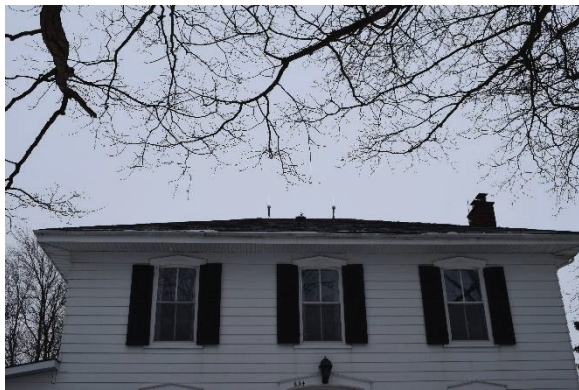
Plate 18: Second storey windows, looking south
