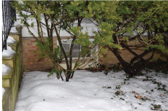
Plate 22: Basement window, looking south
