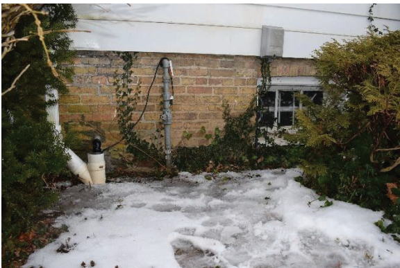
Plate 25: Basement window, looking east
