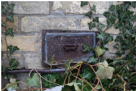
Plate 28: Clean out door, looking east
