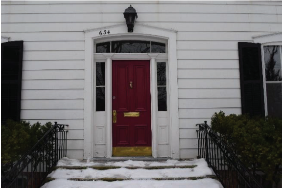
Plate 21: Main entrance details, looking south
