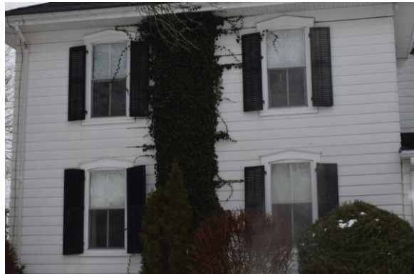
Plate 24: Window details, looking east
