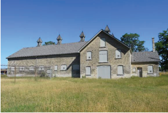
Photo 1: Horse Stable looking northwest
