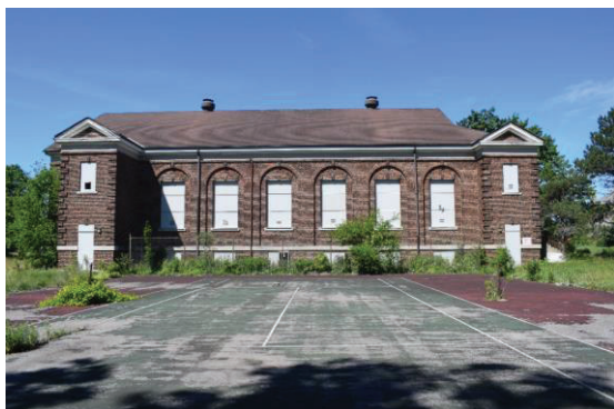
Photo 20: Recreation Hall east elevation looking west
