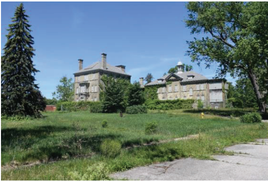
Photo 10: Infirmery south elevation looking northwest
