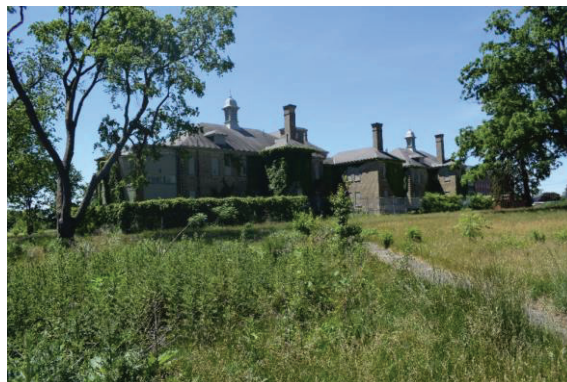
Photo 15: Infirmary north (rear) elevation looking southwest
