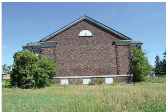
Photo 21: Recreation Hall south elevation looking north
