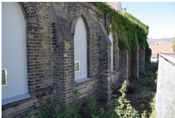
Photo 7: Chapel of Hope south elevation looking east
