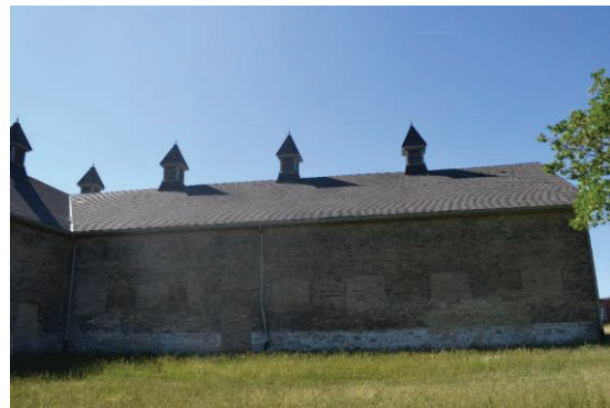
Photo 4: Horse Stable looking south
