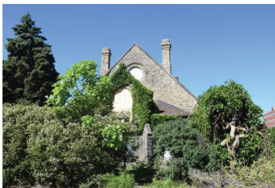
Photo 9: Chapel of Hope rear (east) elevation looking west
