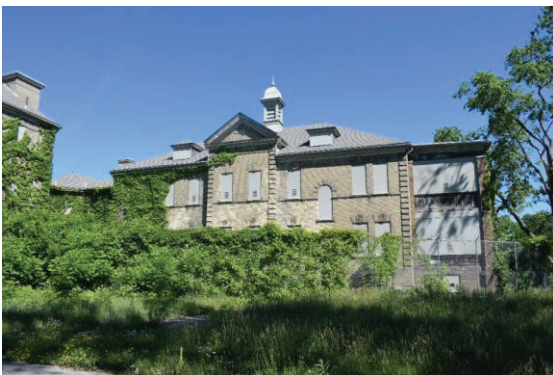
Photo 12: Infirmery south elevation of east wing looking north
