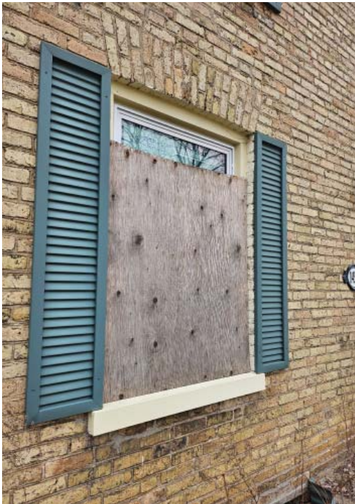
Windows with shutters and voussoirs (not original)
