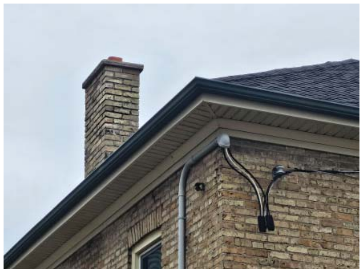
Original chimney with low pitched hipped roof
