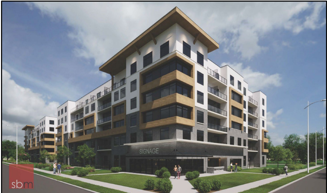
Figure 5: Rendering (facing southwest from the intersection of Royal Magnolia Avenue and Campbell Street North)
