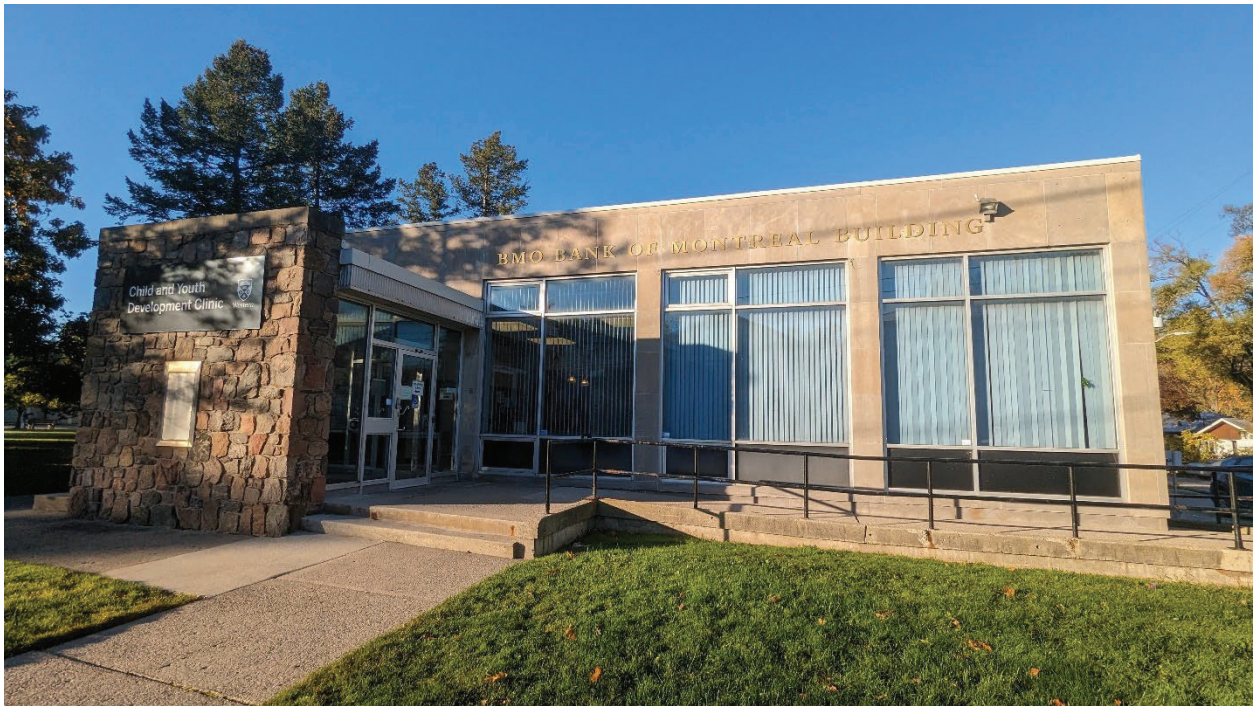
Photos 55 & 56: (above) View of east (front) elevation of the building looking north-west; (below) View of east elevation of building looking westwards and towards vestibule entrance and feature stone wall (MHBC, 2023).
