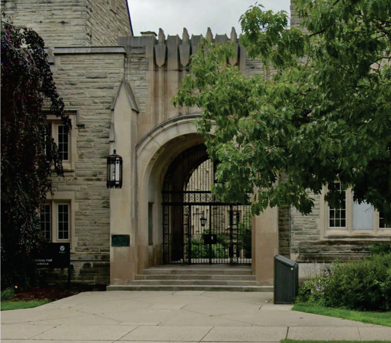
Photo 33: Main entryway of Medway Hall (MHBC, 2023).
