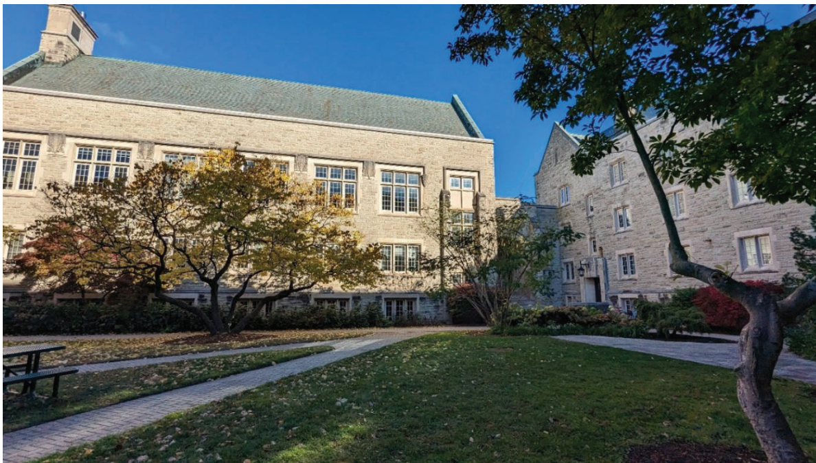
Photos 44-46: (above) View of front (north) elevation from the internal courtyard looking towards the front entryway; (below) View of internal courtyard looking towards front entryway (MHBC, 2023).
