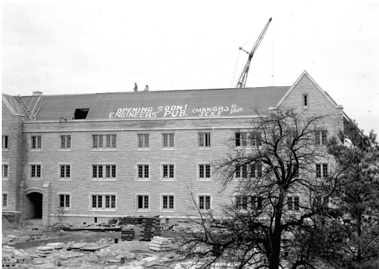
Photo 19: Photograph from 1959 of the construction of Medway Hall (Source: Free Press Collection of Negatives/ Western Archives).
