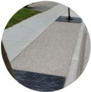
Decorative Paving Treatment
