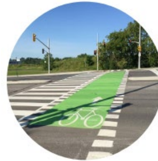
Designated Bike Crossing with Coloured Pavement Marking
