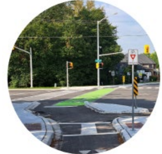
Safe Bike Lane Intersection
