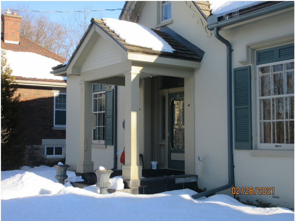
Image 19: Photograph showing the simple form of the painted wood porch over the front doorway with a shingle gable roof, supported by a plain frieze and boxed piers with simple capital and base details (2021).
