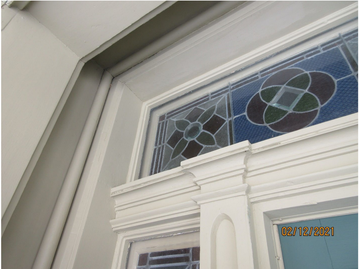
Image 17: Detail photograph showing the entablature of the doorway with pilaster, as well as a detail of the stained glass transom (2021).
