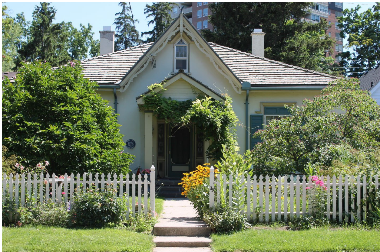
Image 2: Photograph of Carfrae Cottage on July 21, 2015.
