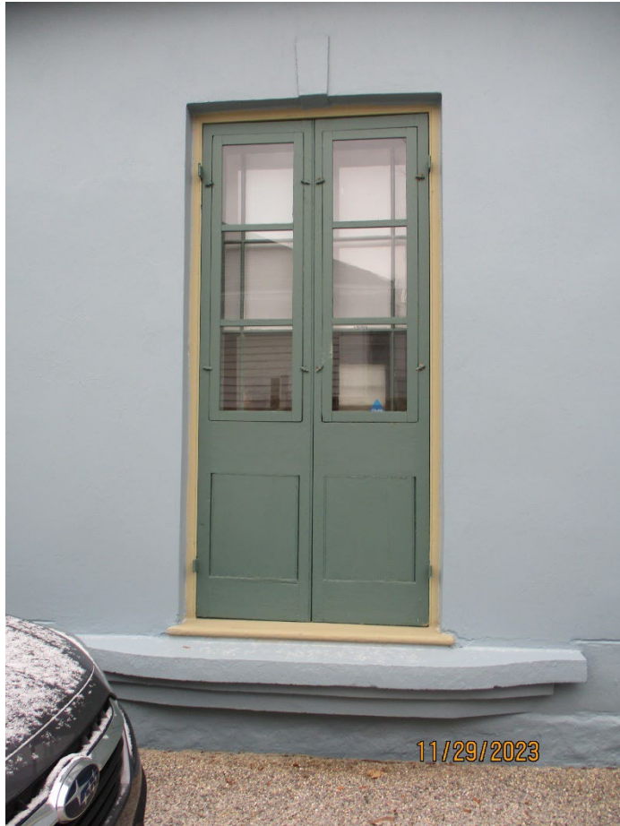
Image 29: Photograph of the painted wood French doors and painted wood storm doors in the opening of the west façade, sill as an indication of the former verandah of Carfrae Cottage (2023).
