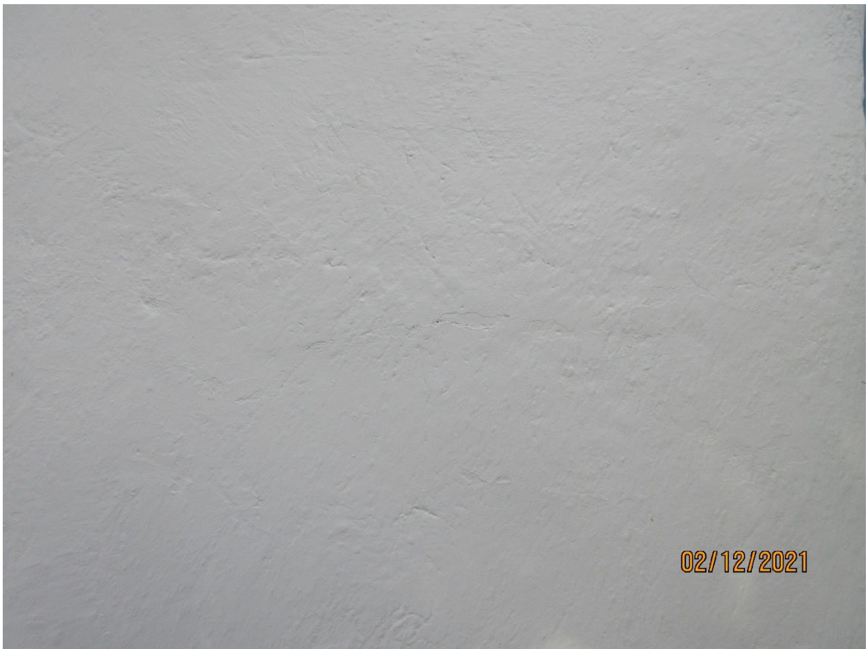
Image 14: Photograph, showing a representative example, of the traditional stucco parging (cementitious smooth textured exterior 'stucco' finish) over the double brick construction of Carfrae Cottage (2021).
