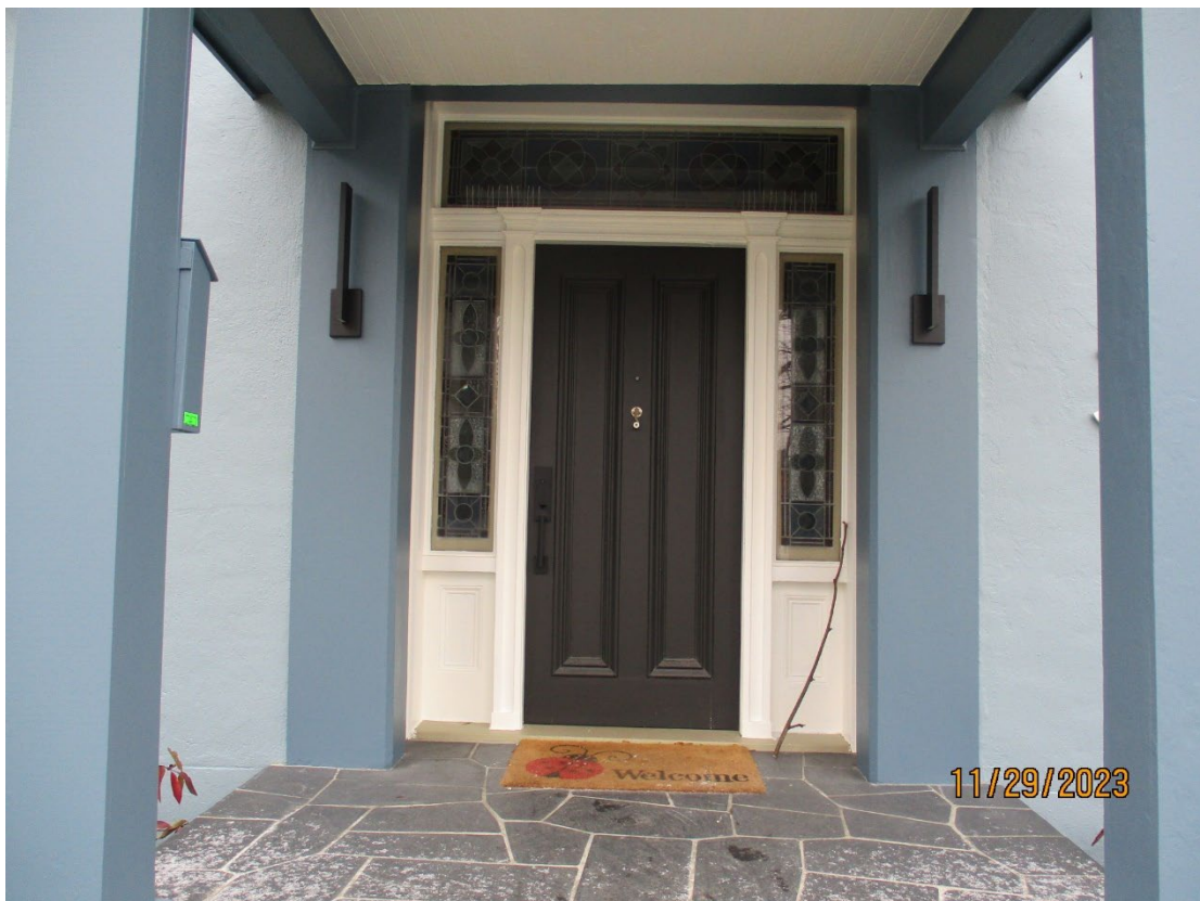
Image 16: Photograph showing the front doorway with single leaf, painted wood door with two long panels, set in a rectangular opening with rectangular sidelights to both sides, a panelled dado below, and a rectangular transom. The sidelights and transom feature reconstructed leaded and stained glass in repetitive geometric patterns with coloured and textured glass. The doorway is recessed in the façade with a plain reveal. The door opening is framed by pilasters, with entablature supporting the architectural framework of the doorway (2023).
