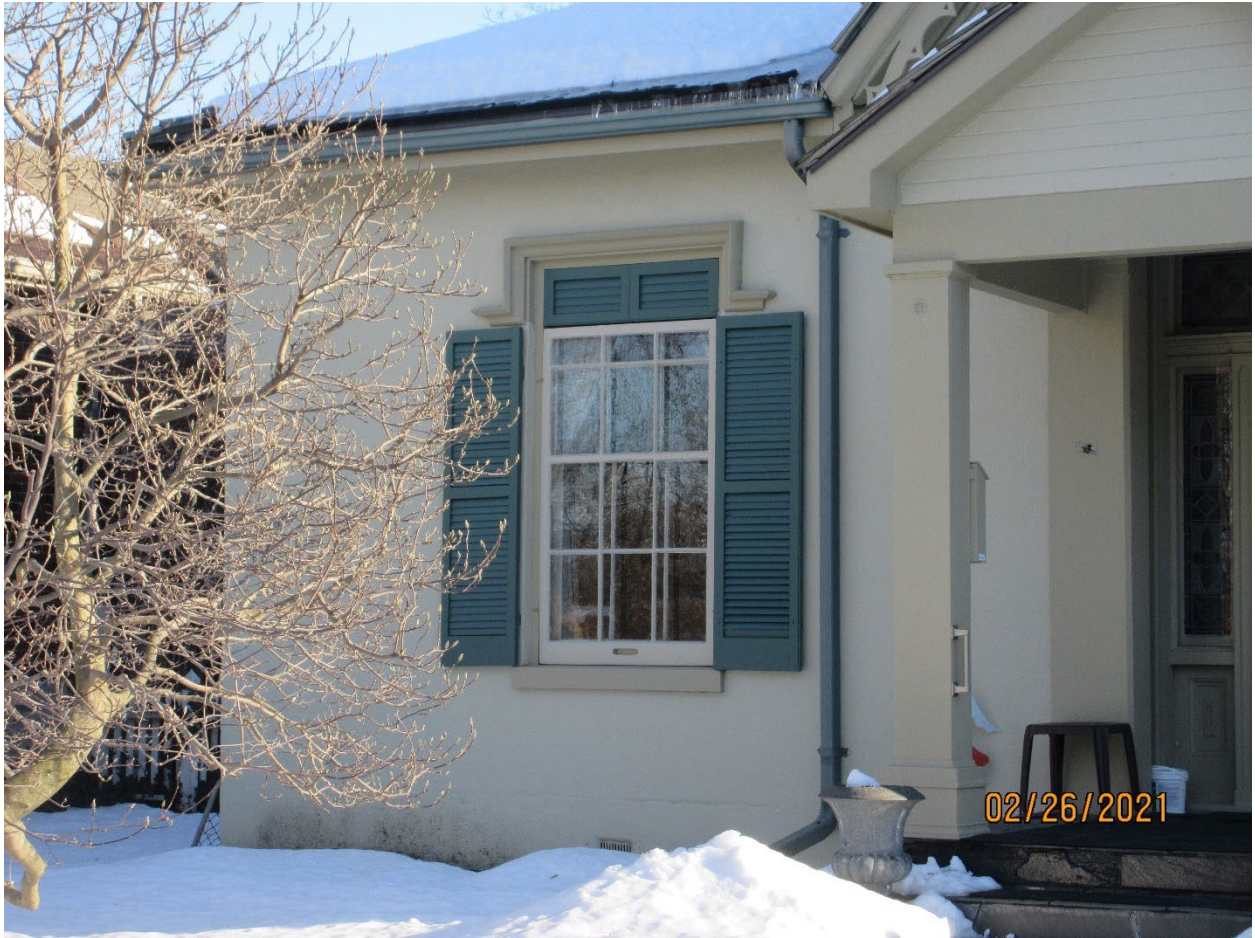
Image 21: View showing the easterly window, sill, and label on the front (north) façade of Carfrae Cottage (2021).
