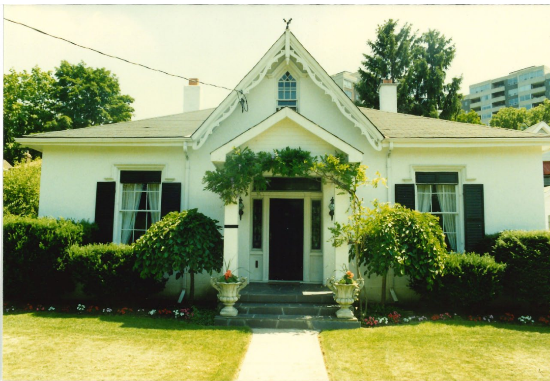
Image 1: Photograph of Carfrae Cottage in 1988 at the time of its designation pursuant to Section 29 of the Ontario Heritage Act.
