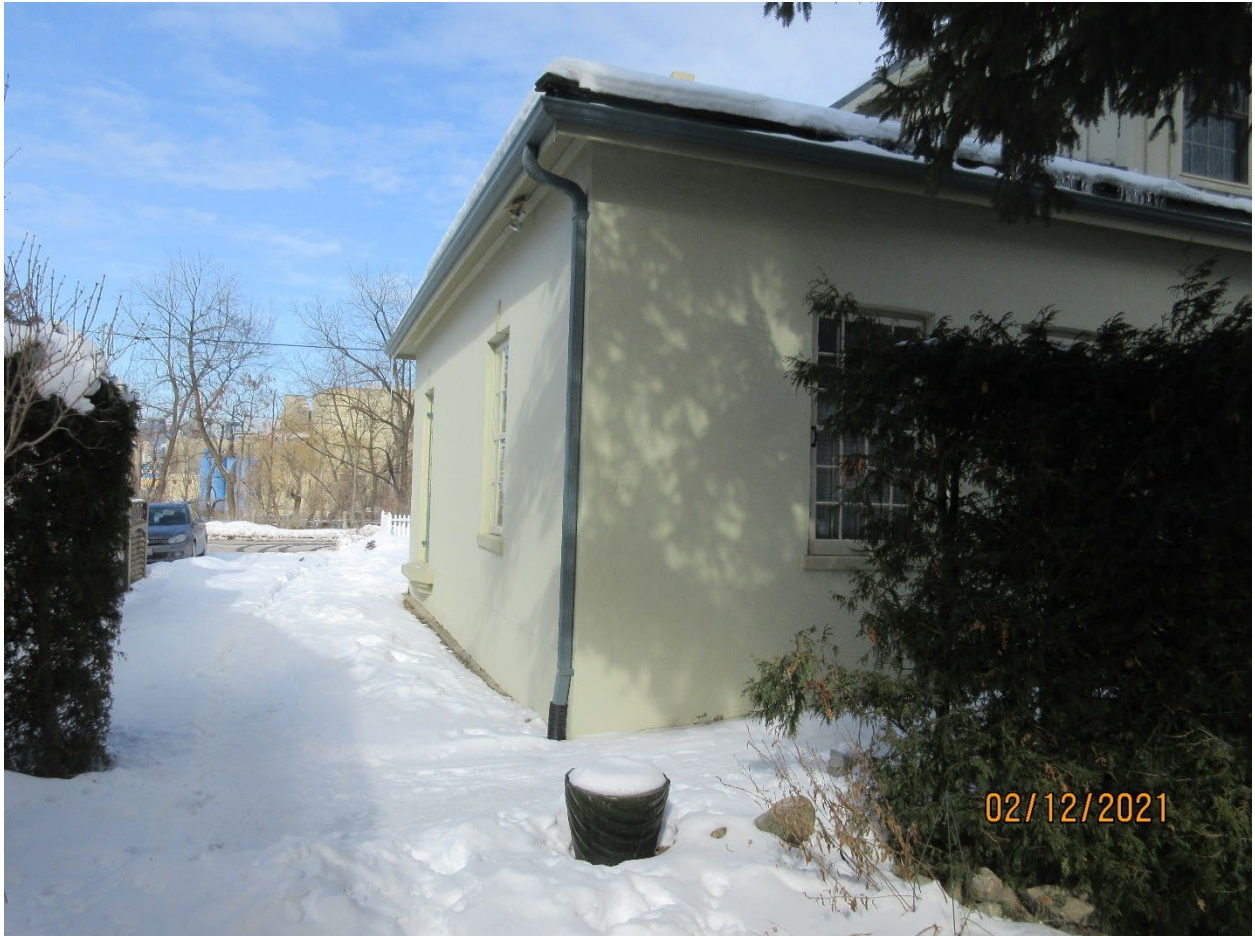
Image 27: View of the west and south facades of Carfrae Cottage, and showing the driveway along the westerly property boundary (2021).
