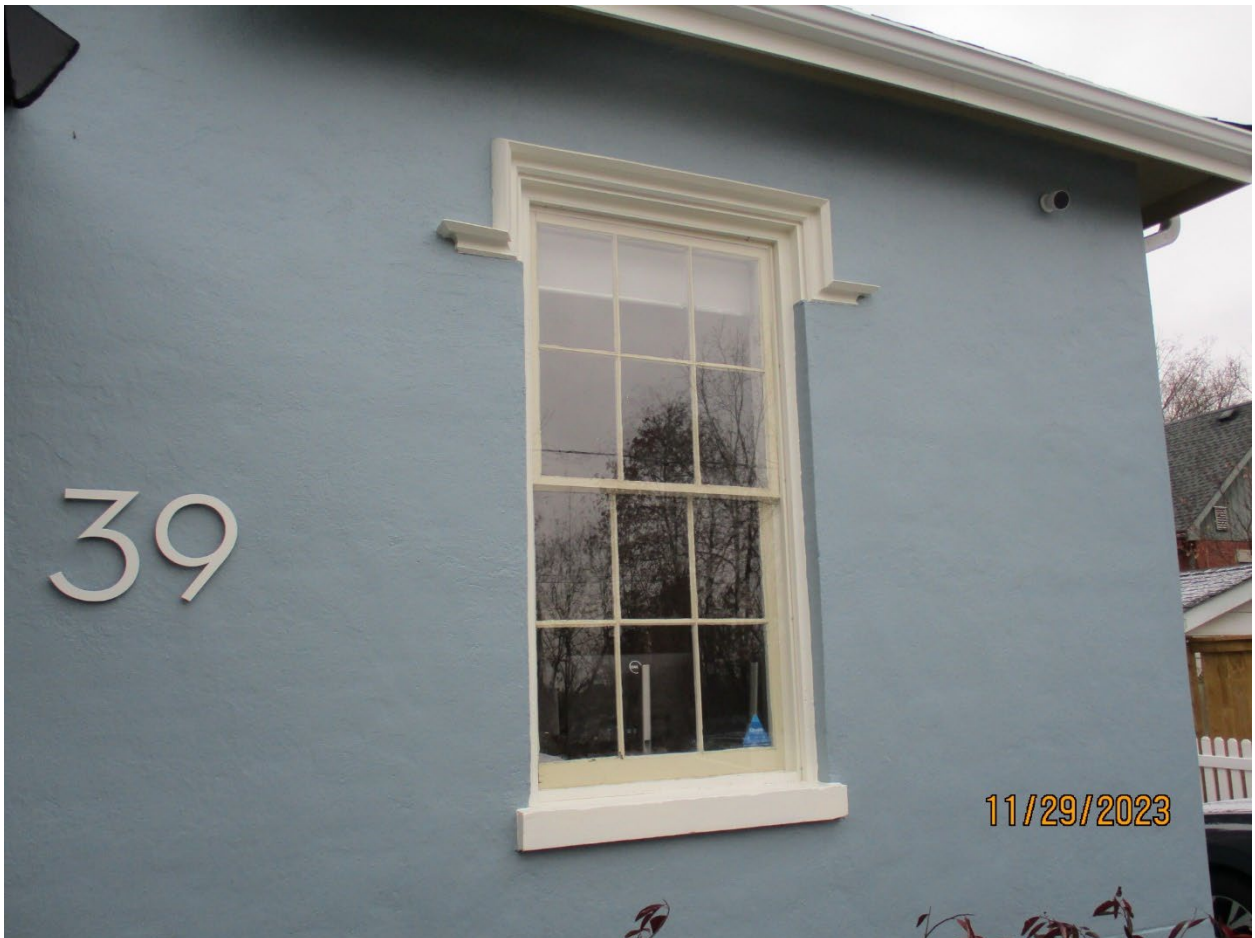
Image 24: Photograph showing the westerly front window, label, and sill of the front (north) façade of Carfrae Cottage (2023).
