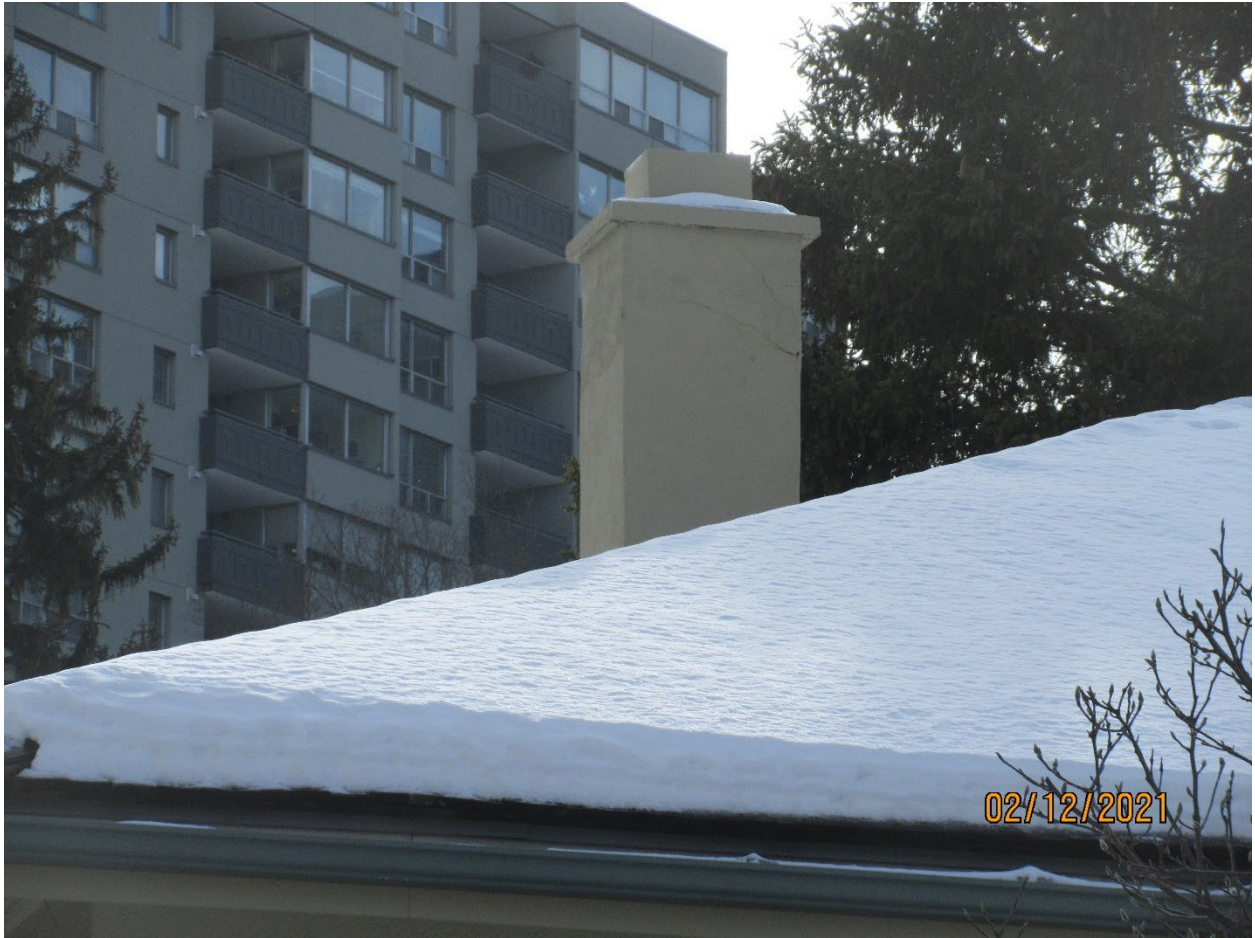
Image 11: Photograph of the east chimney, as seen from Carfrae Street (2021).
