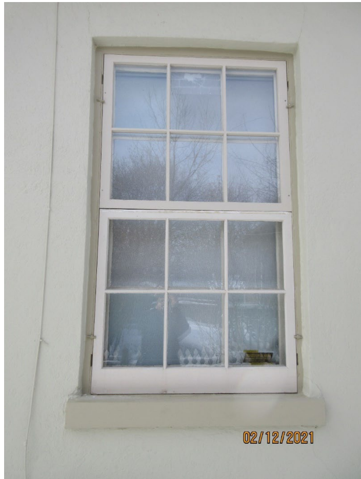
Image 32: Photograph of the six-over-six painted wood window on east façade (2021).
