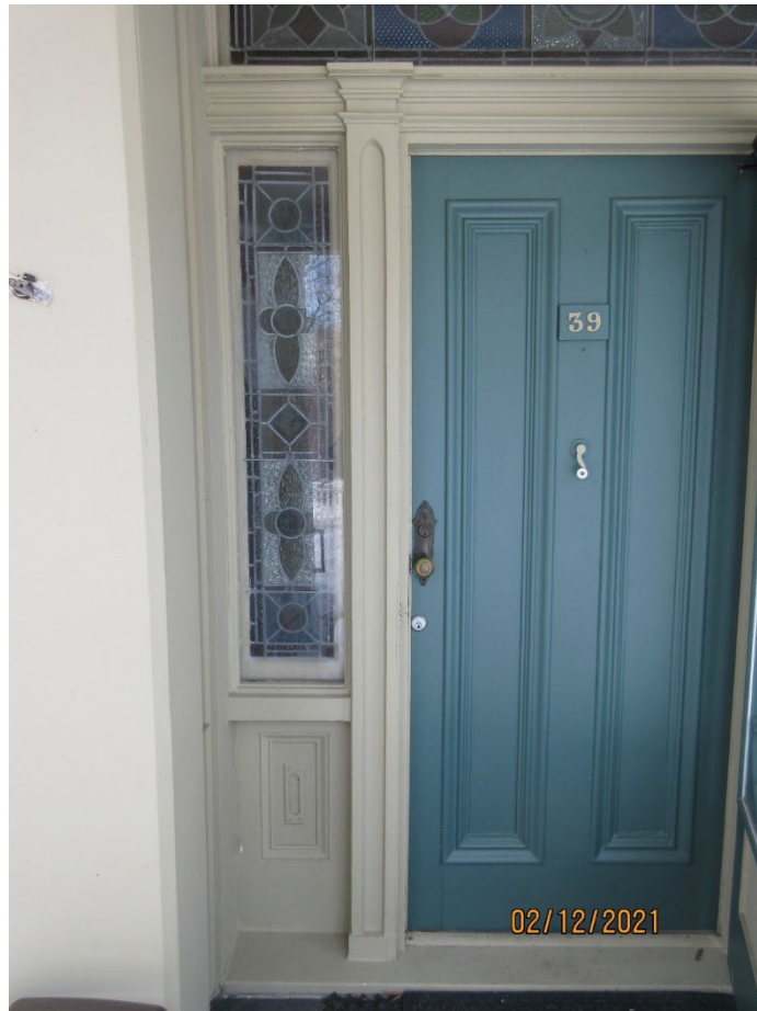
Image 15: Photograph showing the front doorway with single leaf, painted wood door with two long panels, set in a rectangular opening with rectangular sidelights to both sides, a panelled dado below, and a rectangular transom. The sidelights and transom feature reconstructed leaded and stained glass in repetitive geometric patterns with coloured and textured glass. The doorway is recessed in the façade with a plain reveal. The door opening is framed by pilasters, with entablature supporting the architectural framework of the doorway (2021).
