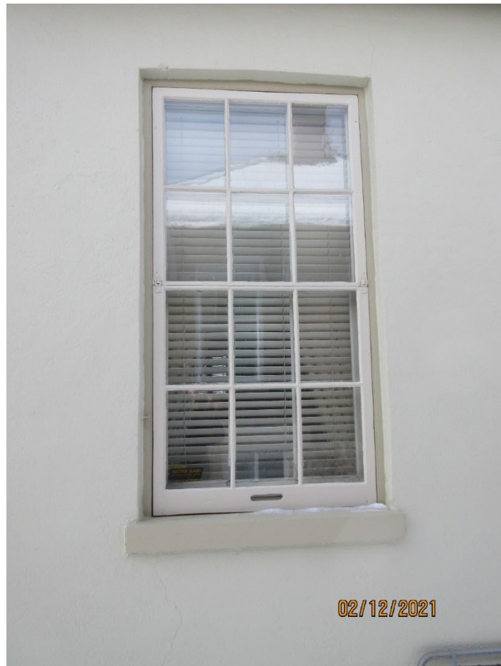
Image 34: Photograph of the six-over-six double hung painted window on east façade and wood sill on the east façade (2021).
