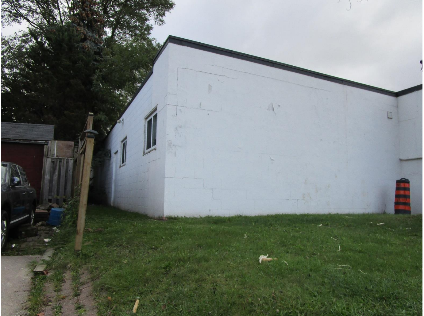
Photograph 3: North elevation and a view of the rear extension, looking southwest (AECOM 2021)
