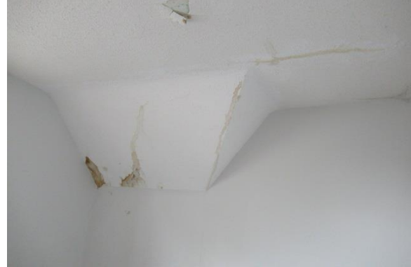
Photo Exhibit No. 22 30 Wellington – large cracks in the ceiling, along with water damage from the roof.
