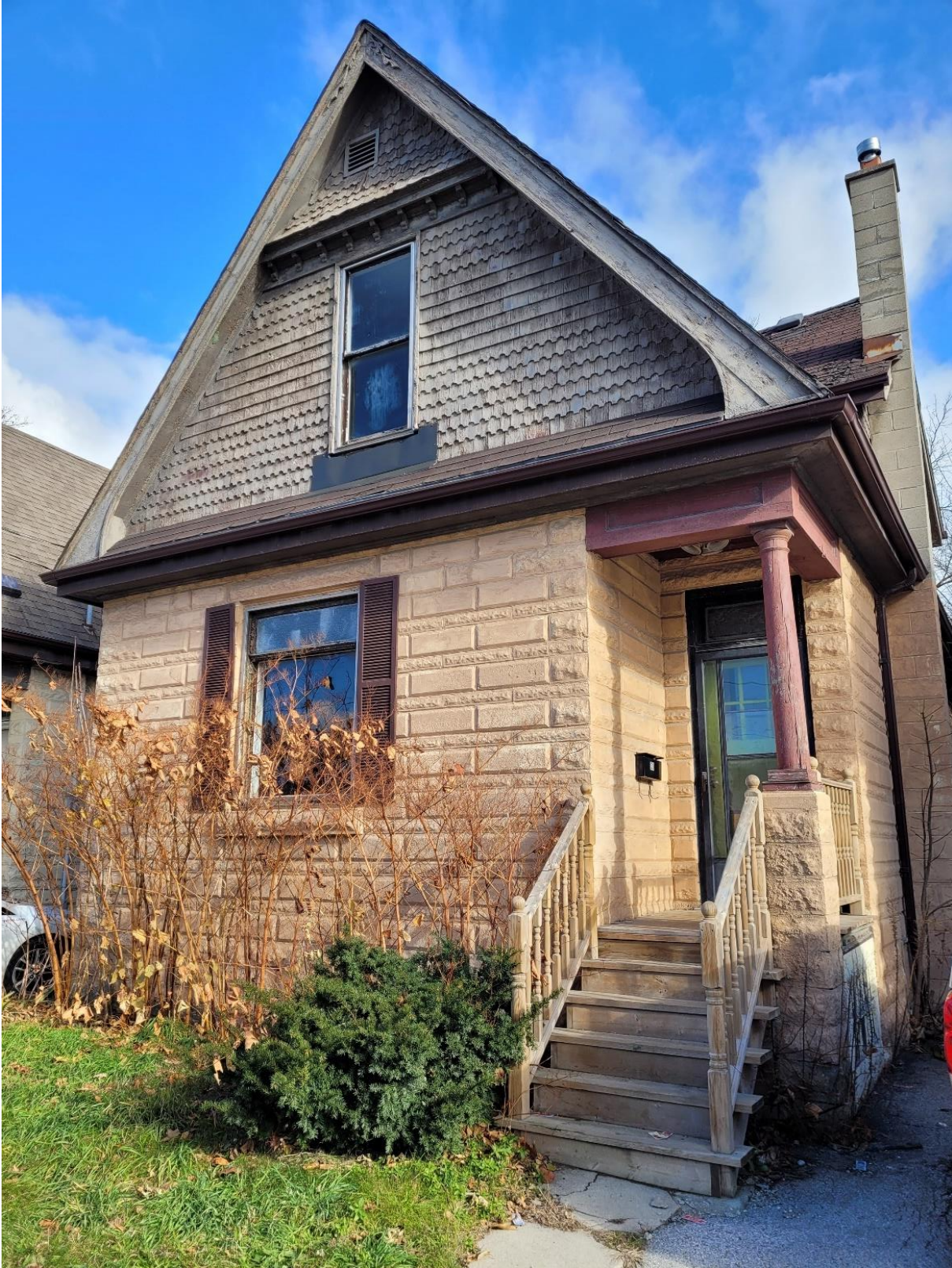
Photograph 9: View of the one-and-a-half storey building located at 30 Wellington Road (AECOM 2021)
