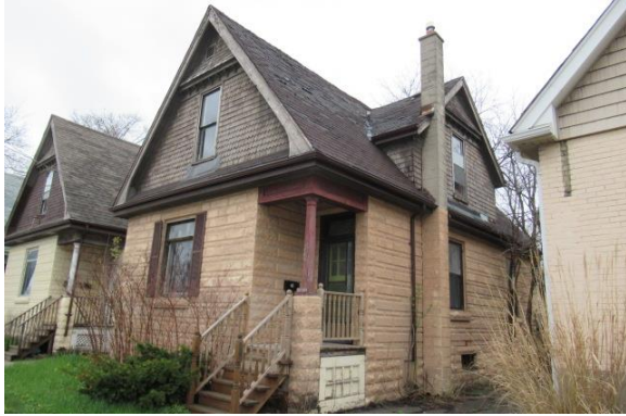
Photo Exhibit No. 13 30 Wellington – overall of front elevation.
