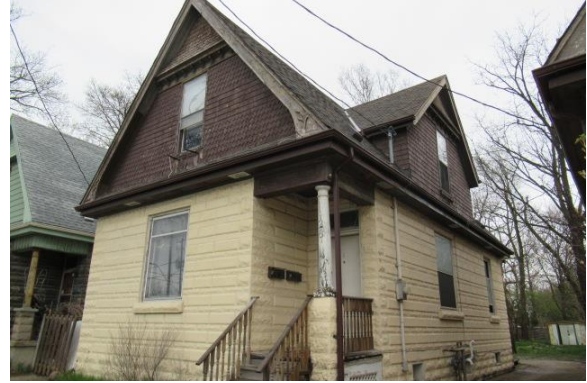
Photo Exhibit No. 4 28 Wellington – front elevation.
