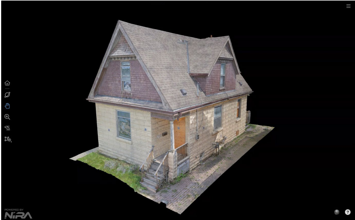
Image 11: Screen capture showing 3D documentation of the house on the property at 28 Wellington Road (SkyDeploy, received August 10, 2023).
