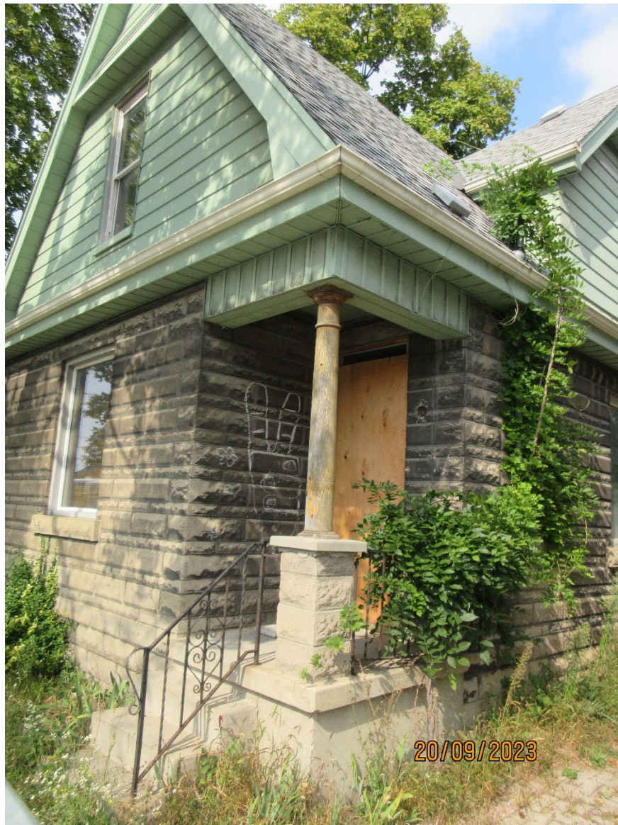
Image 4: Photograph showing part of the building on the subject property at 26 Wellington Road (taken September 20, 2023).
