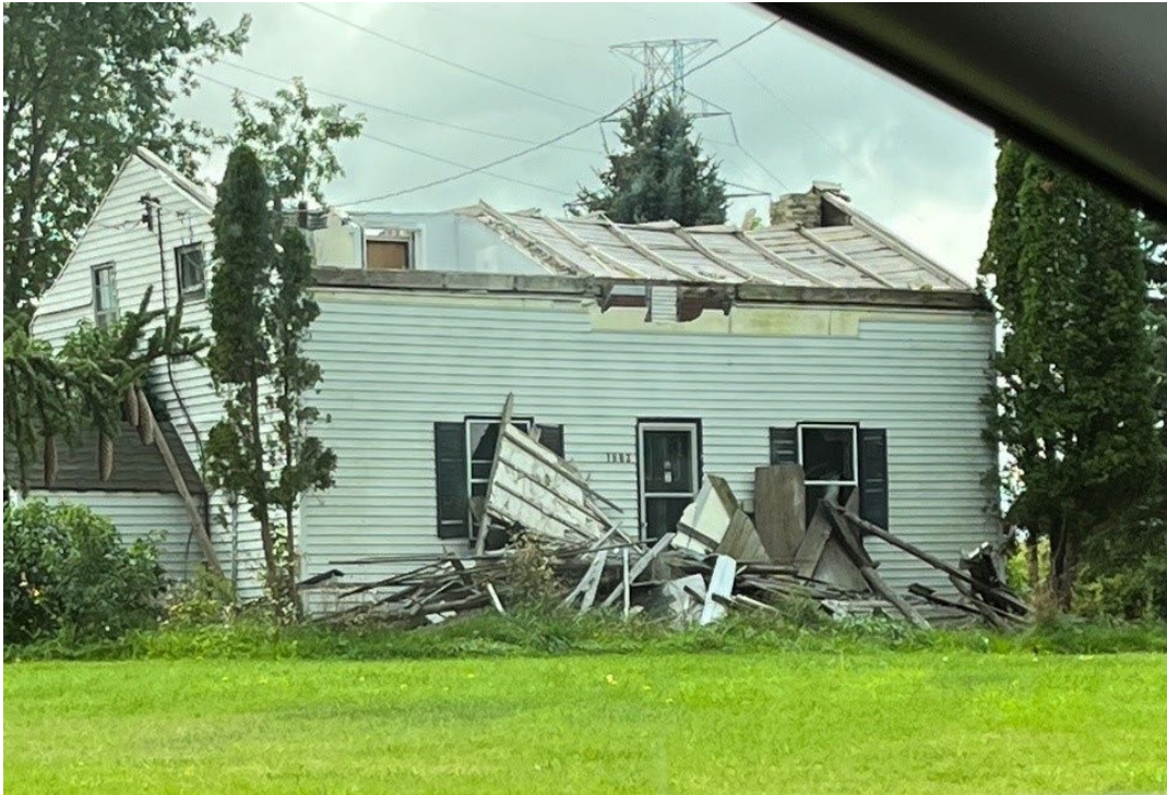
City Initiated Demolition
