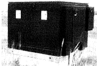
Pad mounted switchgear
