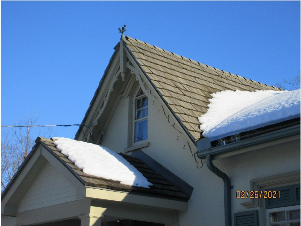
*Image 25: View of the central gable dormer on the front (north) facade of Carfrae Cottage with a primitive Gothic pointed wood window. The decorative wood bargeboard of the central gable dormer is also shown, as well as the Scotch thistle (2021).*
