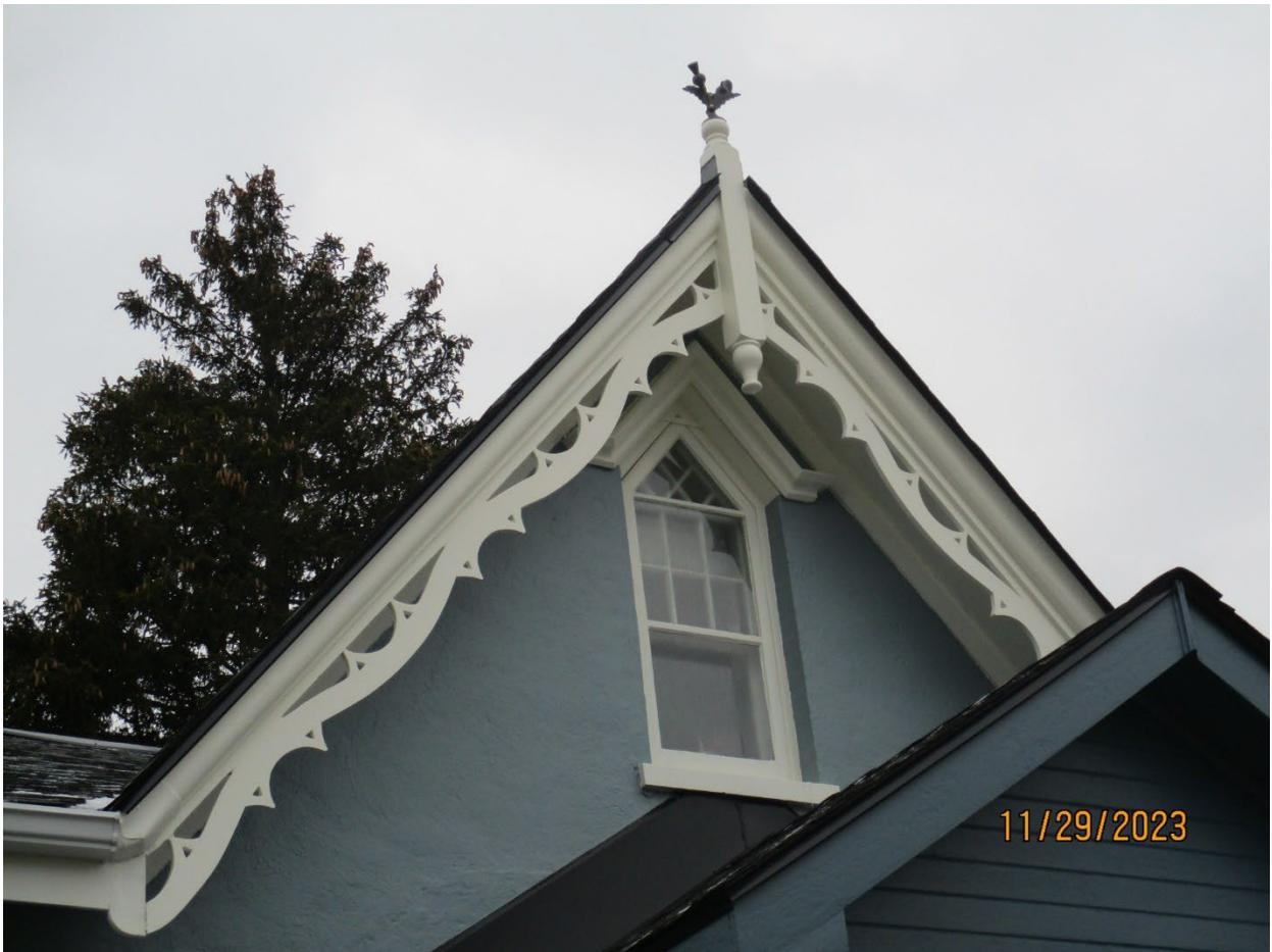
*Image 26: View of the central gable dormer on the front (north) facade of Carfrae Cottage with a primitive Gothic pointed wood window. The decorative wood bargeboard of the central gable dormer is also shown, as well as the Scotch thistle (2023).*
