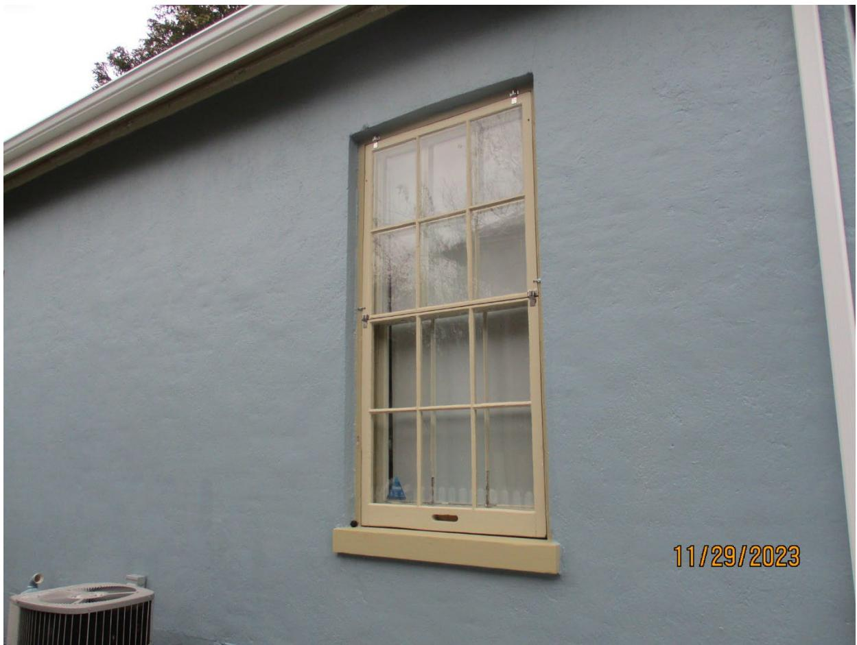
*Image 35: Photograph of the six-over-six double hung painted window on east façade and wood sill on the east façade (2023).*
