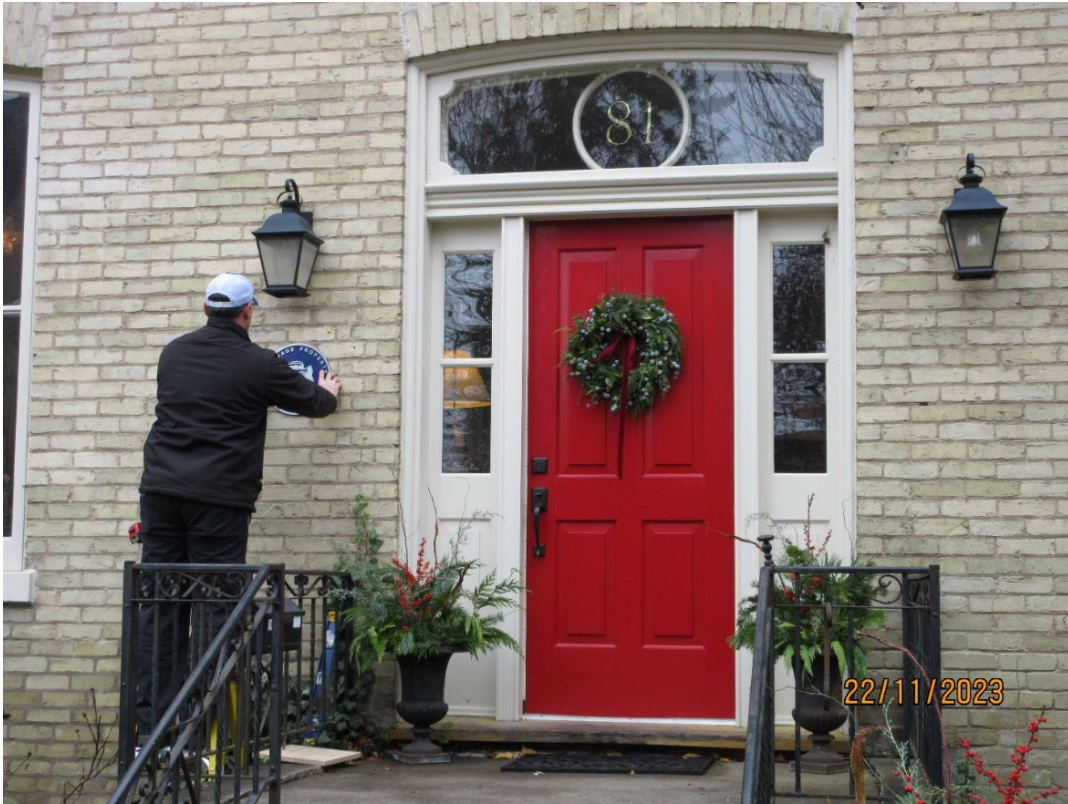
Image 1: Installation of the blue City of London Heritage Property plaque on the heritage designated property at 81 Wilson Avenue on November 22, 2023.
