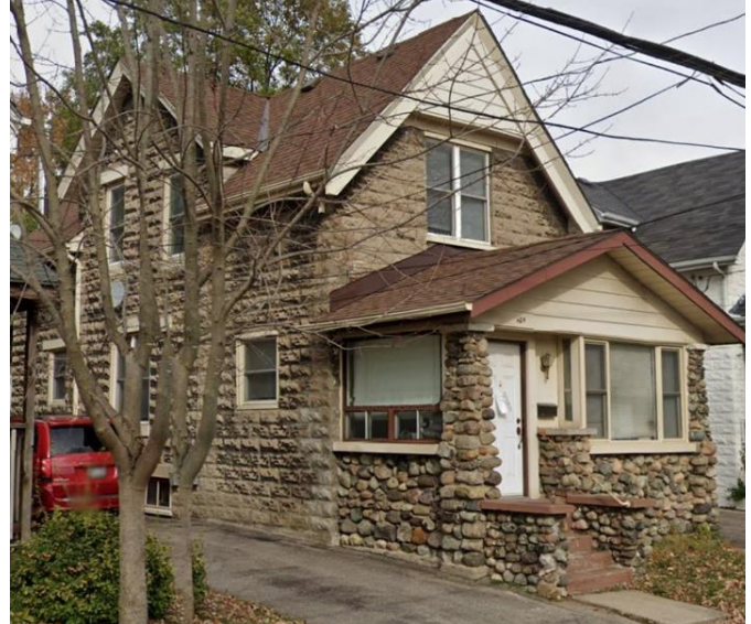
Image 5 924 Princess Avenue (Google Street View, 2020)
