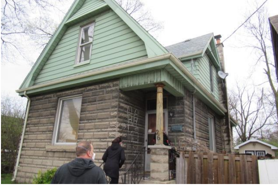
Photo Exhibit No. 1 26 Wellington – front elevation.
