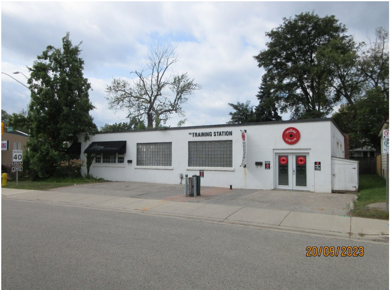
Image 2: Photograph of the south elevation of the building on the subject property at 16 Wellington Road (taken September 20, 2023).
