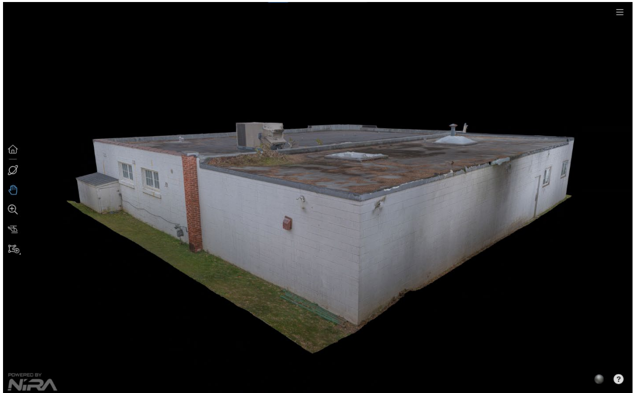
Image 10: Screen capture showing 3D documentation of the building on the property at 16 Wellington Road (SkyDeploy, received November 15, 2023).
