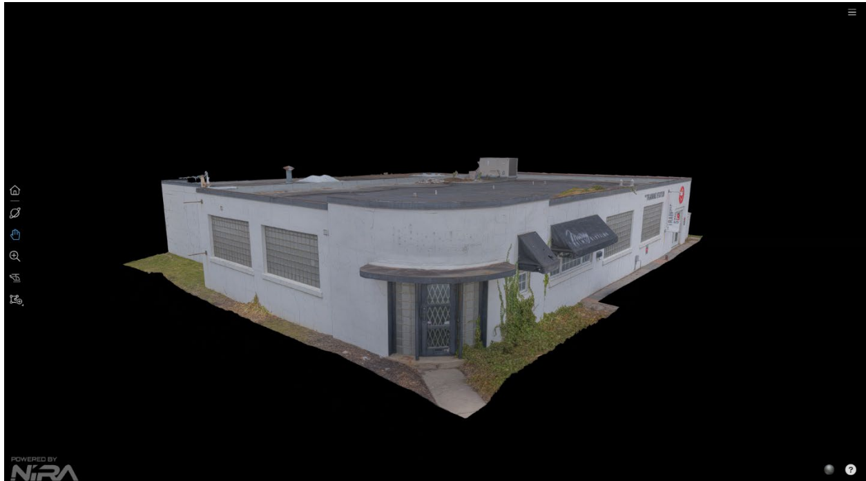
Image 9: Screen capture showing 3D documentation of the building on the property at 16 Wellington Road (SkyDeploy, received November 15, 2023).
