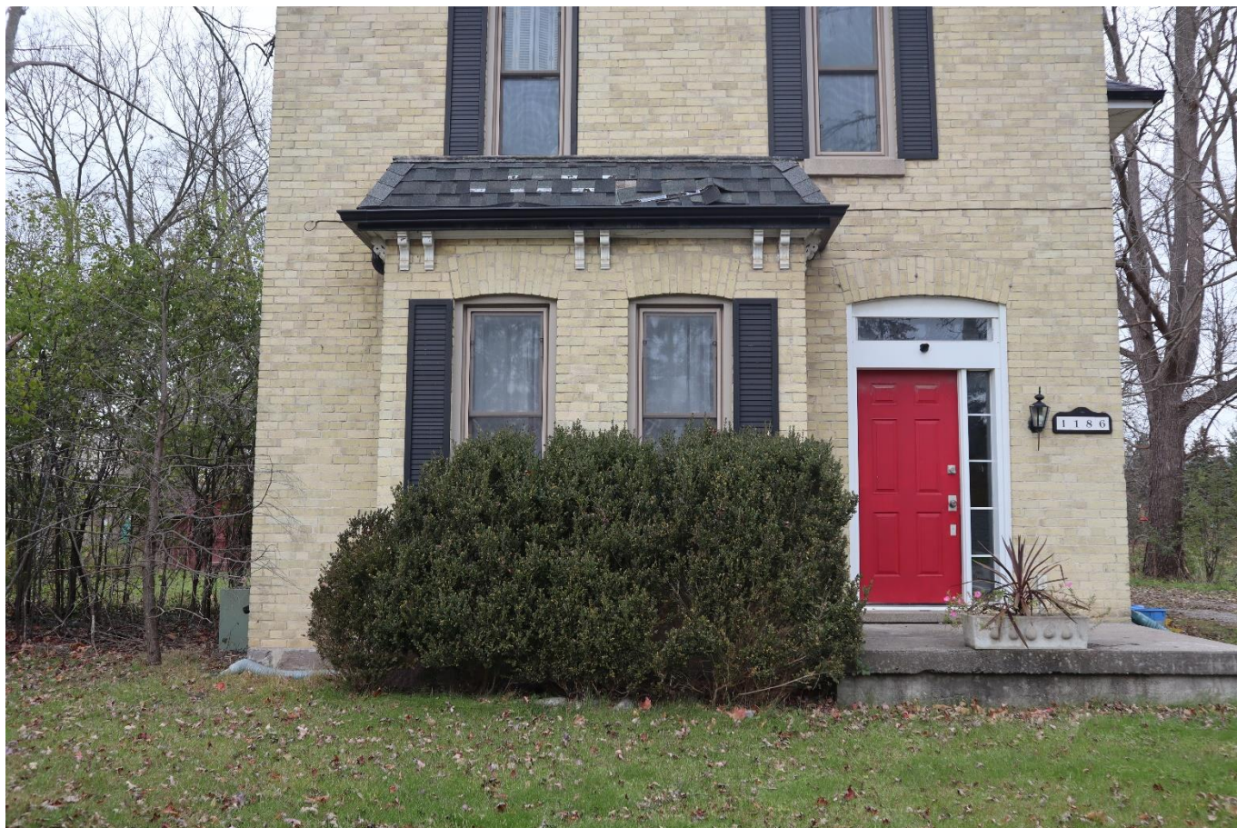
Photograph 12: View of the bay window and front entrance, looking north (AECOM 2021)
