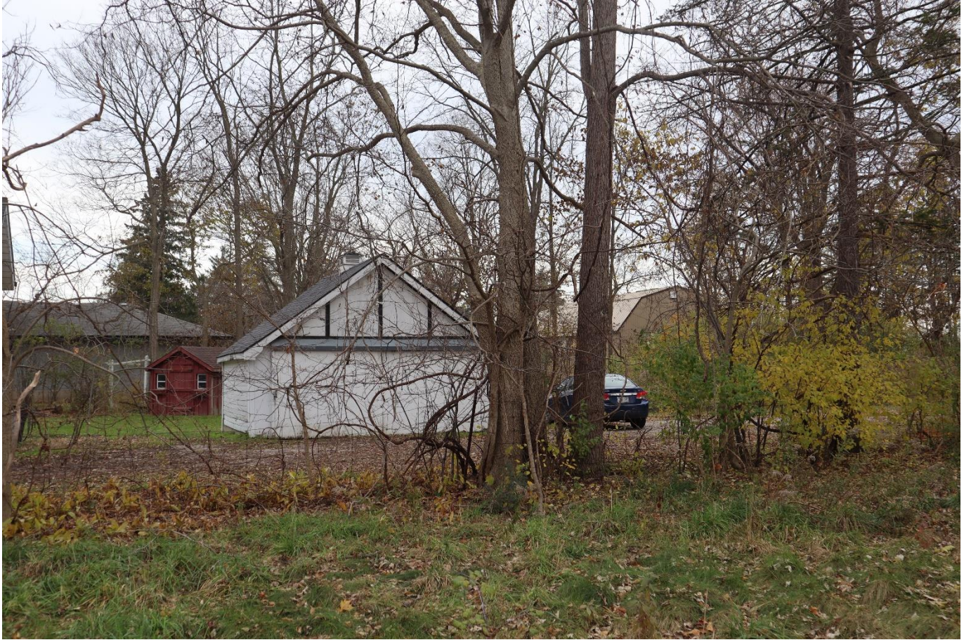
Photograph 18: View of the wood garage and shed, looking west (AECOM 2021)
