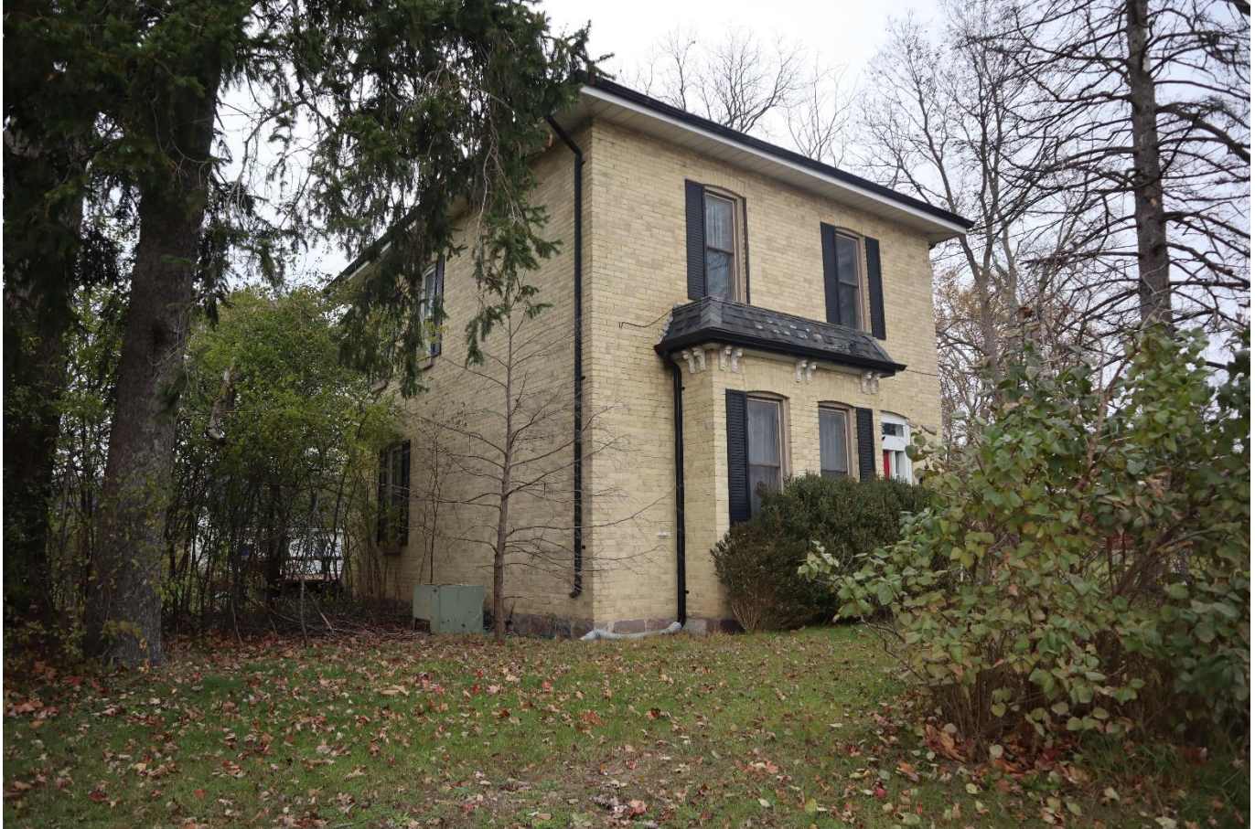
Photograph 15: View of the western elevation looking northeast (AECOM 2021)
