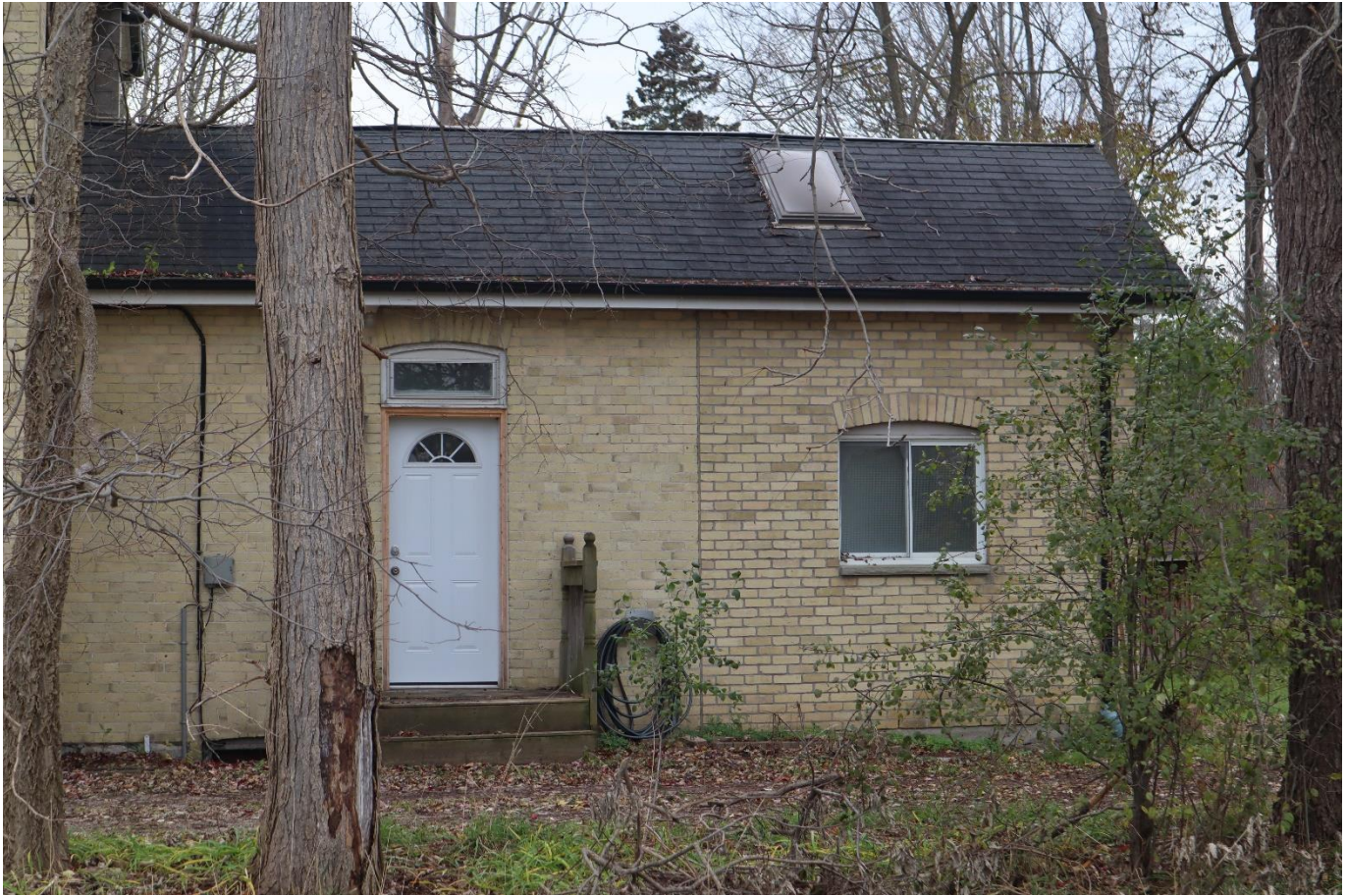
Photograph 14: View of kitchen tail and rear addition, looking west (AECOM 2021)
