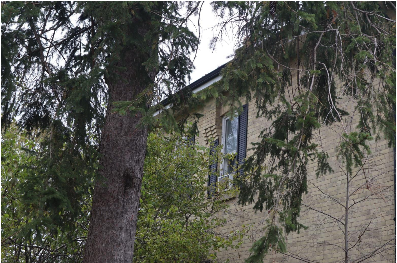
Photograph 16: View of the brick corbelling located on the western elevation, looking northeast (AECOM 2021)
