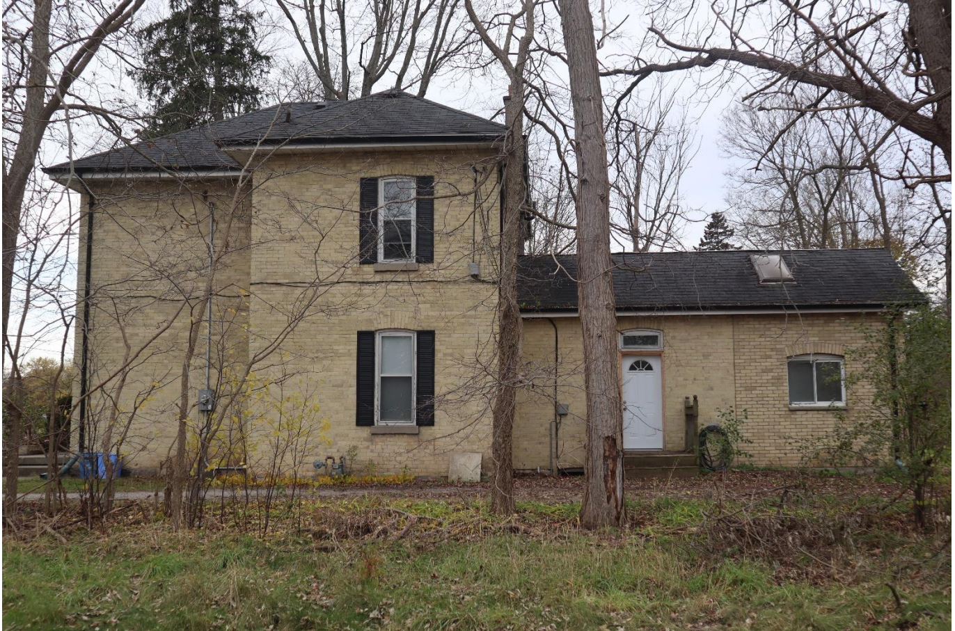
Photograph 13: View of the eastern elevation, looking west (AECOM 2021)
