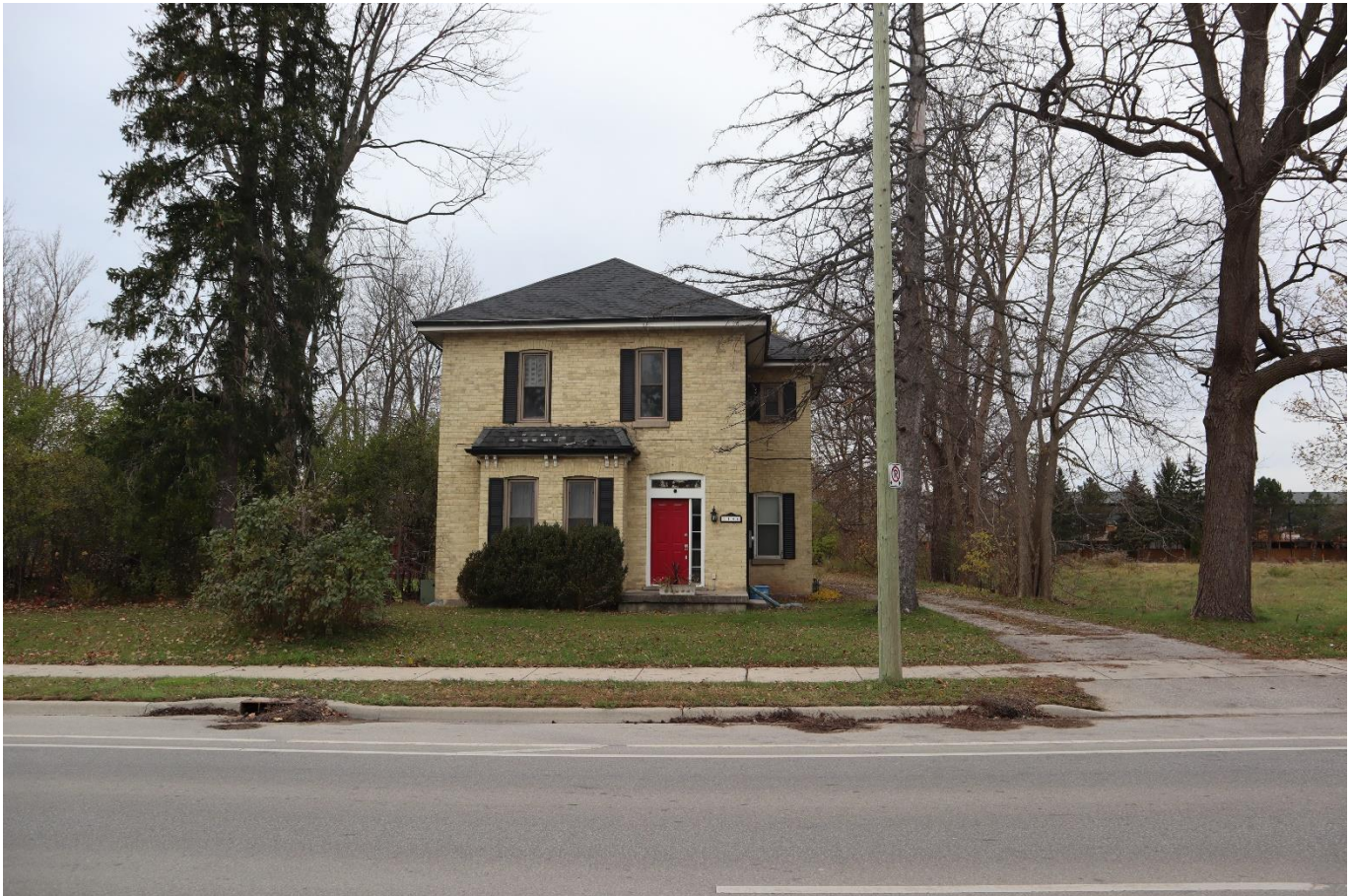
Photograph 11: View of southern elevation, looking north (AECOM 2021)
