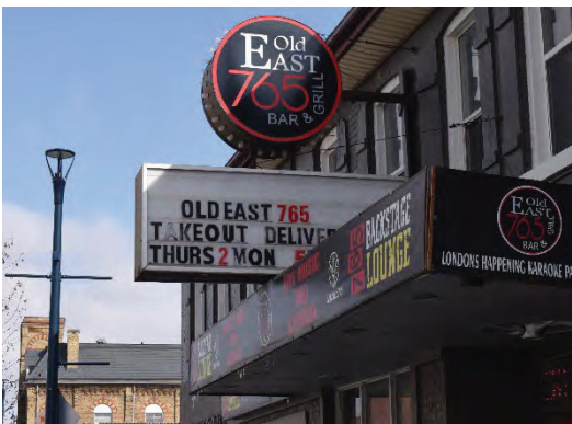
Plate 25: Overhang and signage, looking east
