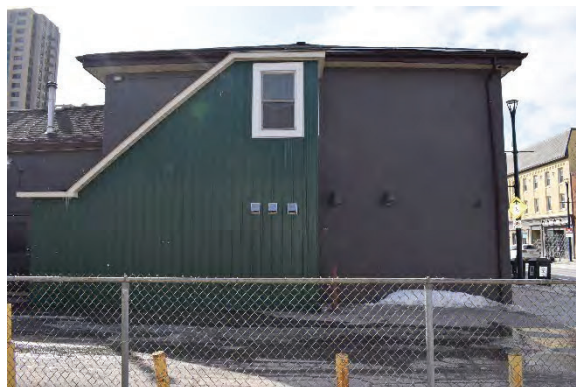
Plate 26: East façade of main section, looking west
