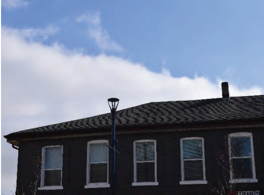
Plate 15: Hip roof section showing east chimney, looking south
