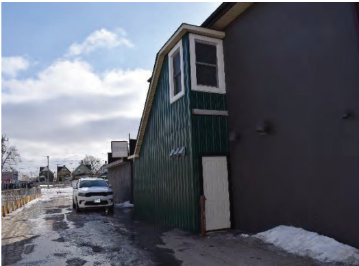
Plate 27: Enclosed staircase, looking south
