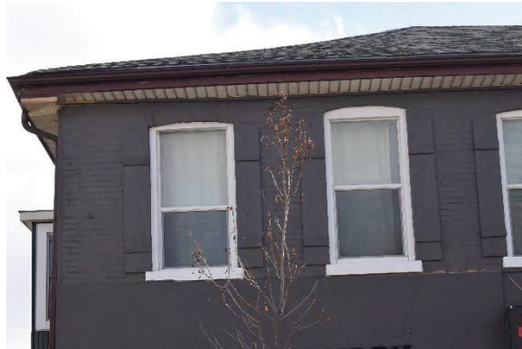
Plate 18: Size difference between eastern windows, looking south
