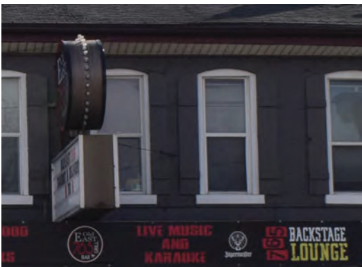
Plate 19: Narrower spacing and width of windows above main entrance, looking south
