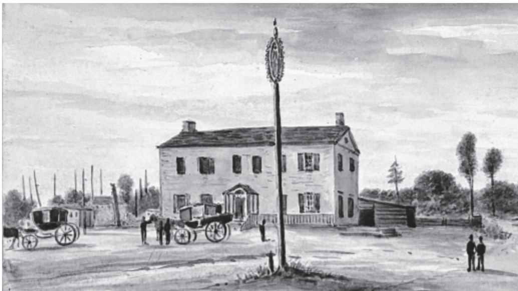
Plate 37: Georgian style hotel on the Bay of Quinte, circa 1830. Note the lack of ornamentation, massing, and strong horizontal line on the second storey fenestration similar to 763-769 Dundas Street (Roberts 2009:19)
