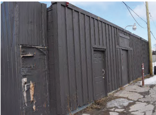
Plate 33: South façade of concrete block additions, looking east
