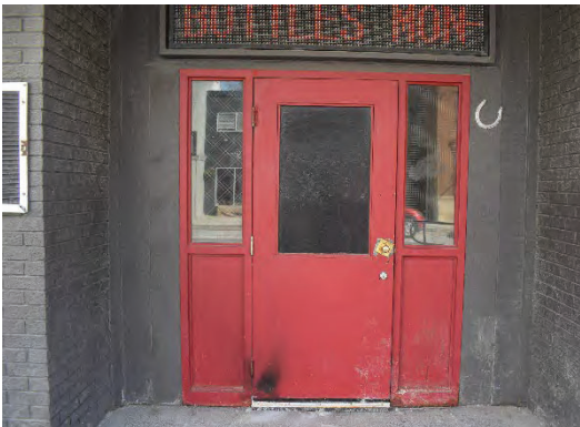
Plate 23: Main entrance, looking south
