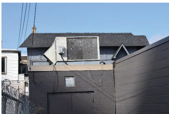
Plate 36: Gable and mansard parapet addition south façade, looking north
