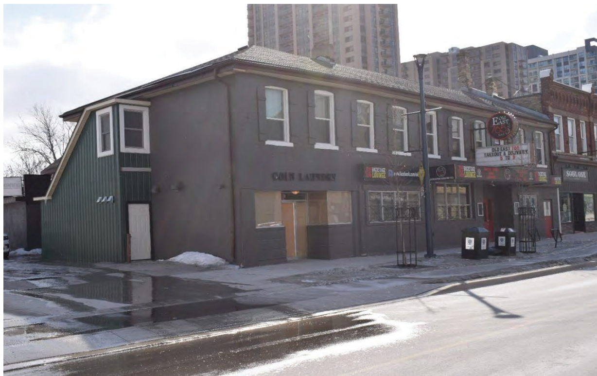
Plate 14: Looking southwest at 763-769 Dundas Street showing two storey structure and roof
