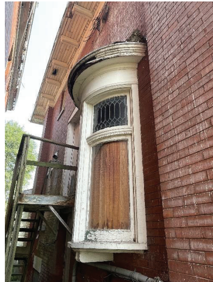
Photo 37: Curved window detail, west façade
