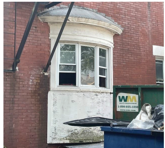
Photo 43: Curved bay window, north façade
