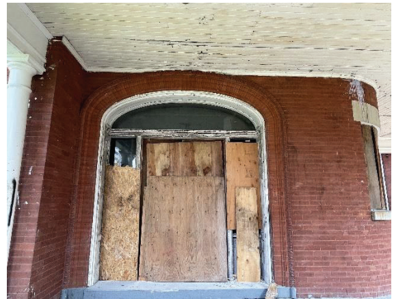
Photo 31: Front entrance door
