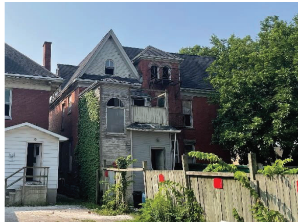
Photo 27: North façade, looking southwest
