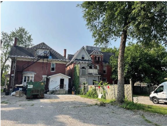
Photo 11: Parking spaces behind 300 and 306 Princess Avenue, looking southwest
