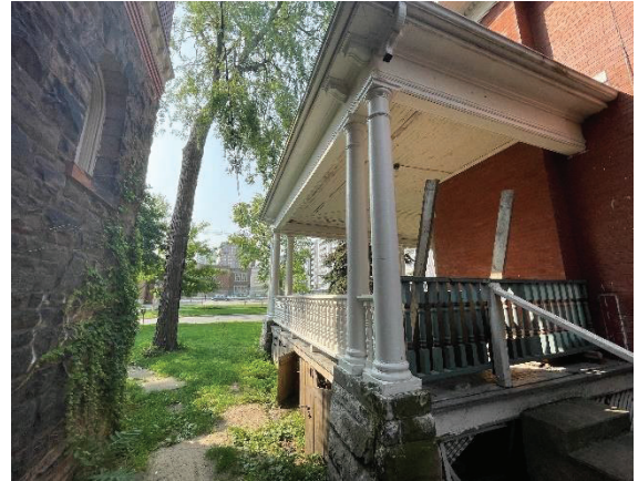
Photo 41: East façade wrap-around porch
