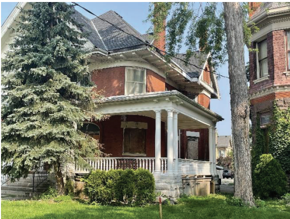
Photo 34: Rounded corner windows and porch
