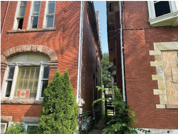
Photo 22: Eastern façade, looking north
