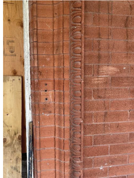
Photo 33: Brickwork surrounding front door
