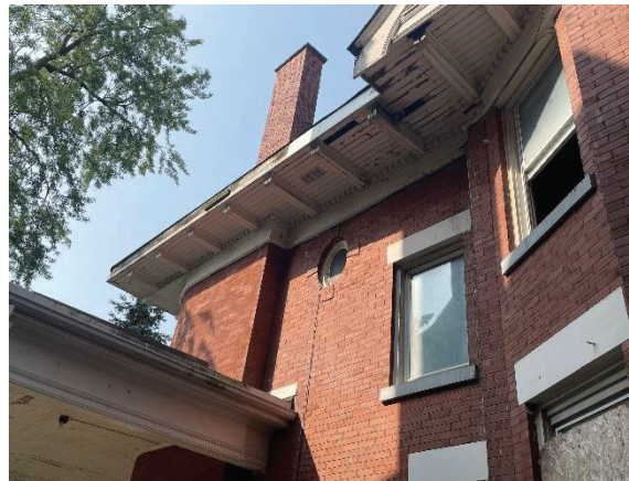
Photo 39: Oval and rectangular windows, east façade
