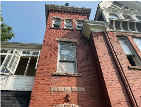
Photo 14: Middle bay of the residence on the front façade, including brick brackets, arched windows, stained-glass transom, and red stone detailing, looking north
