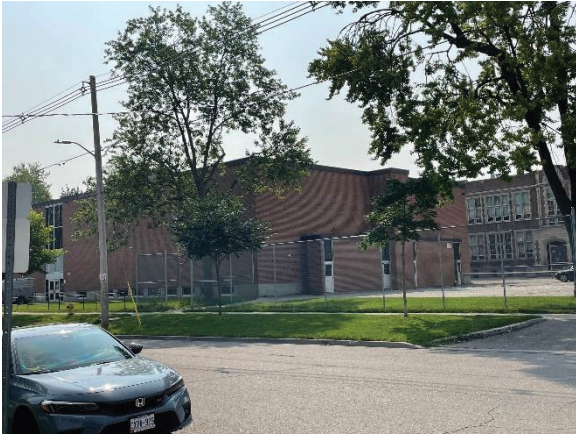
Photo 5: North façades of the London Central Secondary School, looking southeast
