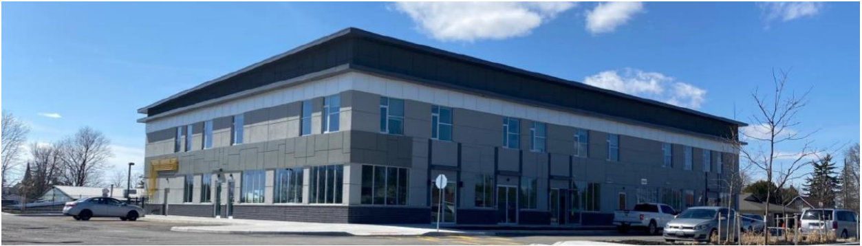
Figure 3: Office to the north
