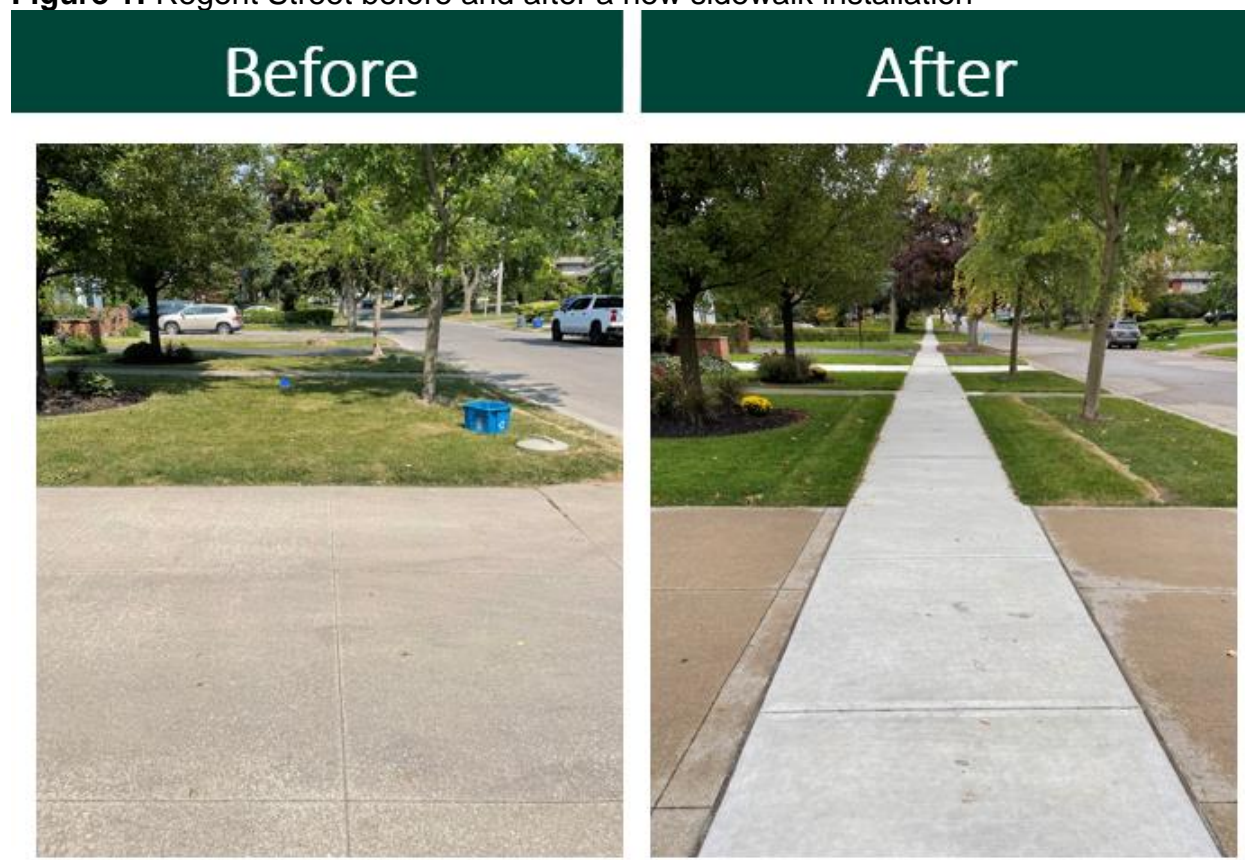
Figure 1: Regent Street before and after a new sidewalk installation
