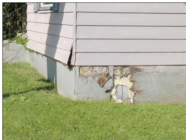
50. (left) approximately 60% of the building area is over a crawl space. This entire crawl space structure is improperly founded and has resulted in differential settlement.
