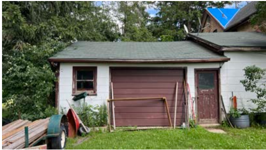
87. 7056 Pack Rd Garage Addition.HEIC
