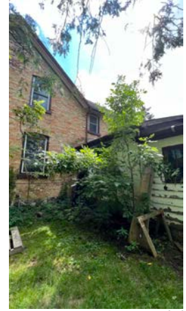
59. 7056 Pack Rd Rear Addition (Garage).HEIC
