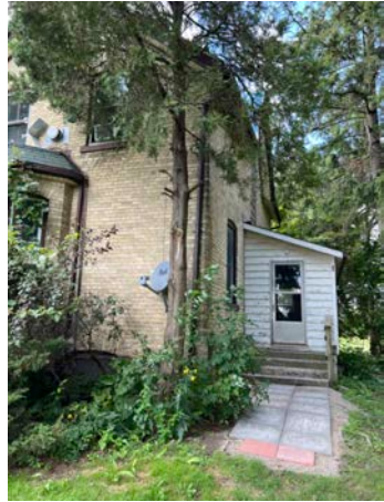
78. 7056 Pack Rd East Side Mud Room Addition.HEIC
