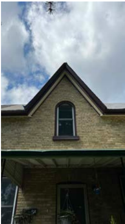
92. 7056 Pack Rd Peaked Dormer and Arched Window Opening.HEIC
