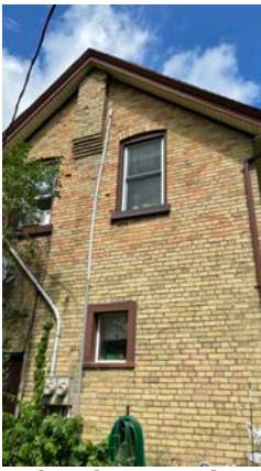
73. 7056 Pack Rd West Elevation Chimney Removal and Re-Bricking.HEIC
