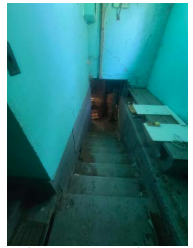
133 - Stairs to Basement.jpg
