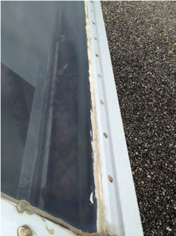
Library skylight exterior
