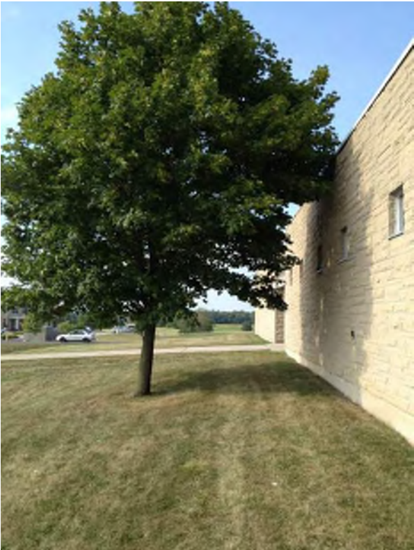
Trees at West elevation of 1988 addition - if not maintained properly will cause similar issues to those of the original building.
