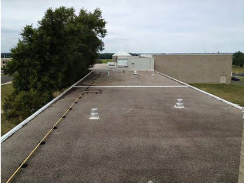
Overhanging trees at Roof H
