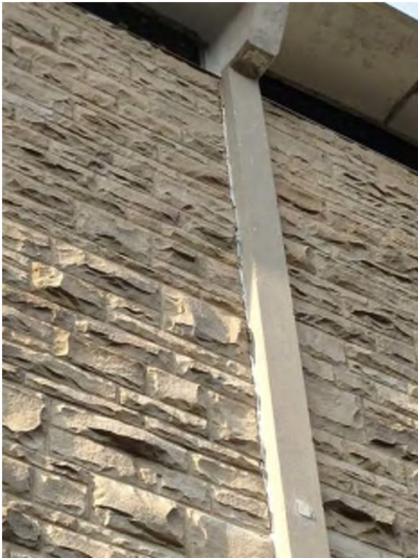
Caulked joint at Gymnasium wall - South Elevation
