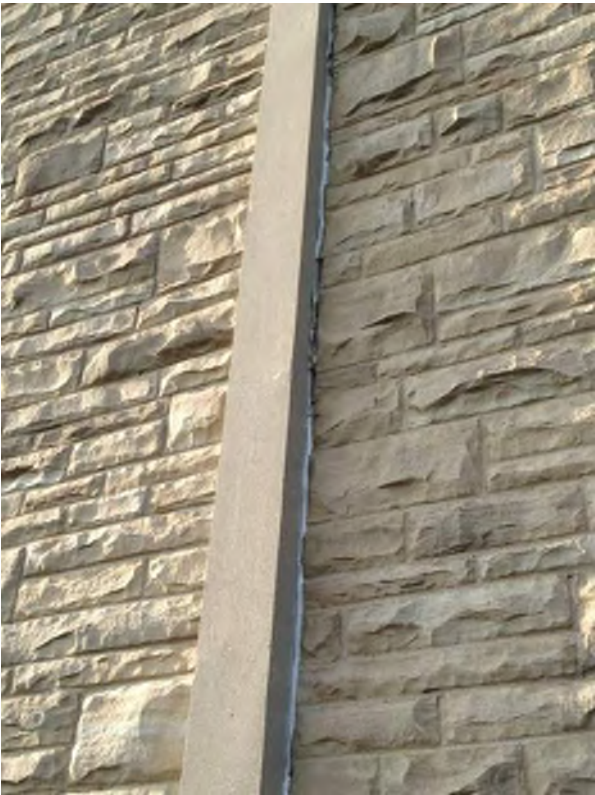
Caulked joint at Gymnasium wall - South Elevation
