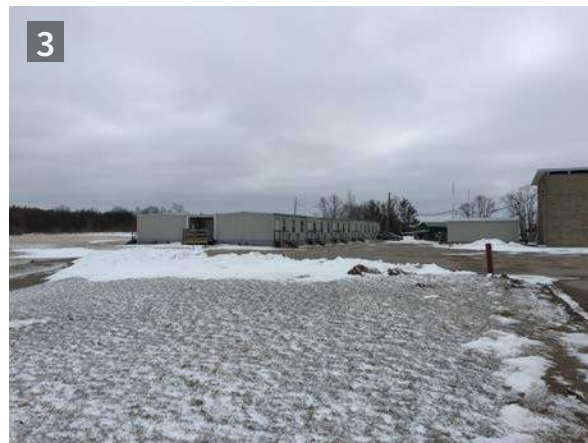
Looking south towards portable classrooms (ERA, 2018).
