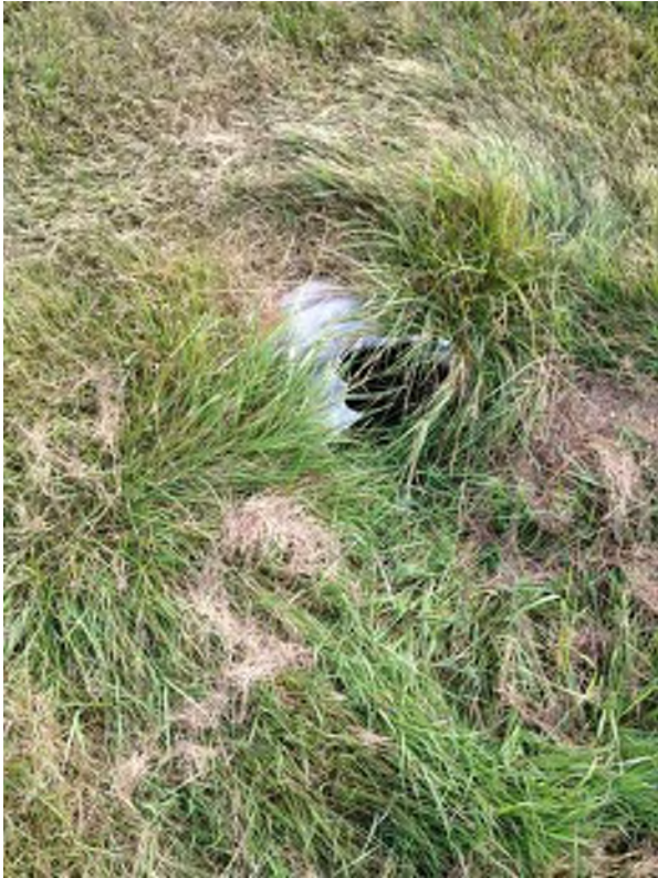
Drain culvert in grass
