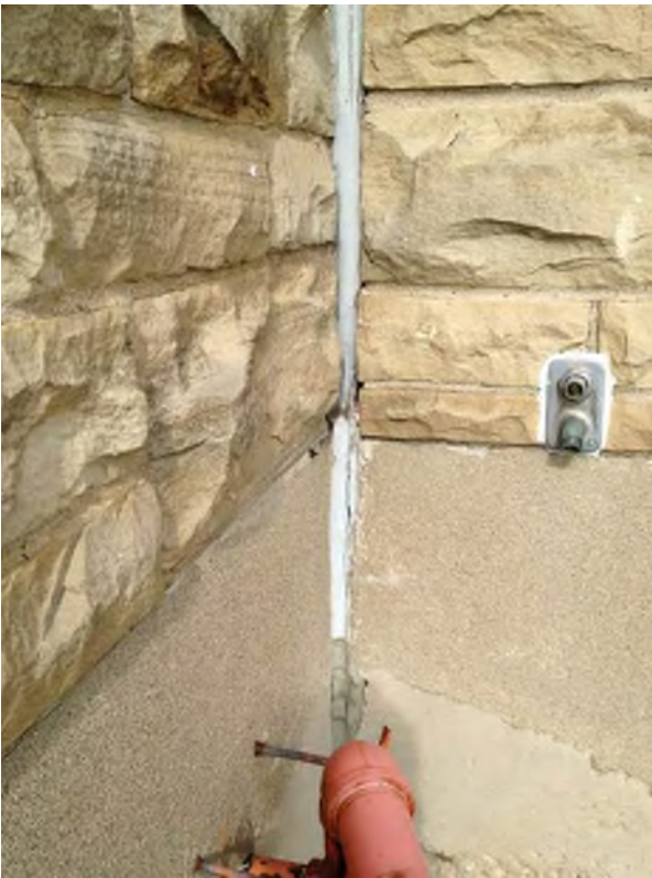
Caulked corner west elevation
