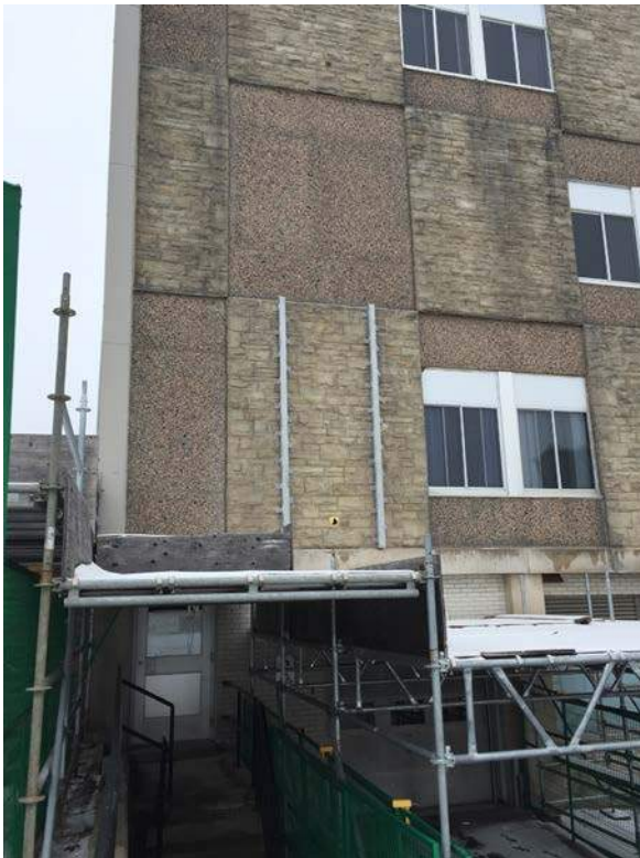
Steel bracing for loose panel, east elevation. Scaffolding installed over maintenance door and garage (ERA, 2018).
