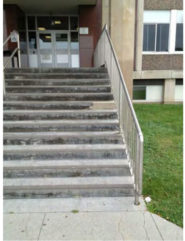
Front entry exterior stairs
