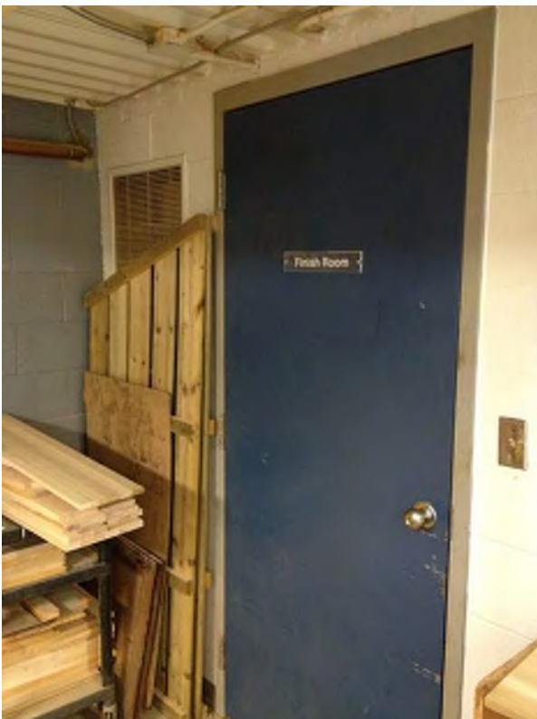
Construction Technology Classroom Finishing Room - entry doors and transfer grill,
