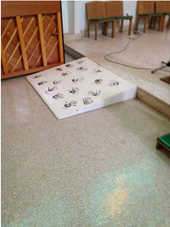
Wood ramp at chapel sanctuary
