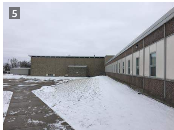
Looking south towards "gymnasium" wing (ERA, 2018).
