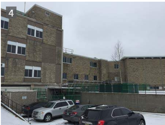
Looking north towards rear elevation of school and "gymnasium" wing (ERA, 2018).
