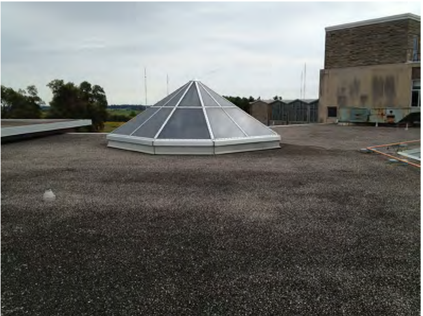
Overall image of library skylight exterior
