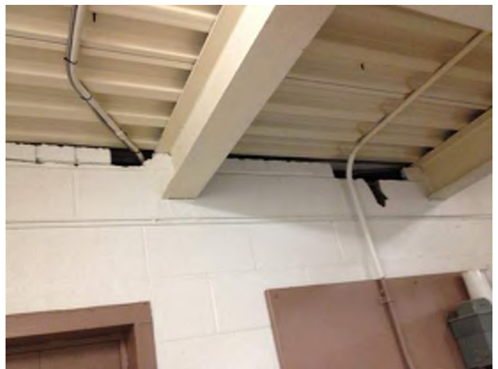
Fire separation at elevator machine room
