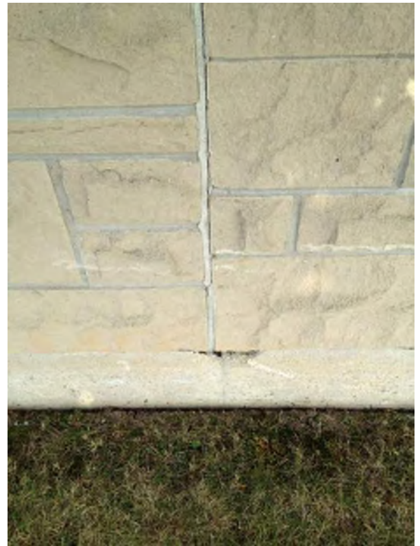
Caulked expansion joint at 1988 addition
