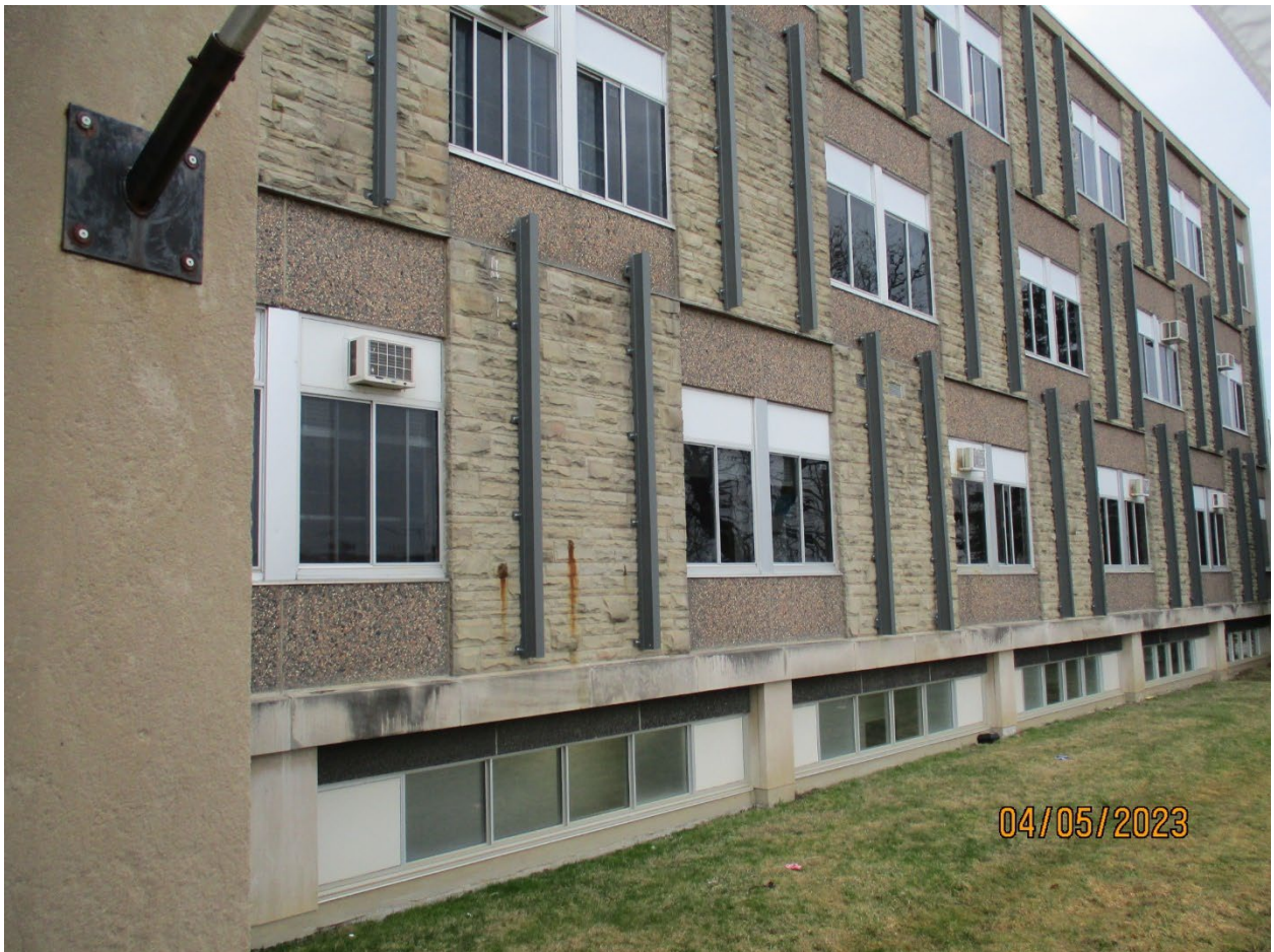
Image 8: Exterior cladding of the Regina Mundi Catholic College showing "checkboard" pattern of precast masonry panels and "random stone" panels.
