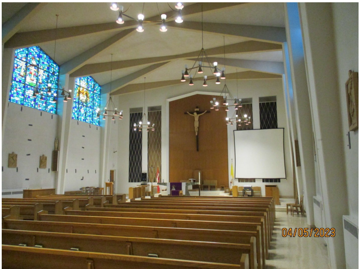
Image 10: Interior of the chapel in the Regina Mundi Catholic College. Note, the tapered columns around the perimeter of the chapel and the folded plate roof structure.
