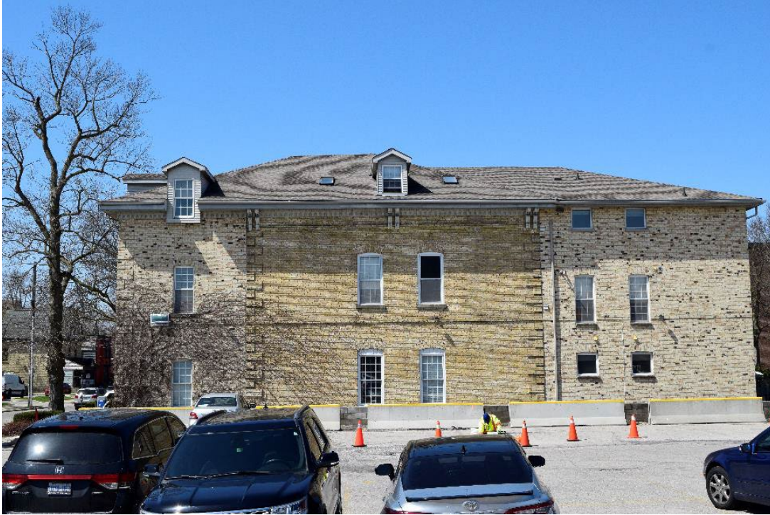
Figure 22: East wall of 186 Albert Street as seen from 200 Albert Street
