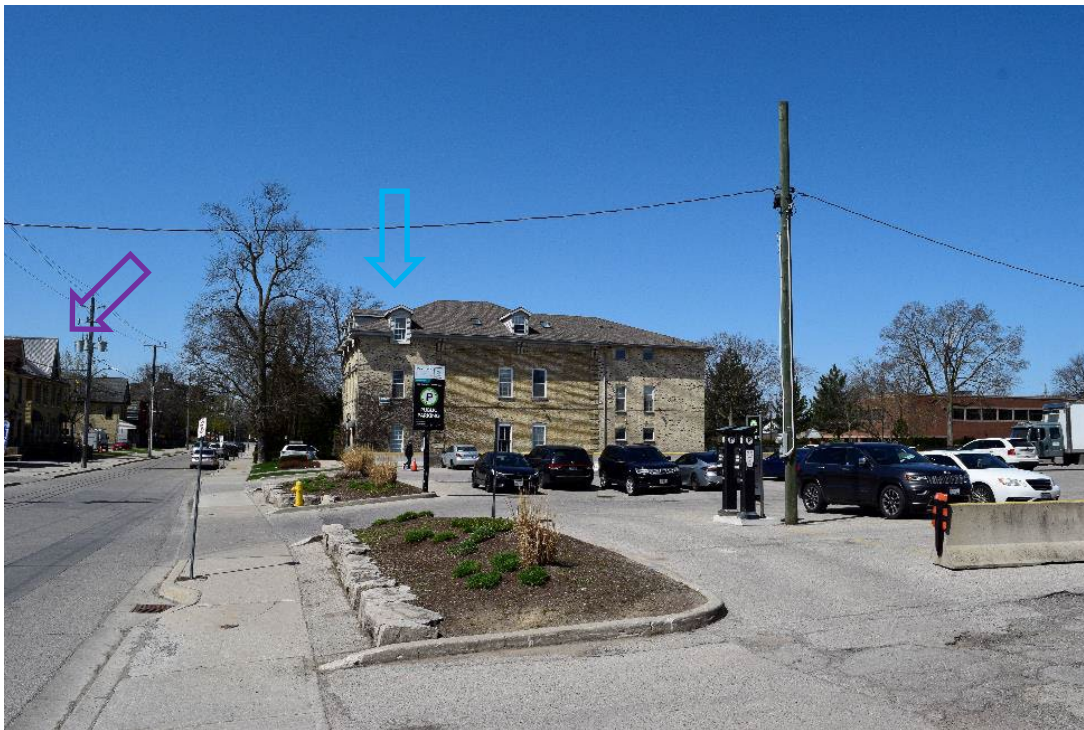
Figure 16: Looking west into 200 Albert Street from southeast corner of property, 186 Albert Street (blue arrow), 179 and 181 Albert Street are on left of image (purple arrow)
