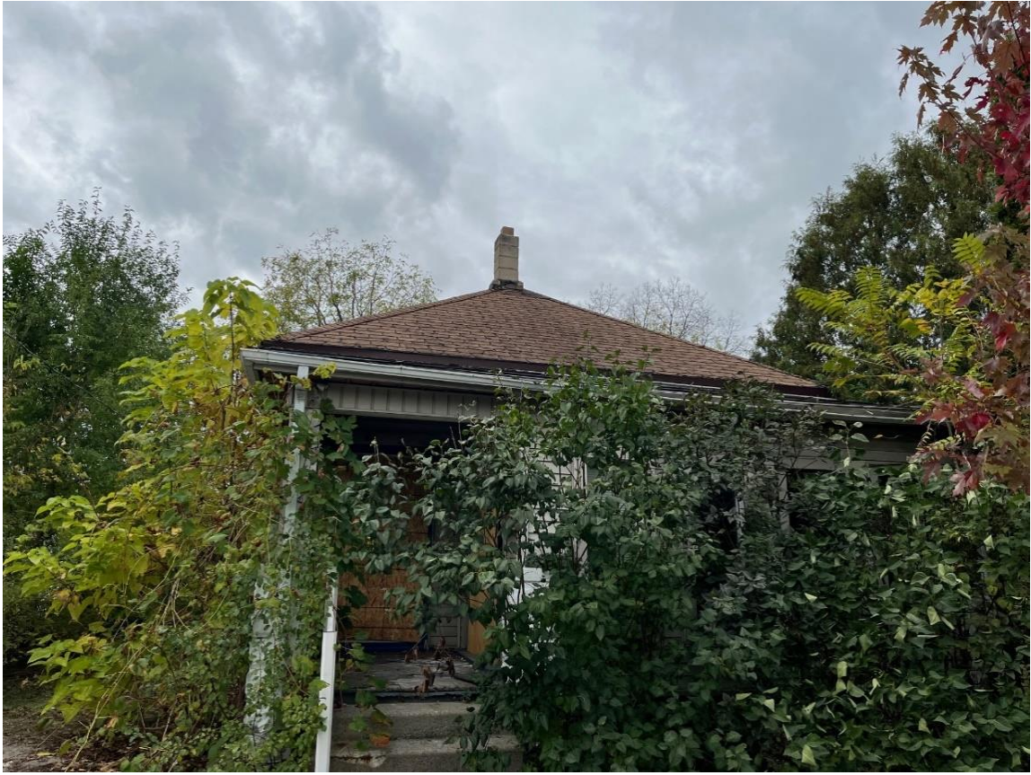
19 Redan Street – Front Exterior
