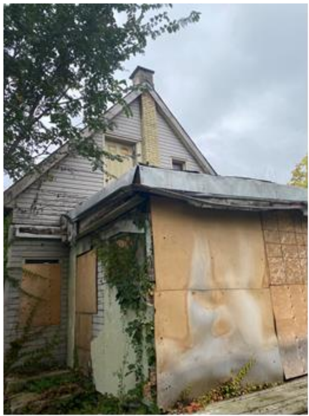
188 Wharncliffe Rd S – Rear Photos
