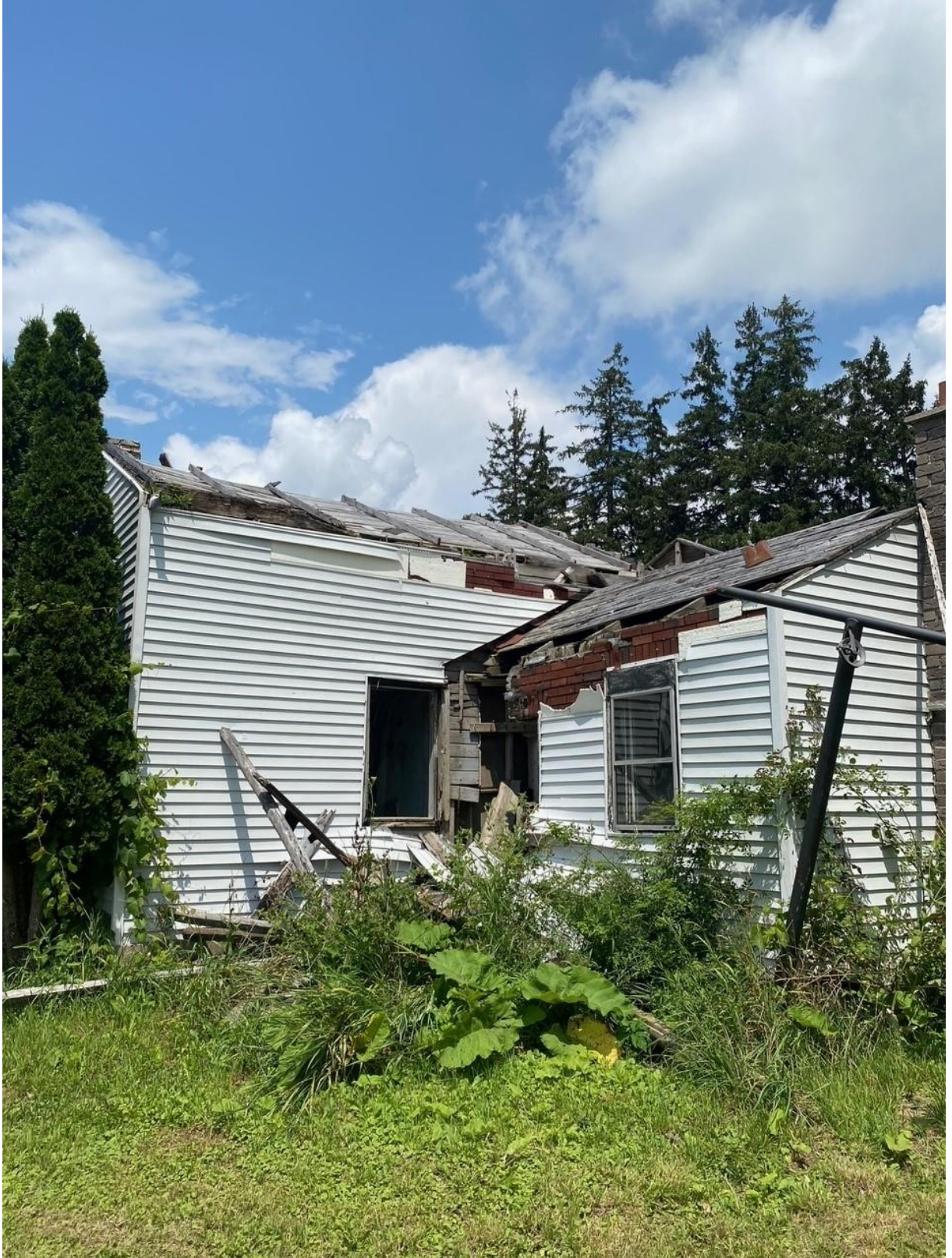
1803 Bradley Ave – Rear Exterior
