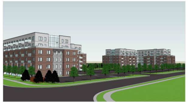
2 VIEW OF BLOCK 6 FROM NW
