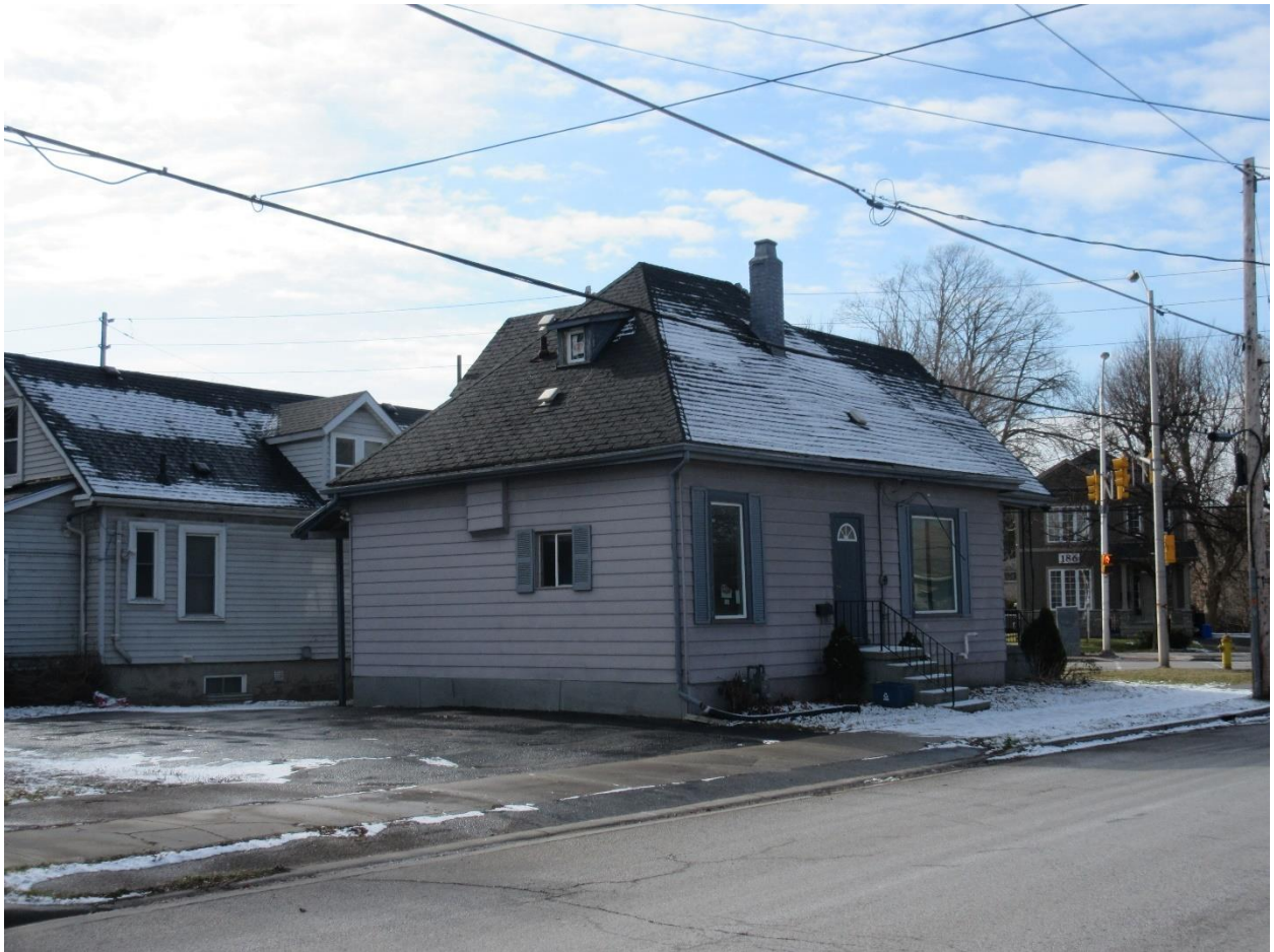
Image 3: Northeast corner of the Contributing Resource at 187 Wharncliffe Road North (taken February 5, 2016).
