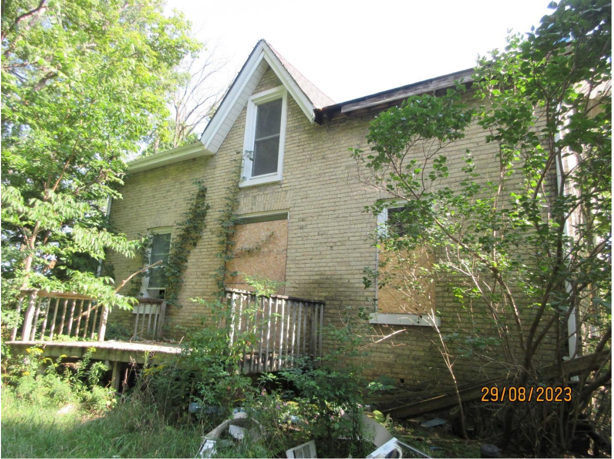
Image 6: Photograph showing north elevation of farmhouse (L.Dent, August 29, 2023).
