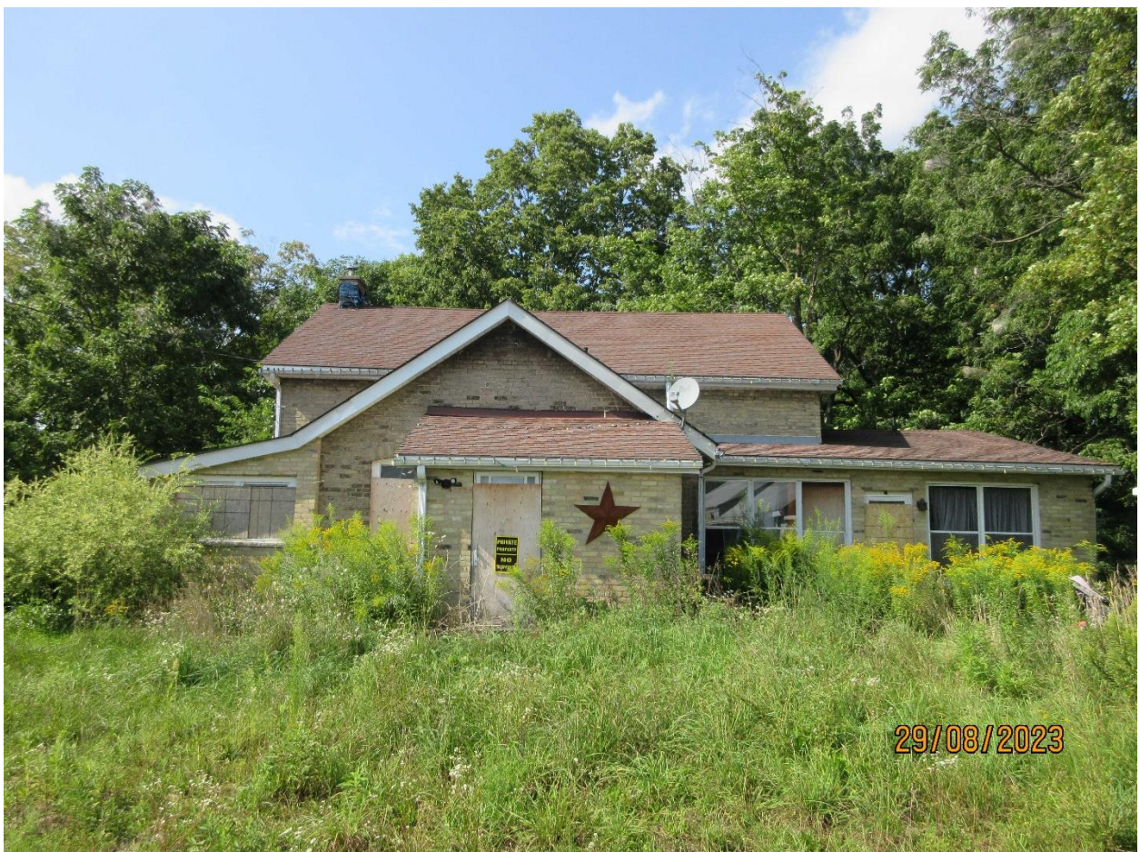
Image 4: Photograph of south elevation of farmhouse showing multiple additions (L.Dent, August 29, 2023).
