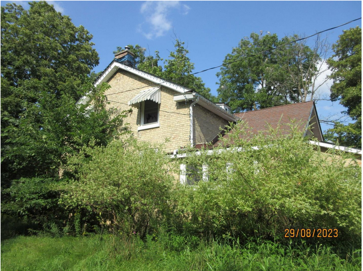
Image 5: Photograph showing west elevation of farmhouse (L.Dent, August 29, 2023).
