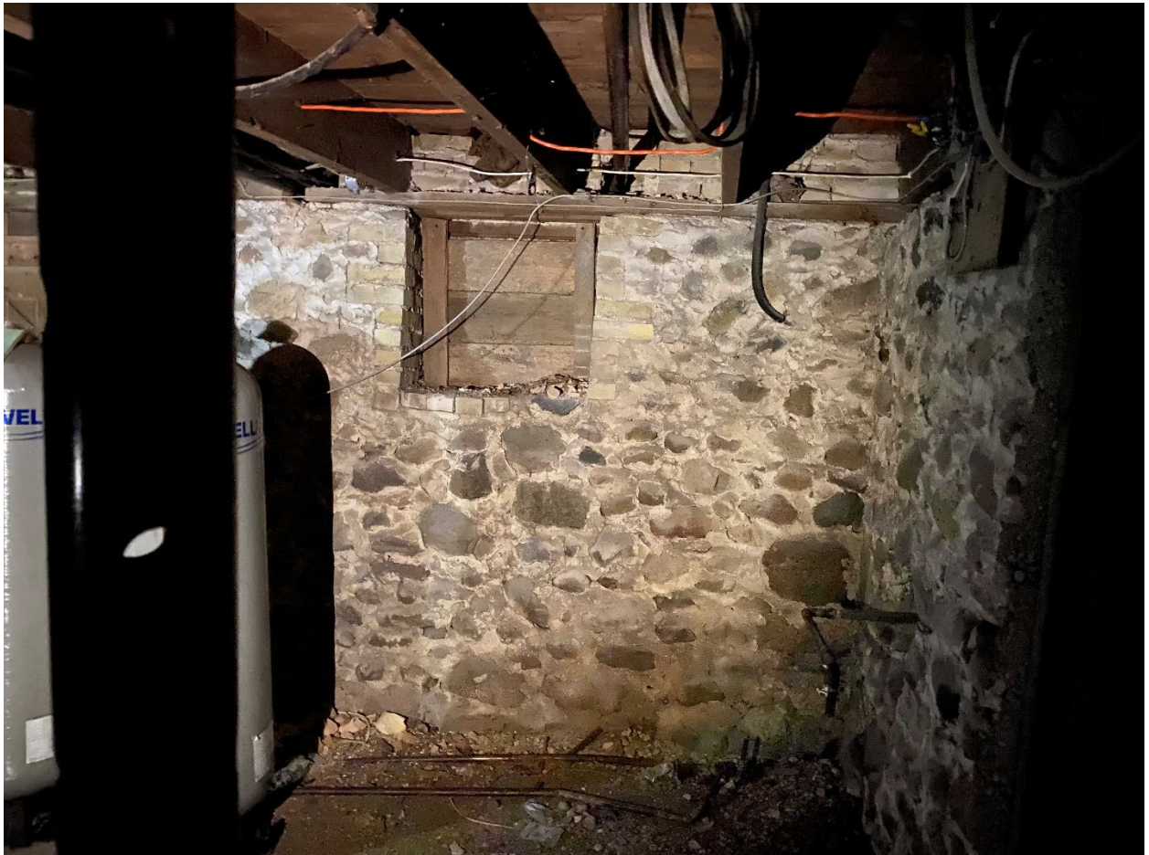
Image 15: Photograph of basement and stone foundation wall (L.Dent, March 14, 2022)
