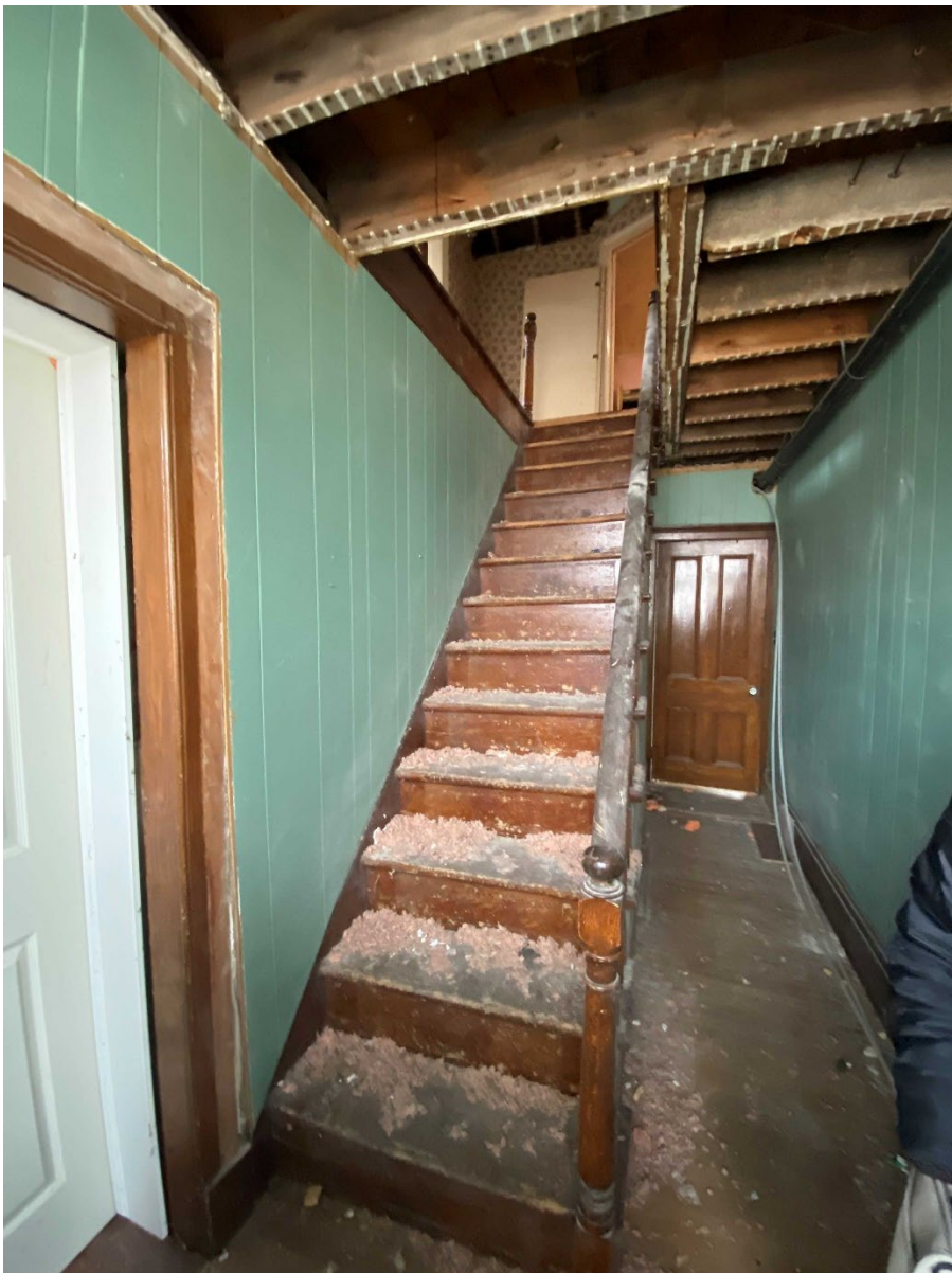
Image 11: Photograph showing interior centre hall and stairway (L.Dent, March 14, 2022).
