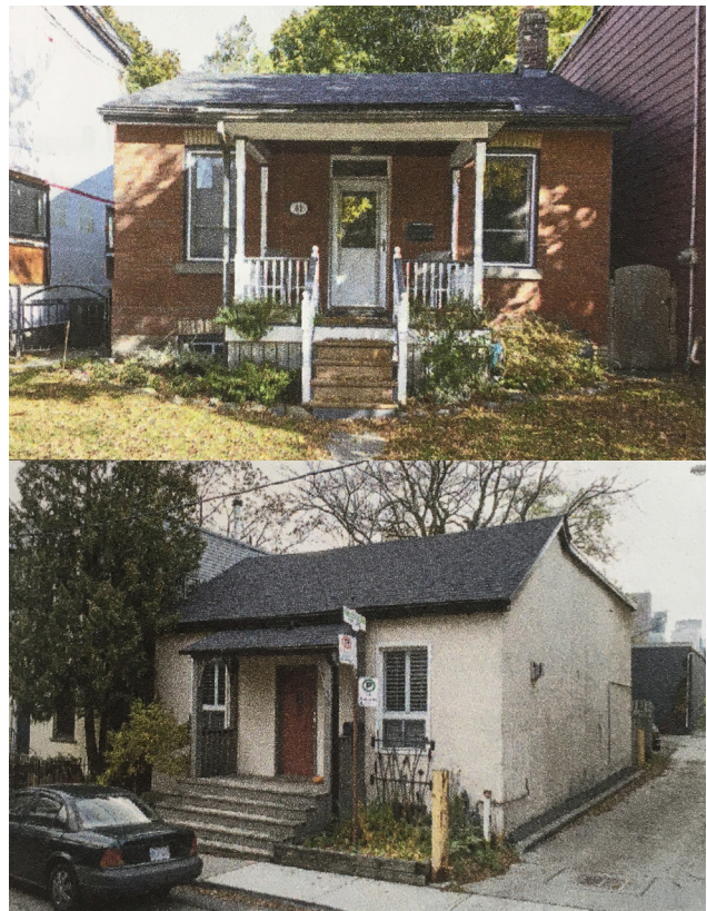
Figure 45: Examples of one-storey workers' cottages in Toronto. Hipped roofs are more common on London examples (Modest Hopes, pp. 30 & 33).
