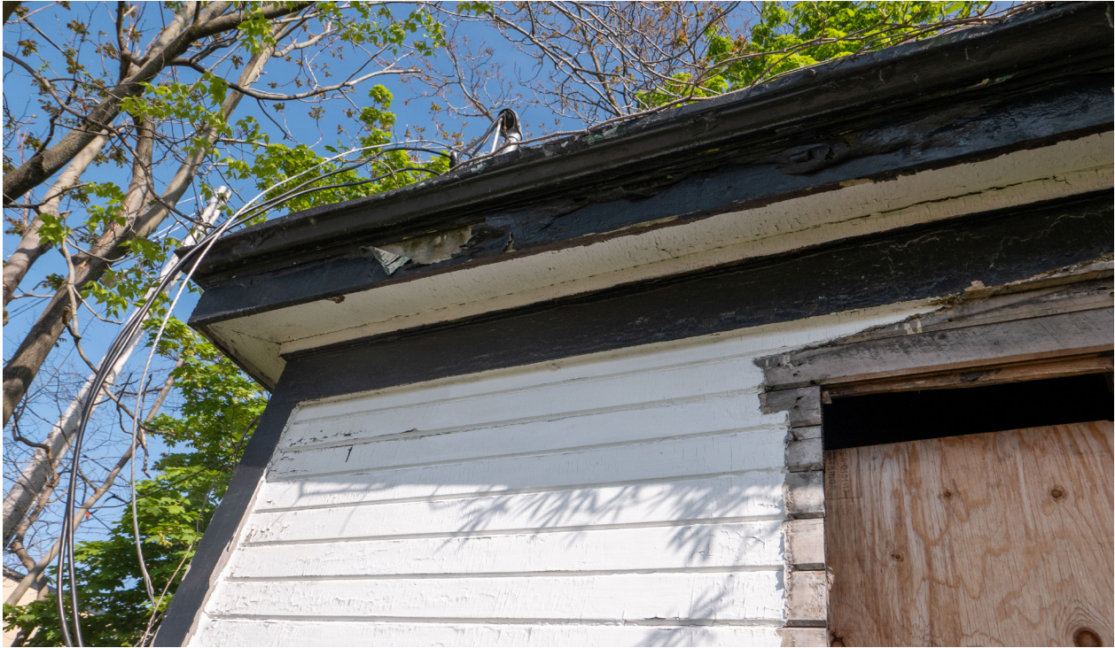
Figure 15: Upper west corner of the south elevation, showing wood siding, corner and cornice board detailing (CBCollective, 2023).
