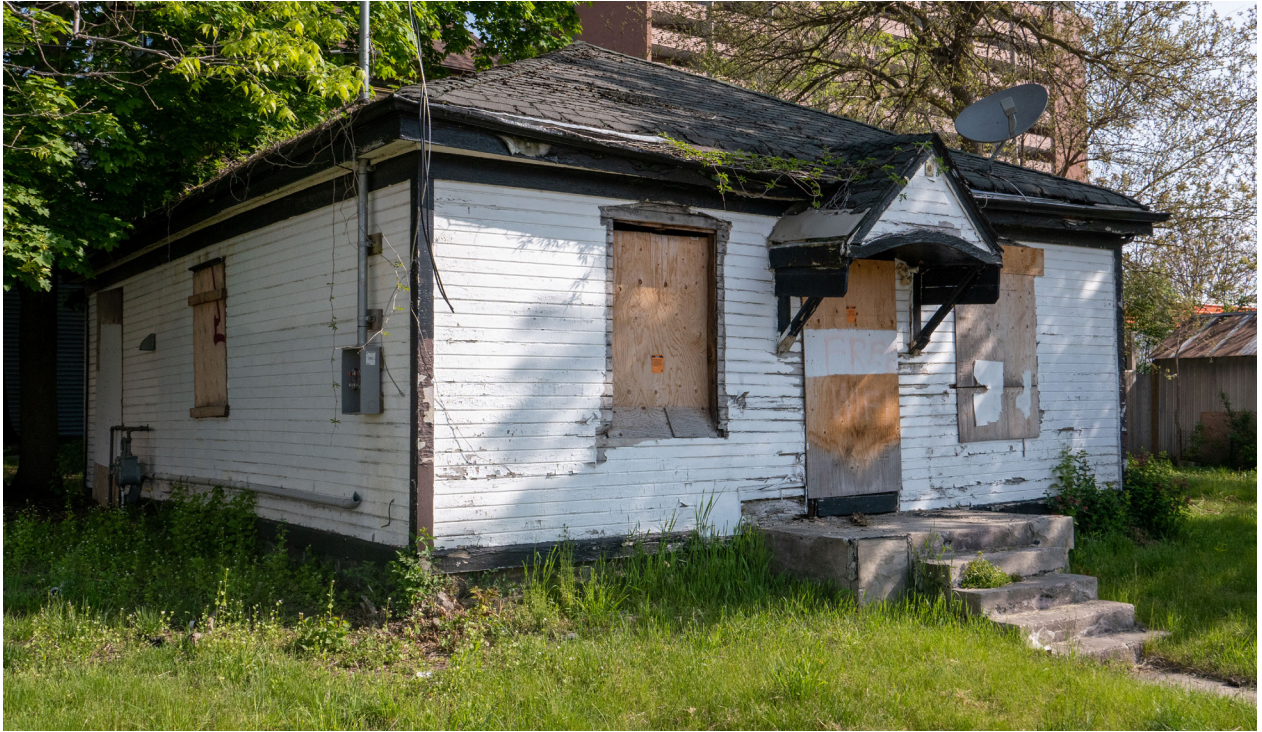
Figure 9: View of the dwelling's south and west elevations (CBCollective, 2023).
