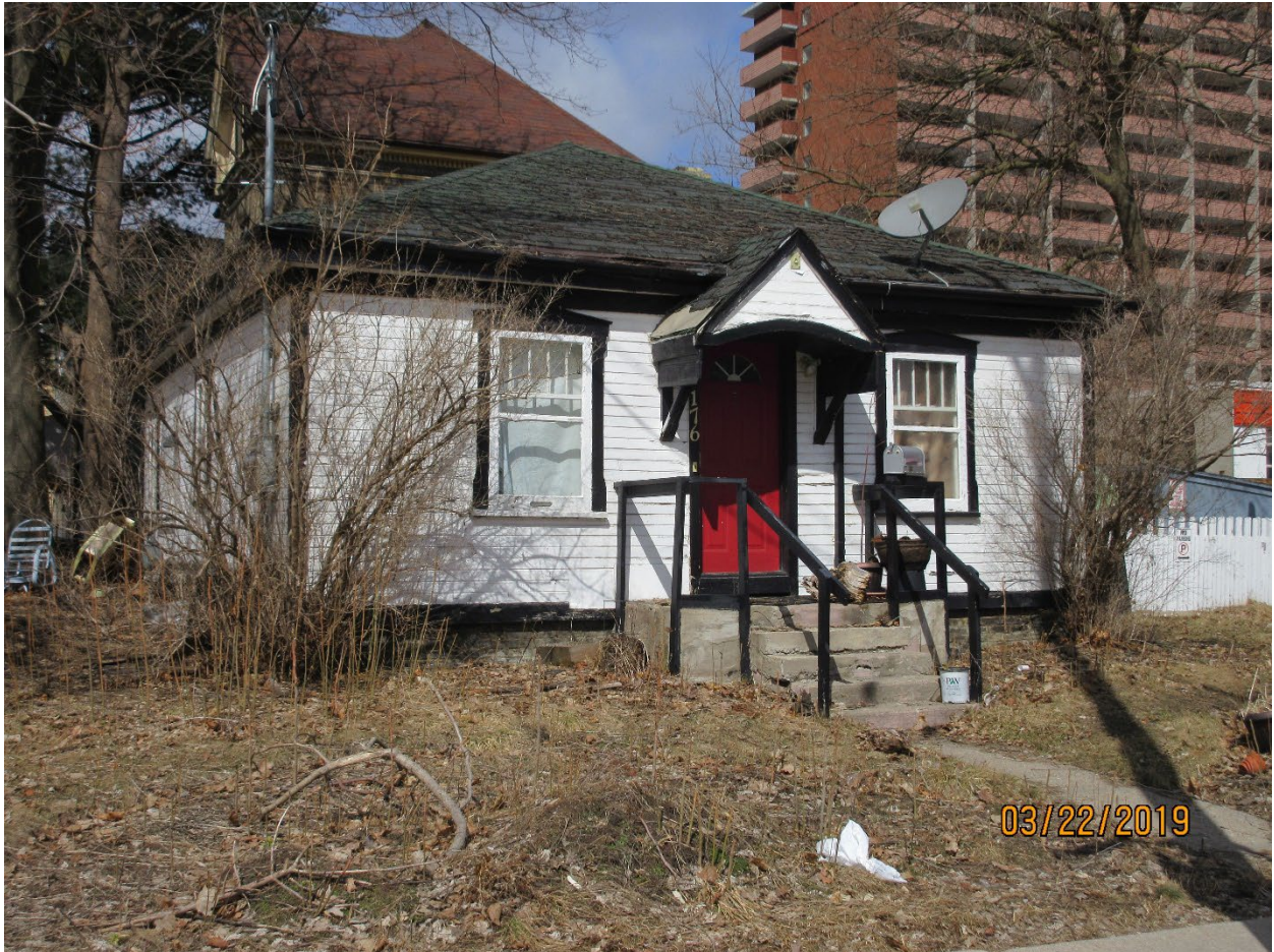
Image 9: South elevation of the building on the subject property at 176 Piccadilly Street, March 22, 2019.
