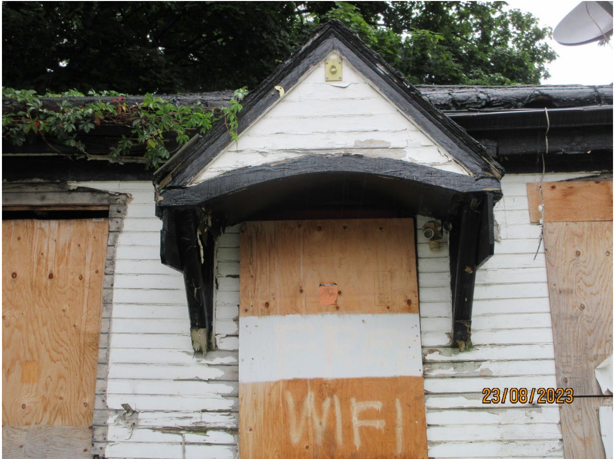
Image 5: Awning on the south elevation of the building on the subject property at 176 Piccadilly Street, August 23, 2023.
