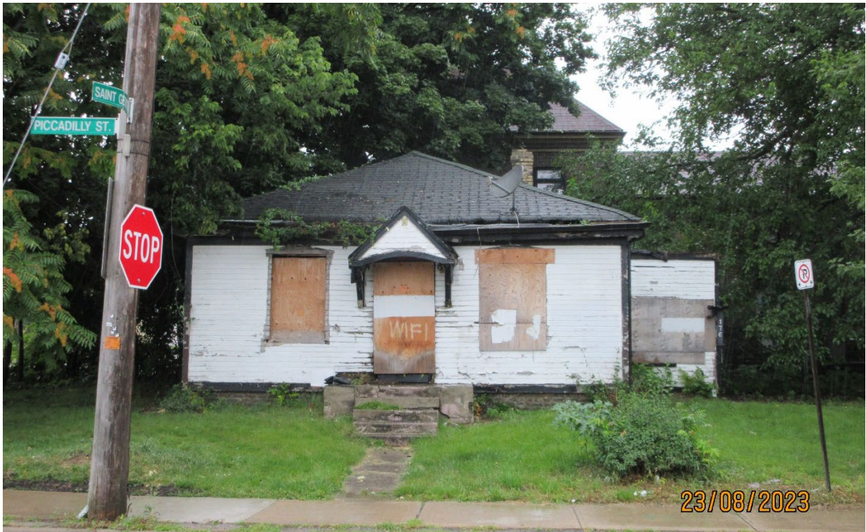
Image 1: South elevation of the building on the subject property at 176 Piccadilly Street, May 2, 2022.
