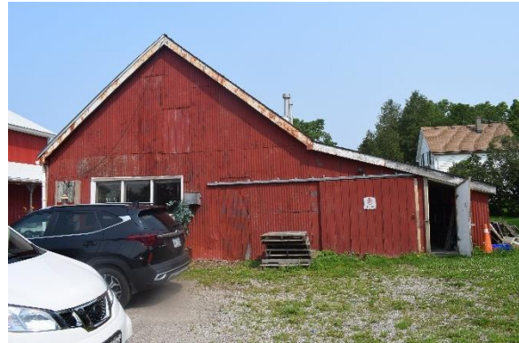
Plate 55: South elevation, looking north
