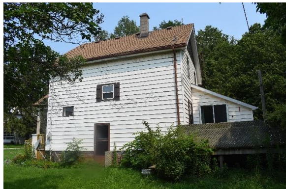
Plate 43: South elevation, looking north
