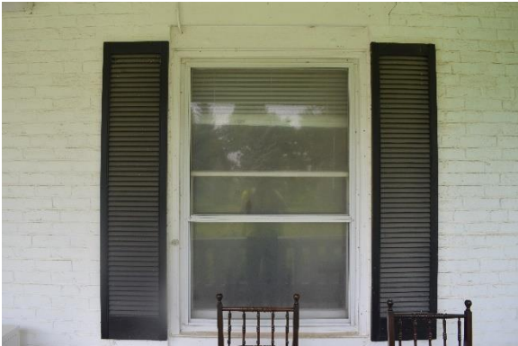
Plate 24: First storey window west of main entrance, looking south
