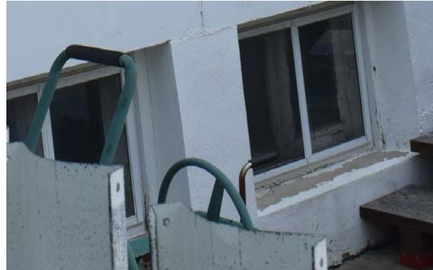
Plate 19: Concrete foundation, looking east
