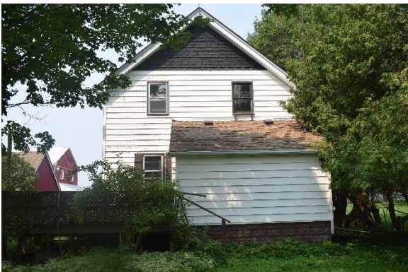
Plate 42: East elevation, looking west
