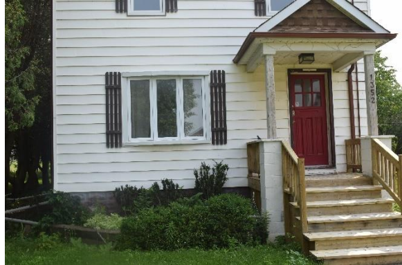
Plate 39: First storey of west elevation, looking east
