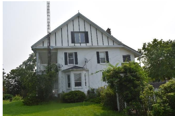
Plate 27: West elevation, looking east
