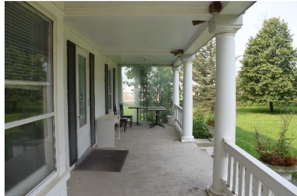
Plate 25: View of porch, looking west
