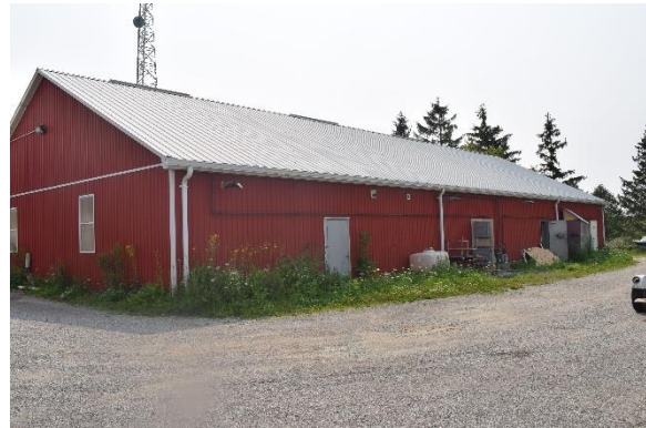
Plate 57: Outbuilding, west and north elevations, looking south
