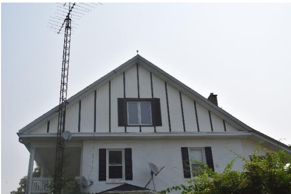
Plate 28: Second storey details, looking east
