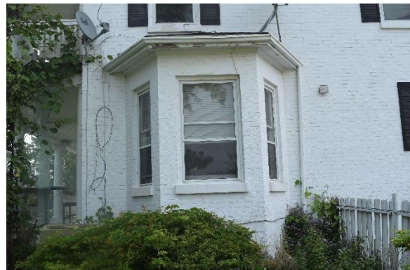
Plate 29: Bay window, looking east
