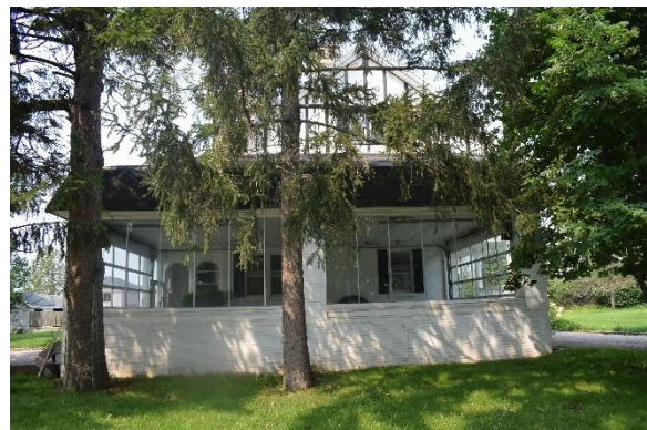
Plate 35: East elevation, looking west
