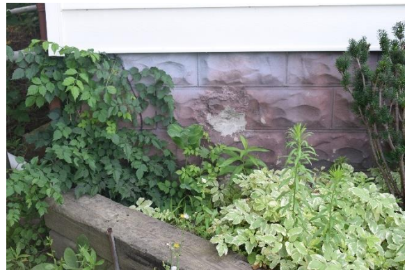
Plate 37: Foundation, looking east
