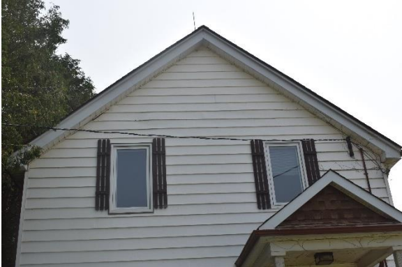
Plate 38: Second storey of west elevation, looking east
