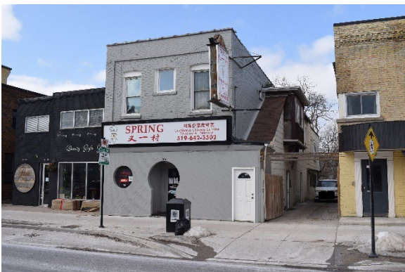
Plate 8: Example of modified structures, looking north
