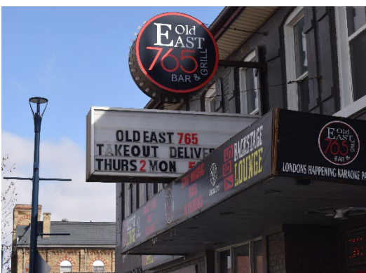
Plate 25: Overhang and signage, looking east
