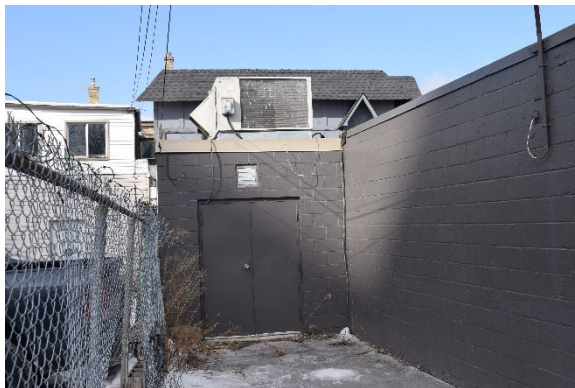
Plate 34: South façade showing doors and concrete block exterior
