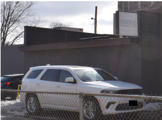
Plate 29: East façade of flat roof addition with parapets, looking west
