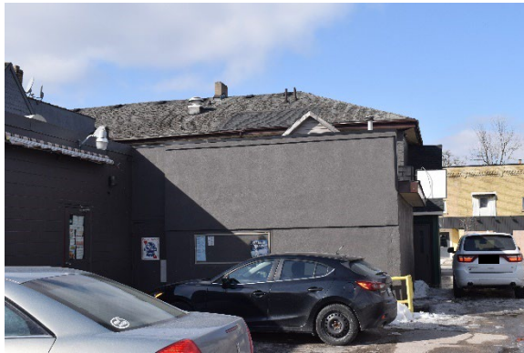
Plate 32: Looking north showing south façade of flat roof with parapet addition
