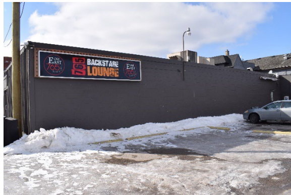
Plate 30: East façade of concrete block addition, looking west
