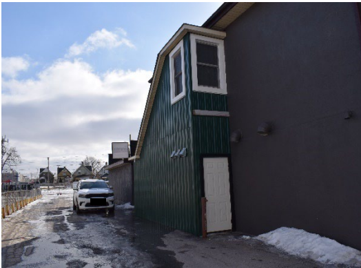
Plate 27: Enclosed staircase, looking south
