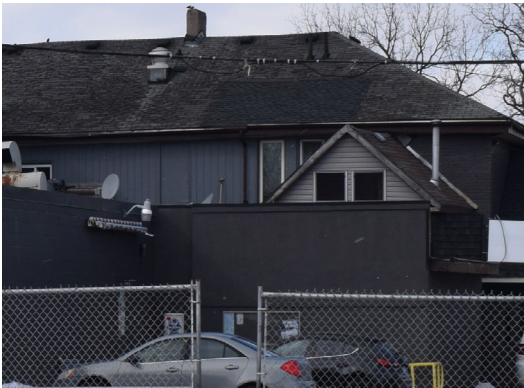
Plate 31: Looking north showing south façade of main section and gable addition
