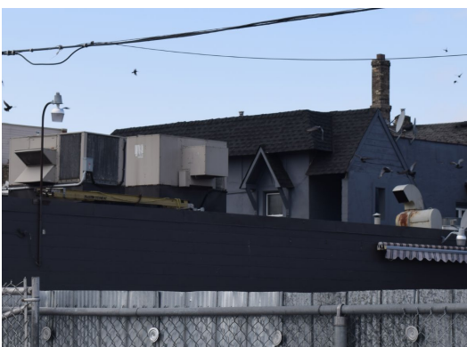
Plate 35: Looking southwest at gable and mansard parapet addition
