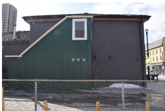
Plate 26: East façade of main section, looking west
