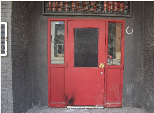
Plate 23: Main entrance, looking south
