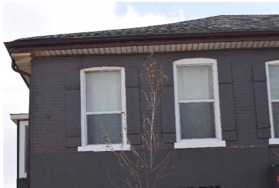
Plate 18: Size difference between eastern windows, looking south
