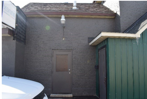
Plate 28: East façade of gable roof addition, looking west
