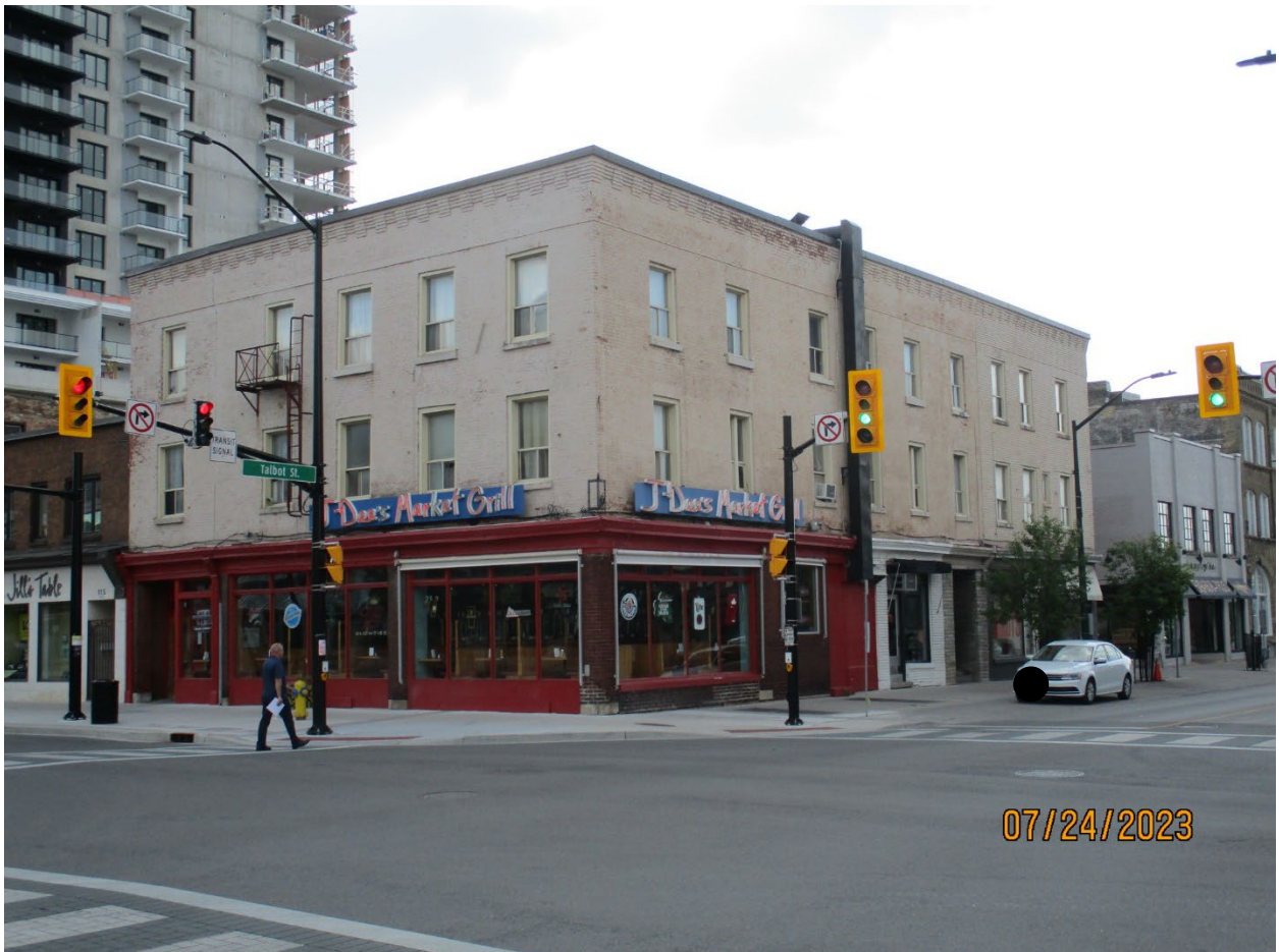
Image 8: Photograph showing the heritage designated property at 360-366 Talbot Street (Bank Hotel, c. 1870), located within the Downtown Heritage Conservation District.
