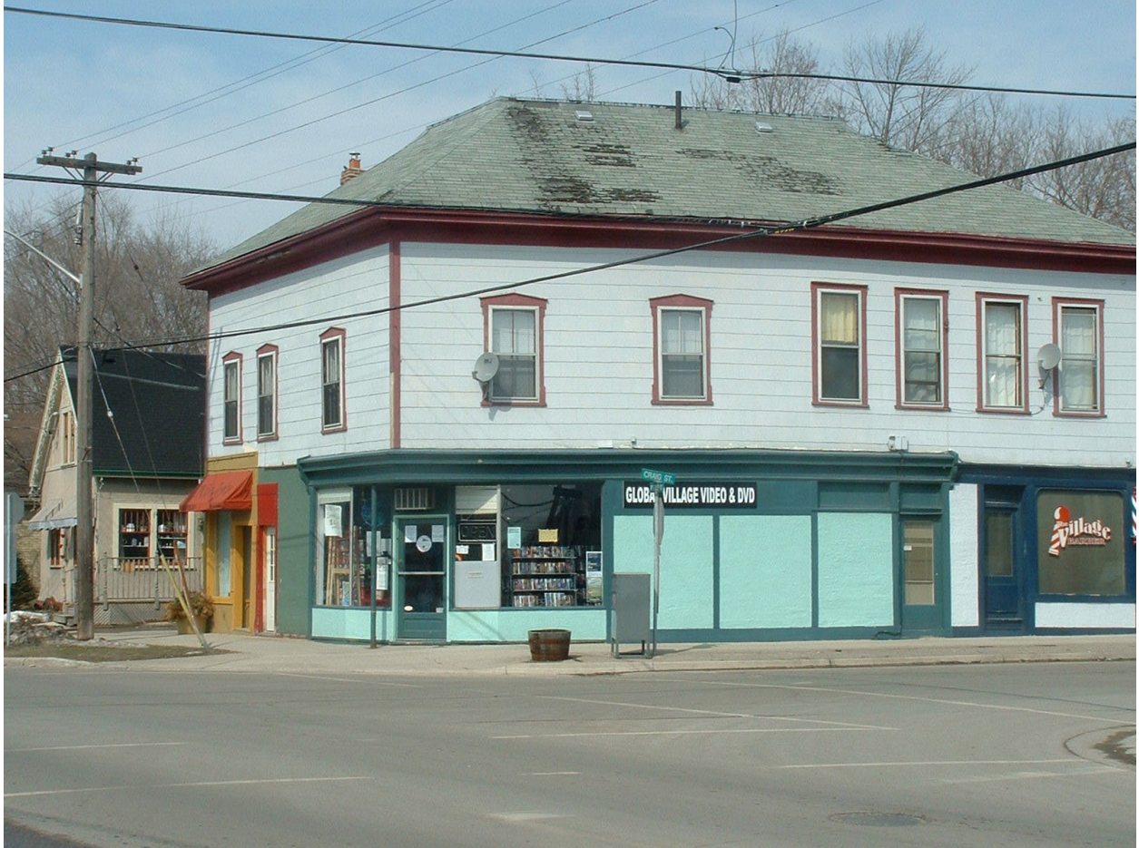
Image 1: Photograph taken on March 17, 2002, showing the former building at 134 Wortley Road.
