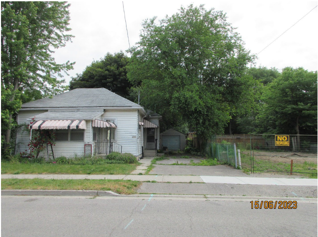
Image 4: Photograph of the dwelling at 526 Ontario Street, located north of the subject property, June 15, 2023.
