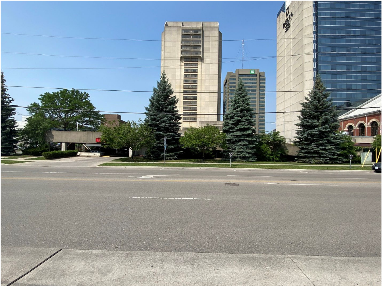
Image 3: View of existing parking garage showing green buffer and plantings – facing west (L.E. Dent, June 28, 2023).
