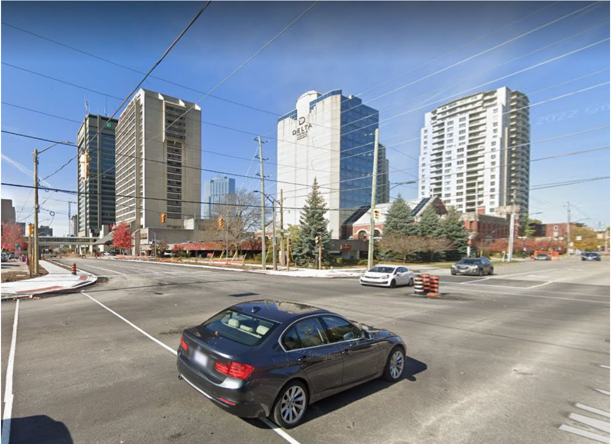
Image 6: View of King Street and Waterloo Street intersection with the existing parking structure at the corner and high-rise buildings including the Hilton DoubleTree Hotel, Delta Armouries Hotel, and City Place apartment – facing northwest (Google Street View, October 2022 - extracted July 22, 2023).
