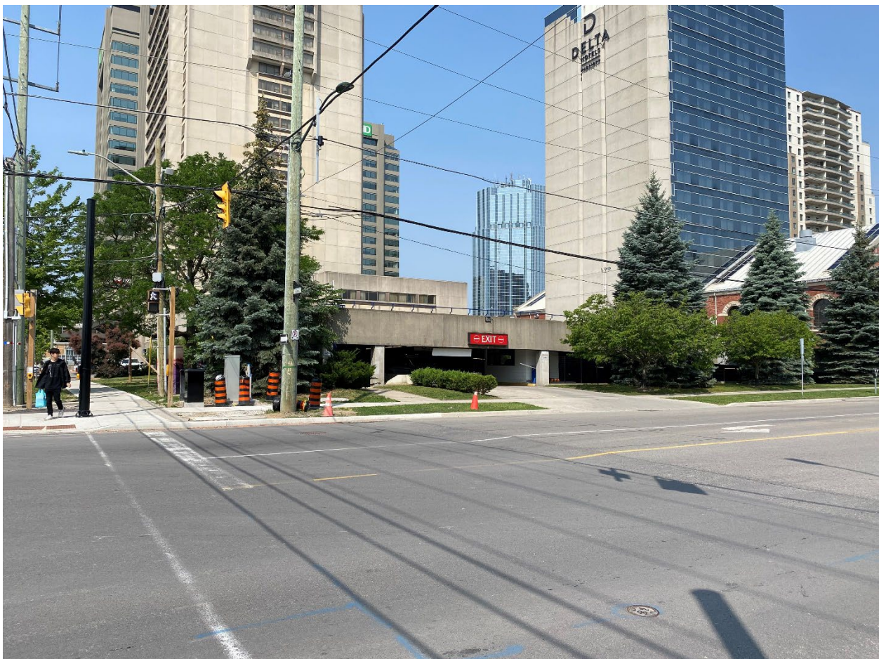
Image 2: View of existing parking garage exit ramp onto Waterloo Street – facing west (L.E. Dent, June 28, 2023).
