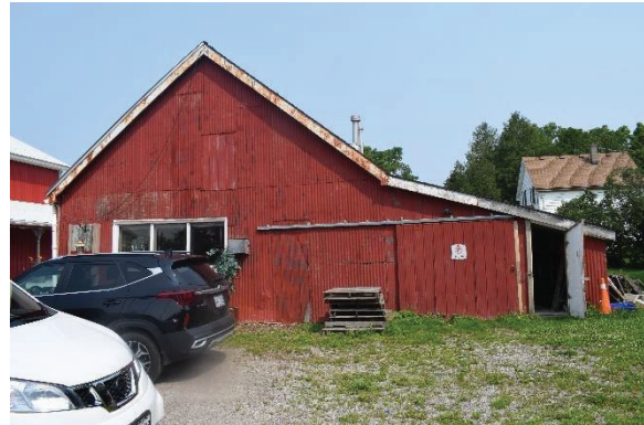
Plate 55: South elevation, looking north
