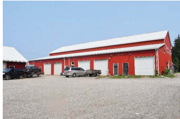
Plate 51: South elevation, looking north
