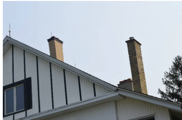
Plate 17: Chimney details, looking east
