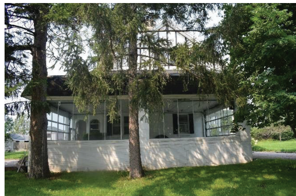
Plate 35: East elevation, looking west
