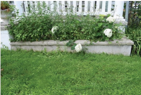
Plate 26: Concrete planter attached to porch, looking south
