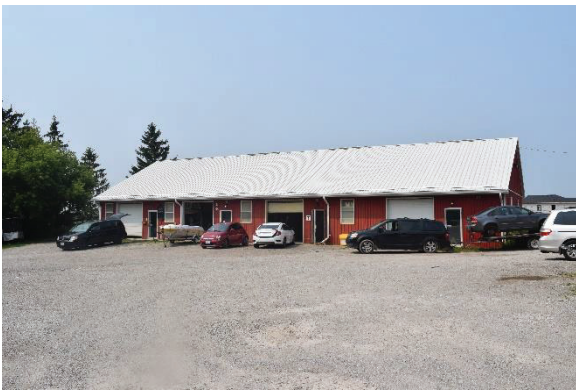
Plate 56: Outbuilding main elevation, looking west
