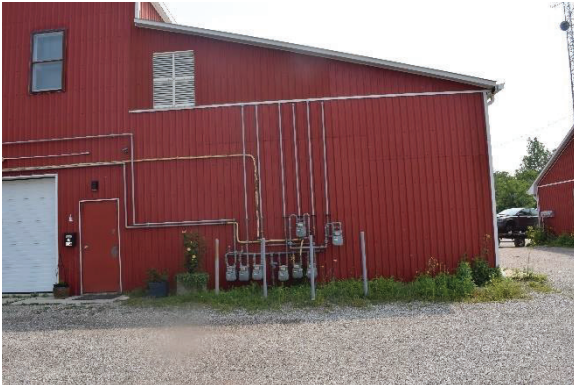
Plate 50: Shed roof section, looking east
