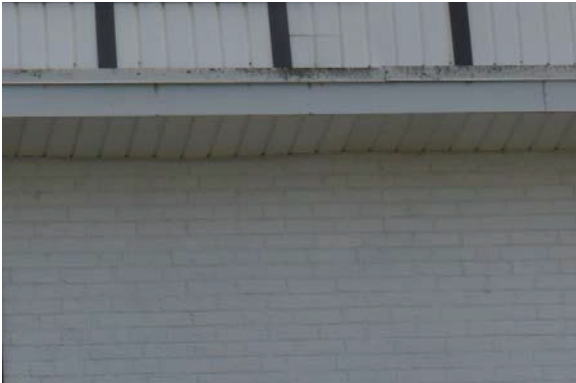
Plate 18: Painted brick exterior (bottom) and modern siding (top), looking east
