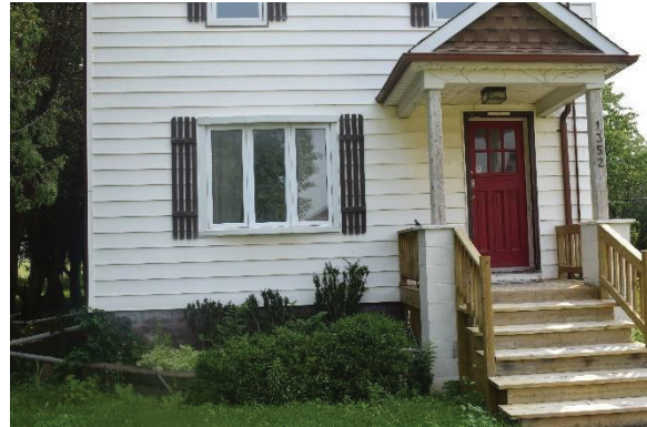
Plate 39: First storey of west elevation, looking east
