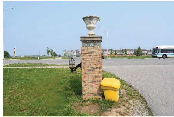
Plate 7: Details of west gate post, looking northwest
