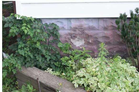
Plate 37: Foundation, looking east
