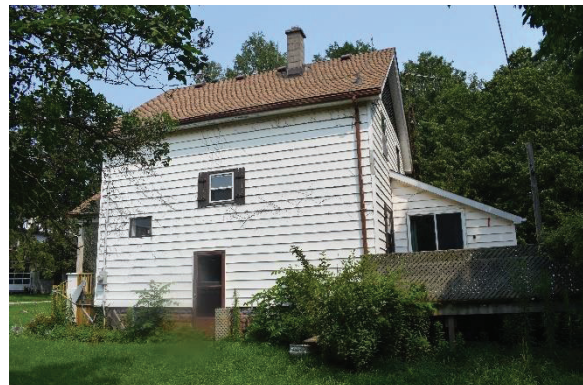
Plate 43: South elevation, looking north
