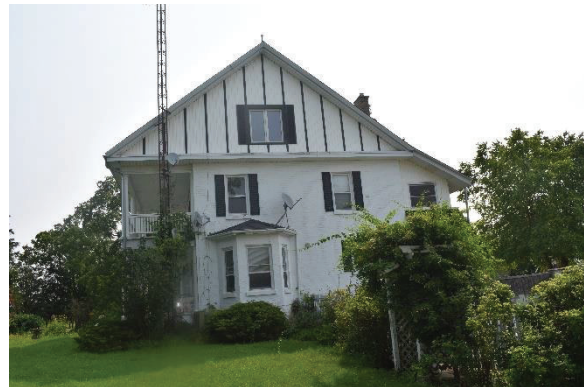
Plate 27: West elevation, looking east
