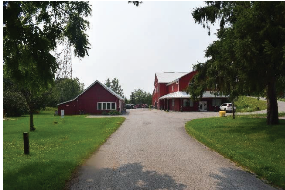
Plate 11: Looking south towards circulation routes
