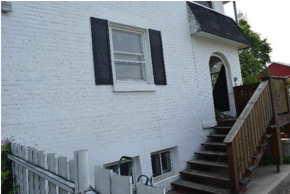
Plate 30: Looking southwest at doorway to pool area
