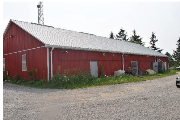
Plate 57: Outbuilding, west and north elevations, looking south
