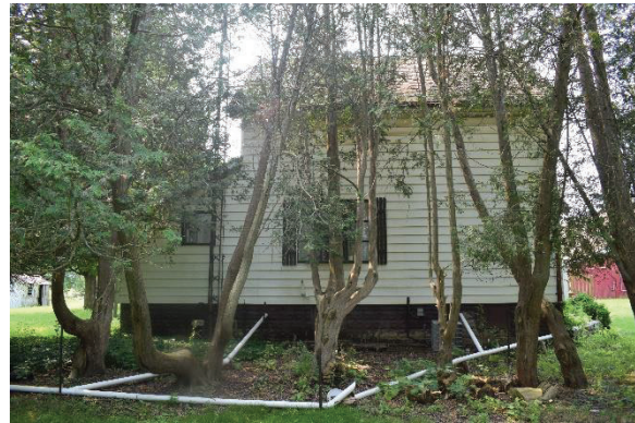
Plate 41: North elevation, looking south showing window in shed roof projection (left)
