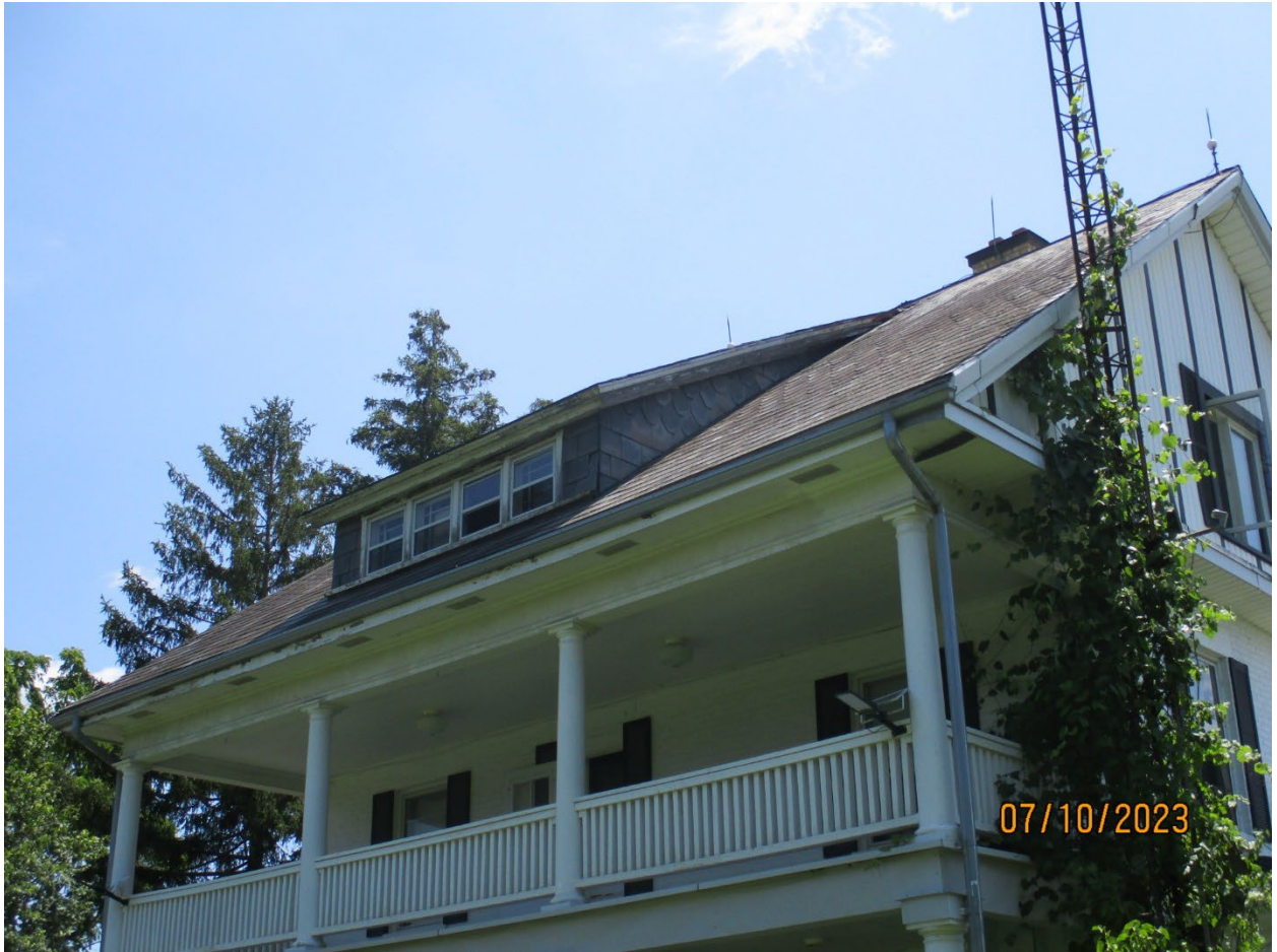
Image 3: Photograph showing the slate roof, second storey porch and shed roof dormer.
