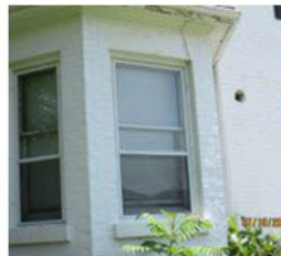
5. One-over-one windows with wood surrounds and wood sills.
