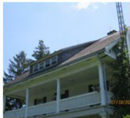
2. Steeply pitched side gable roof with slate cladding, shed roof dormer, two brick chimneys, and concrete chimney.
