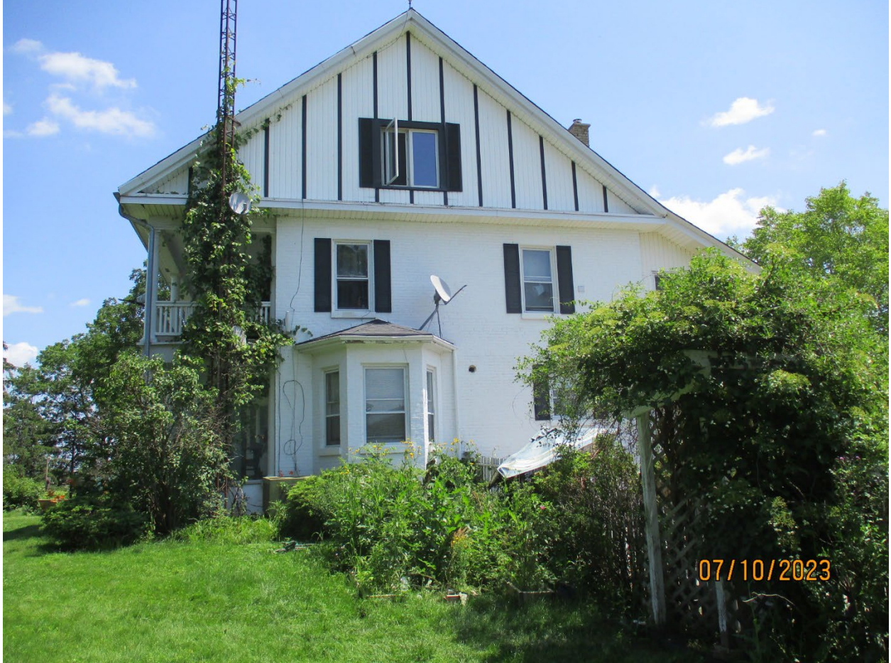
Image 8: Photograph showing the west façade of the Weldwood Farmhouse.
