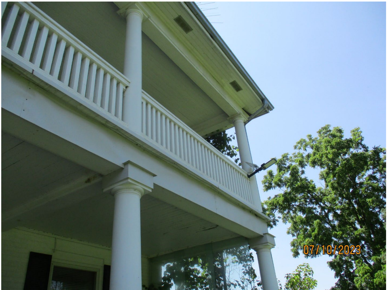
Image 6: Photograph showing the porch and columns details on the Weldwood Farmhouse.
