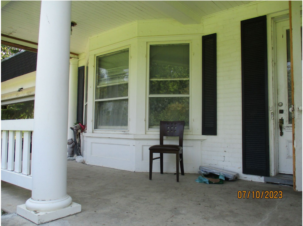
Image 9: Photograph showing the porch, and bay windows on the first storey.
