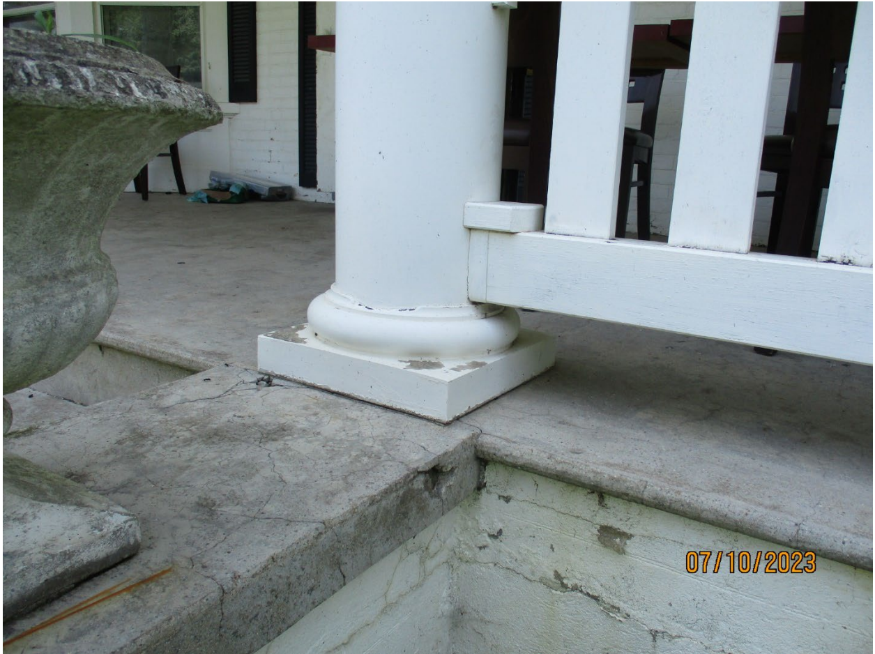
Image 5: Photograph showing the column details on the first storey porch.
