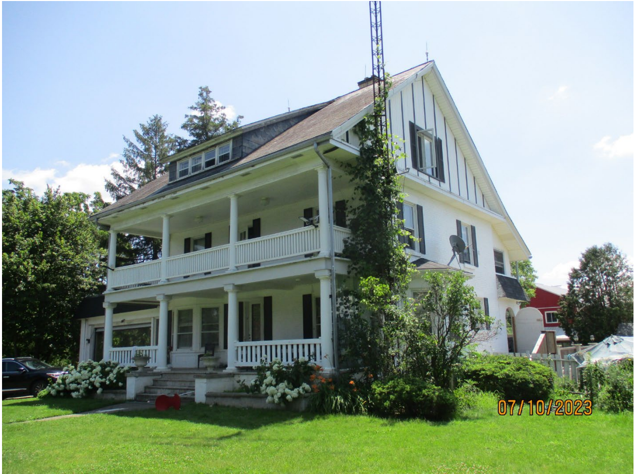
Image 7: Photograph showing the steeply-pitched gable roof of the Weldwood Farmhouse.
