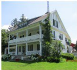
1. Two-and-one-half storey structure with square plan.
