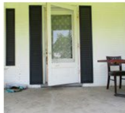
7. Wood and glass storm door and main door on north elevation.
