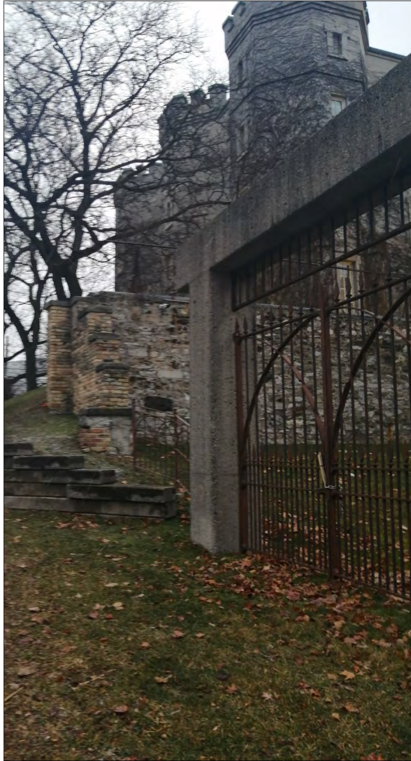
Figure 21: View of masonry wall and cast concrete squared arch along northern property line of jail (MHBC, 2022).
