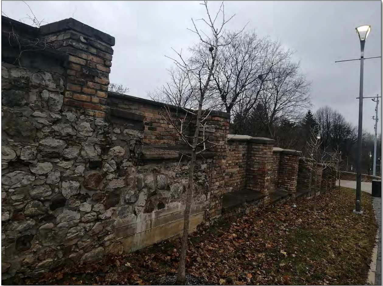
Figure 22: View of masonry wall along northern property line of jail (MHBC, 2022).
