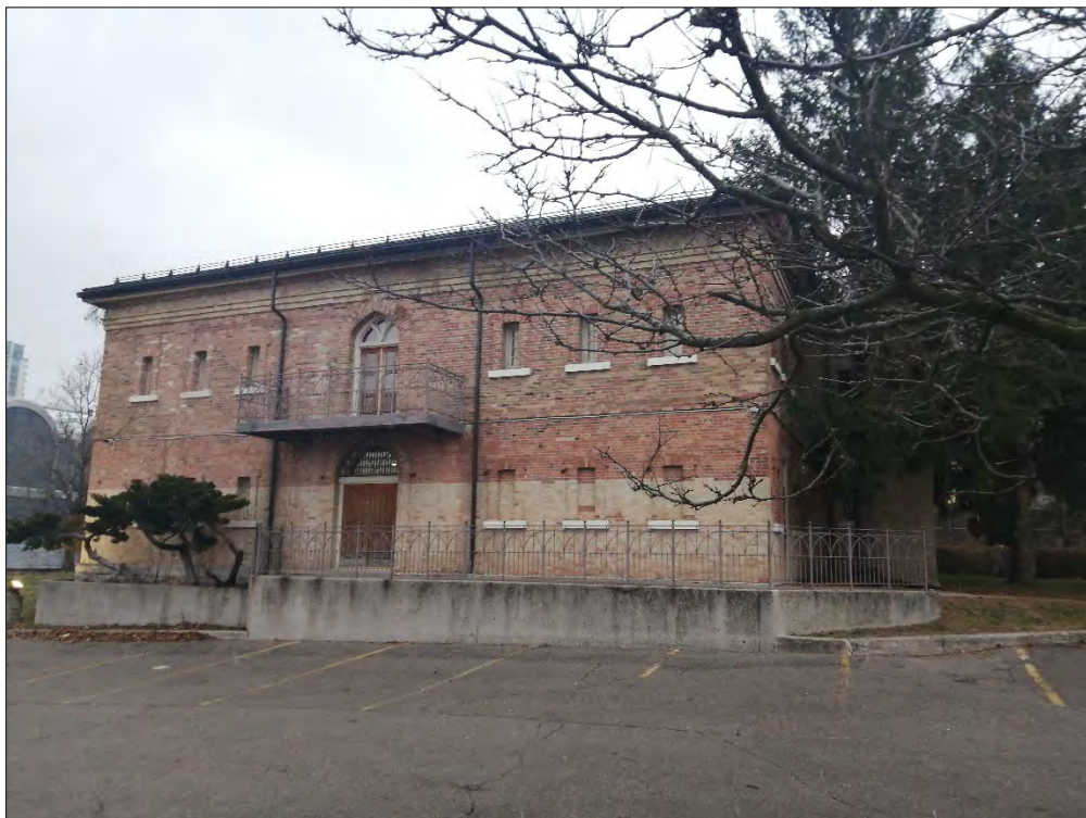
Figures 16 & 17: (above) View of southern elevation of the jail (western half) looking north-east; (below) View of western (rear) elevation of the jail looking eastwards (Source: MHBC, 2022).
