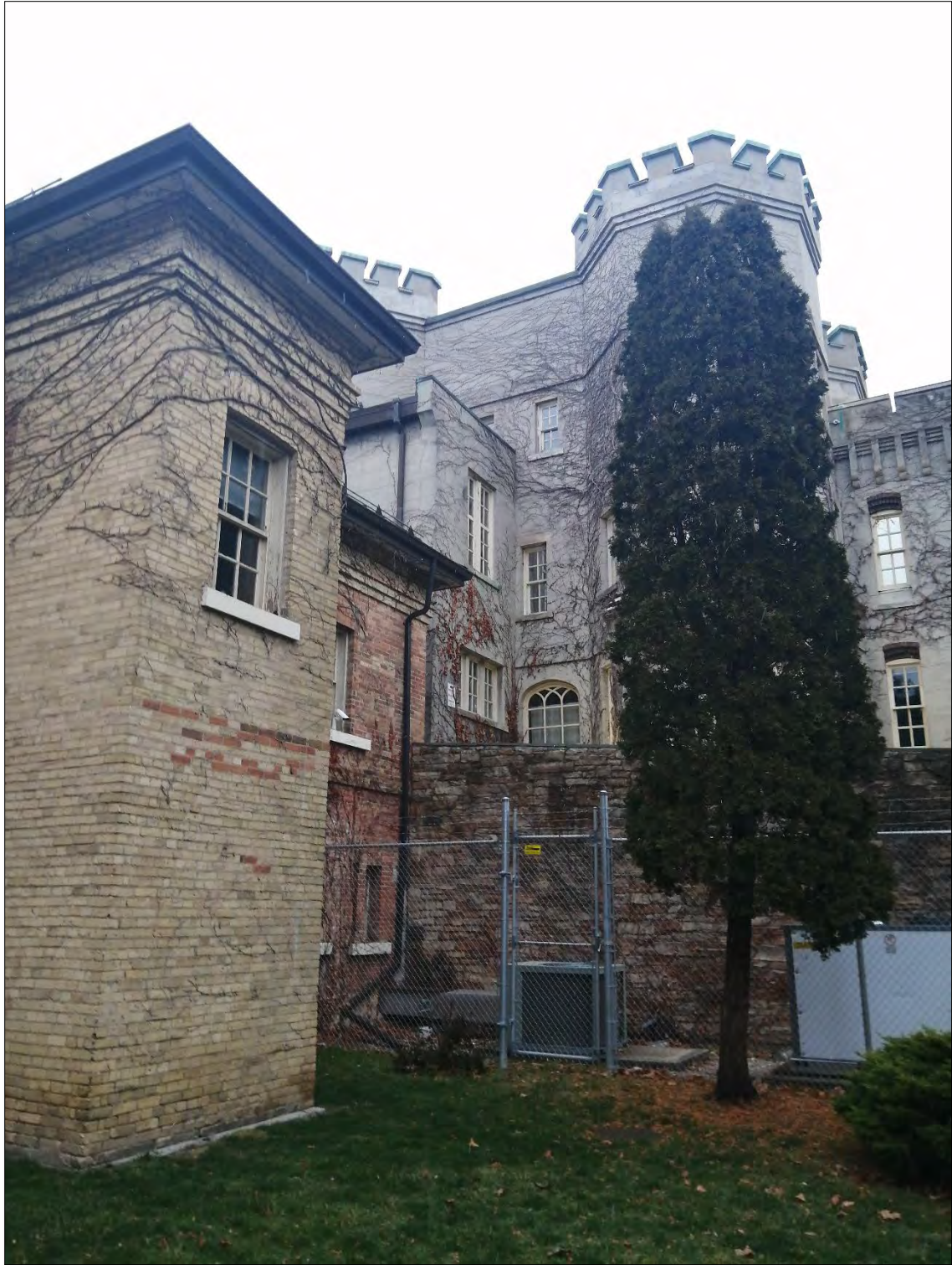
Figure 15: View of south elevation of the jail (eastern half) looking north-west towards courthouse (Source: MHBC, 2022).
