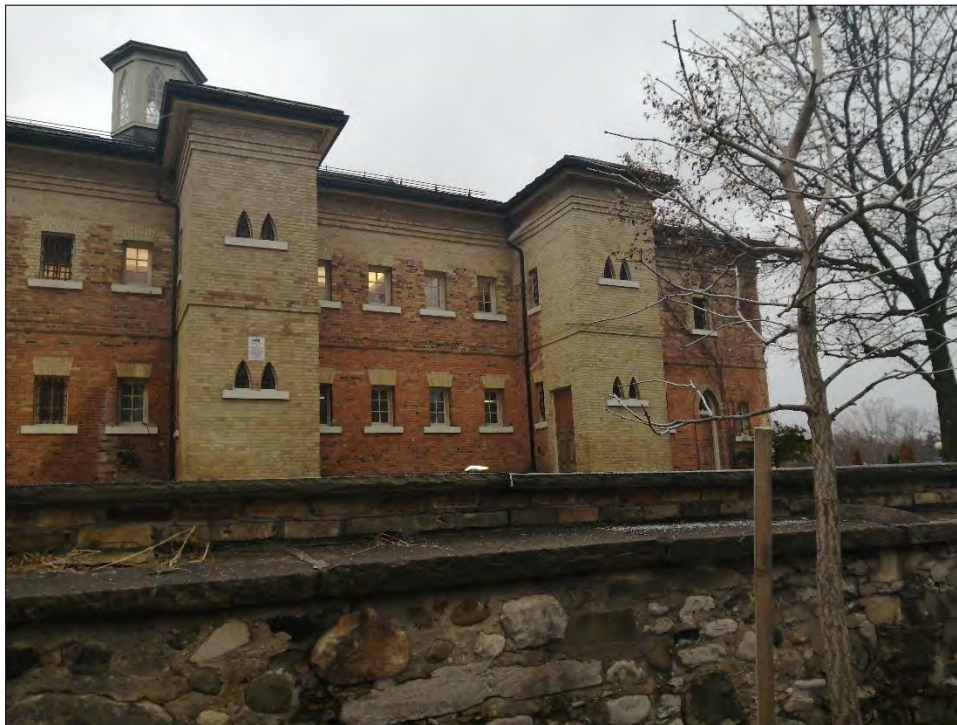
Figures 12 & 13: (above) View of northern elevation of jail (eastern half) looking southwards; (below) View of northern elevation of jail (western half) looking southwards (Source: MHBC, 2022).
