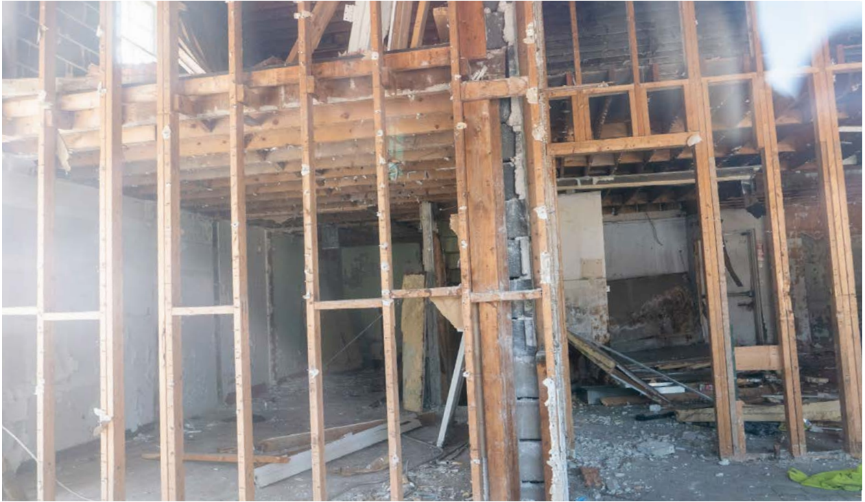
Figure 13: Limited view of the building interior. Note the original concrete block exterior and interior walls (CBCollective 2023).
