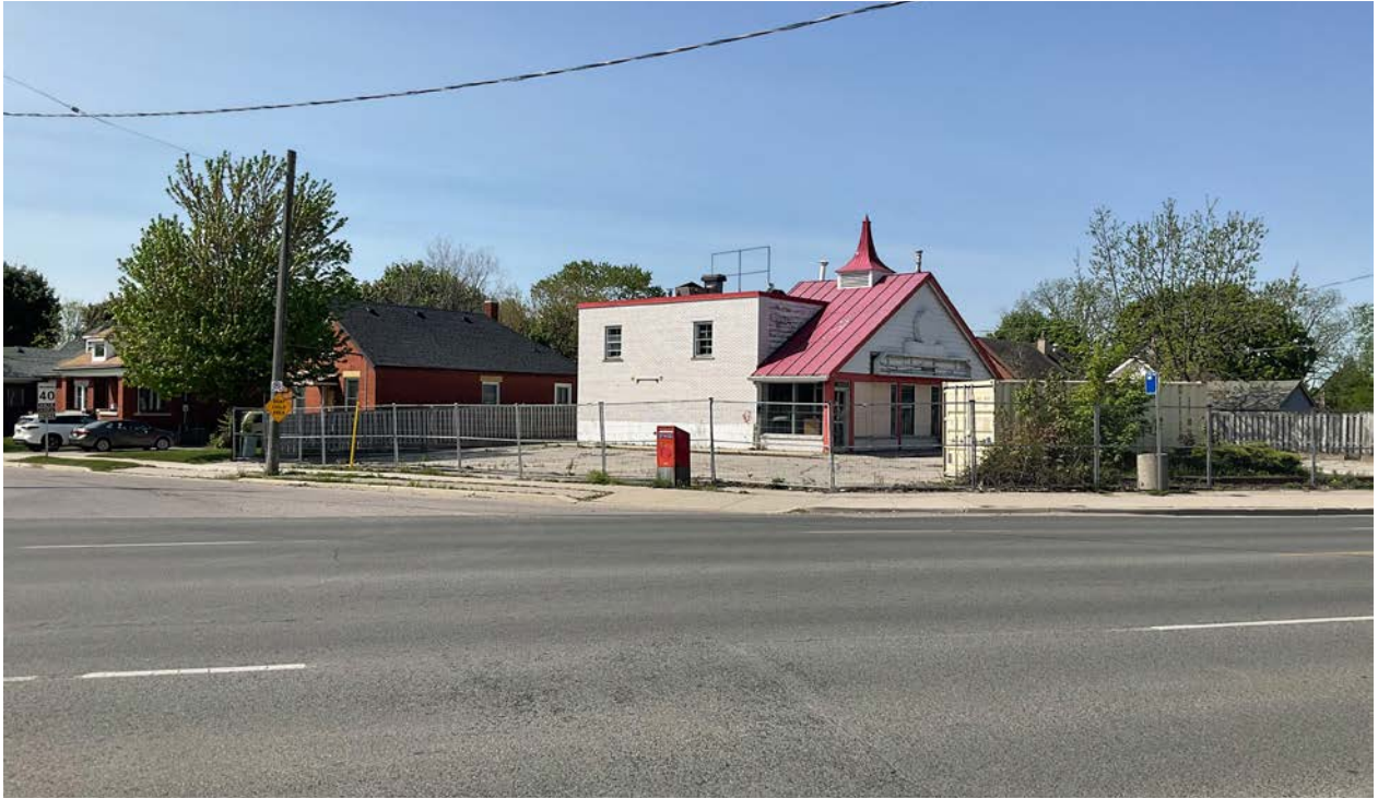
Figure 3: View southwest of the subject property, showing the former restaurant building in the landscape (CBCollective 2023).
