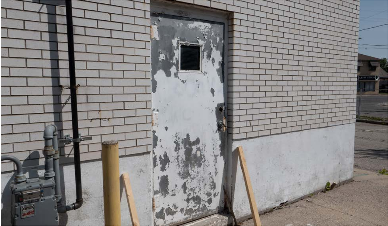
Figure 9: Metal slab door on the south elevation (CBCollective 2023).
