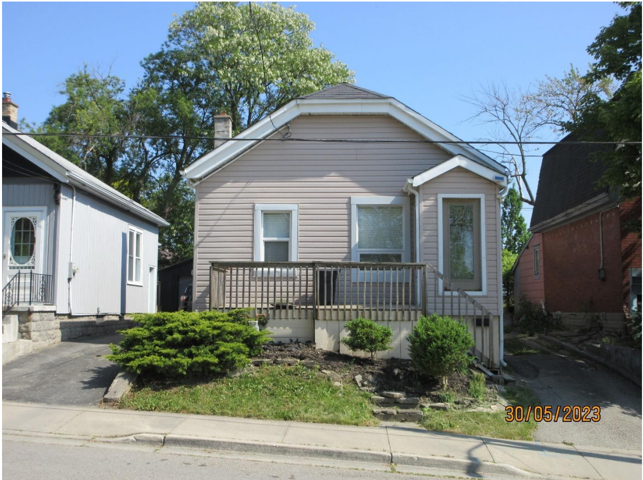
Image 1: Photograph of the dwelling located on the subject property at 2 Kennon Place, May 30, 2023.
