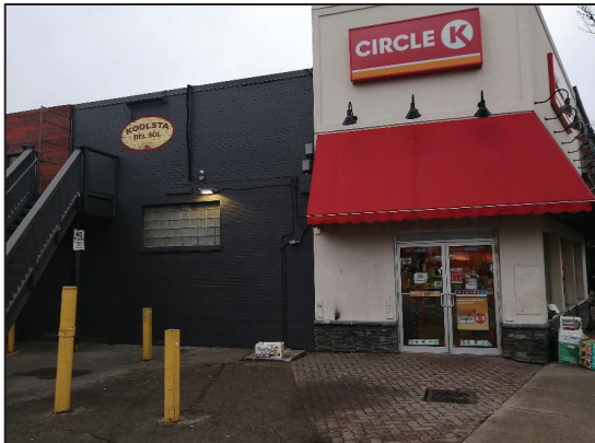
Figure 40: View of right side of the south elevation (Source: MHBC, 2020).
