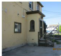
5. Projecting enclosed entry vestibule on the north façade including a) decorative panel door, b) decorative wood door surrounds, and c) arched window on the east and west sides of the entry vestibule.
