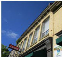
2. Painted brick veneer exterior on the east façade of the building.
