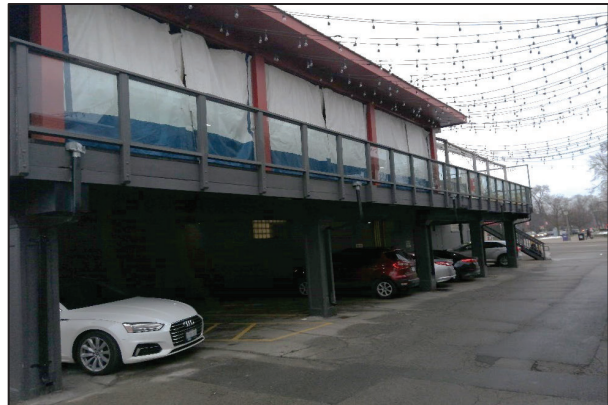
Figure 41: View of verandah along south elevation looking north-east (Source: MHBC, 2020).
