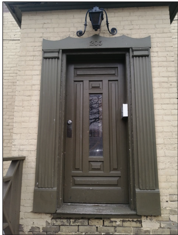
Figure 35: View of front door entryway of portico (Source: MHBC, 2020).
