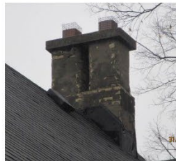
5. Chimney on the north gable, originally paired with a chimney on the south gable (not extant)
