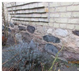
11. Fieldstone foundation walls
