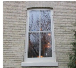
8. Exceptionally large (7 feet in height), two-over-two wood windows, with wood storm windows, on the main floor
