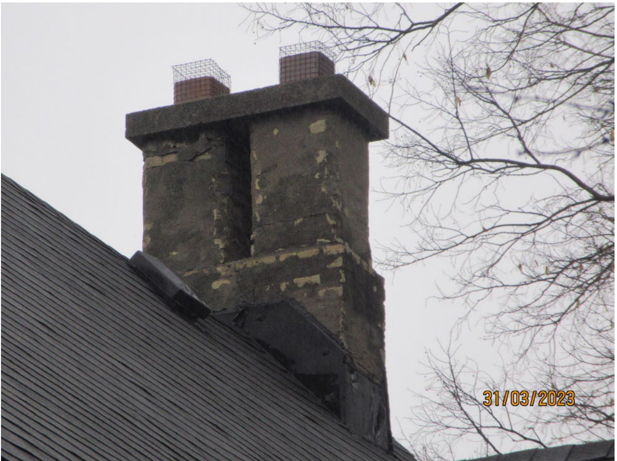
Image 8: Chimney on the north gable.
