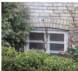
9. Basement window openings
