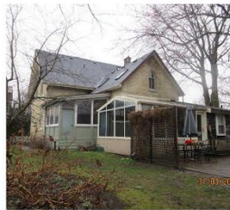
2. T-plan of the building, with the main block (front) built in c.1865-1866 and the back wing built in c. 1854-1862
