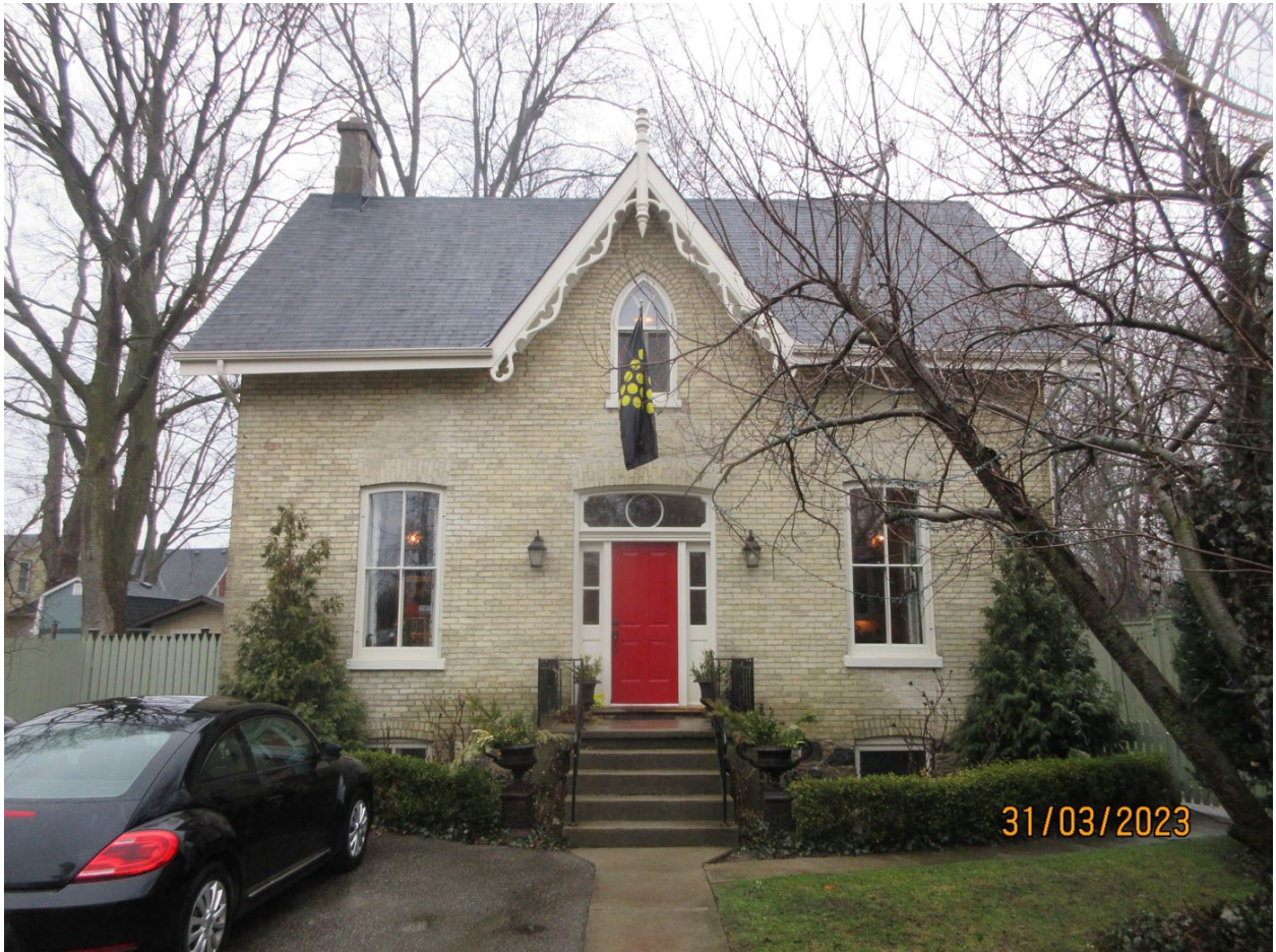
Image 1: Photograph of the main elevation of the main block of the house.
