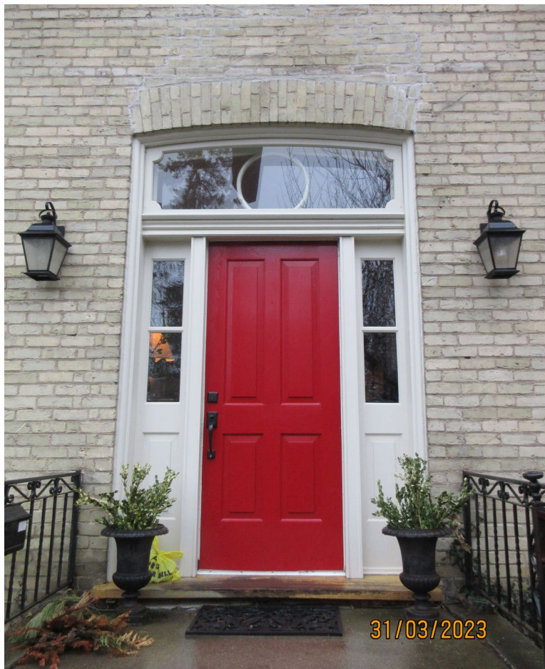
Image 2: Front entranceway with pair of divided sidelights flanking central door.
