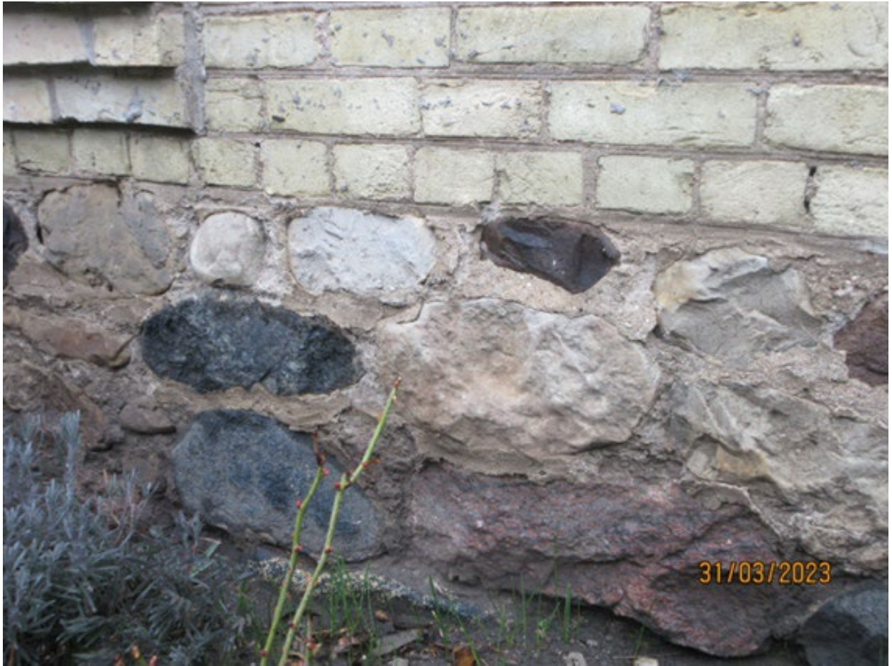
Image 9: Fieldstone foundation wall on the west elevation.
