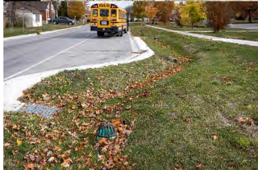
Wellington Road Exfiltration System (2019); East Lions Park (2020)
