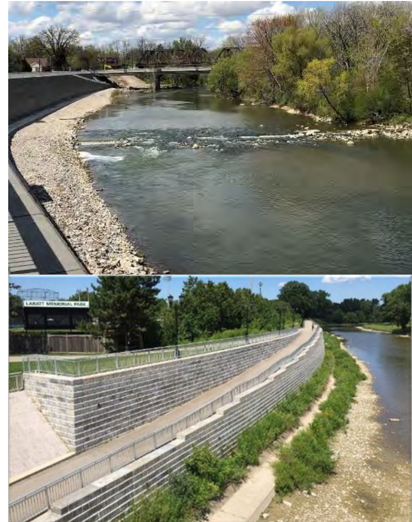
West London Dyke Reconstruction
