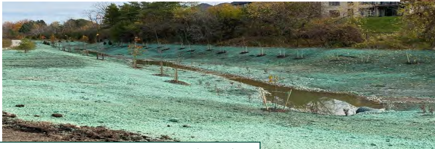
Powell Drain Reconstruction (2020)
