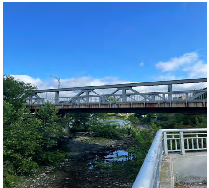
Photograph 8. ↑ View of North Thames River and Kensington Bridge
