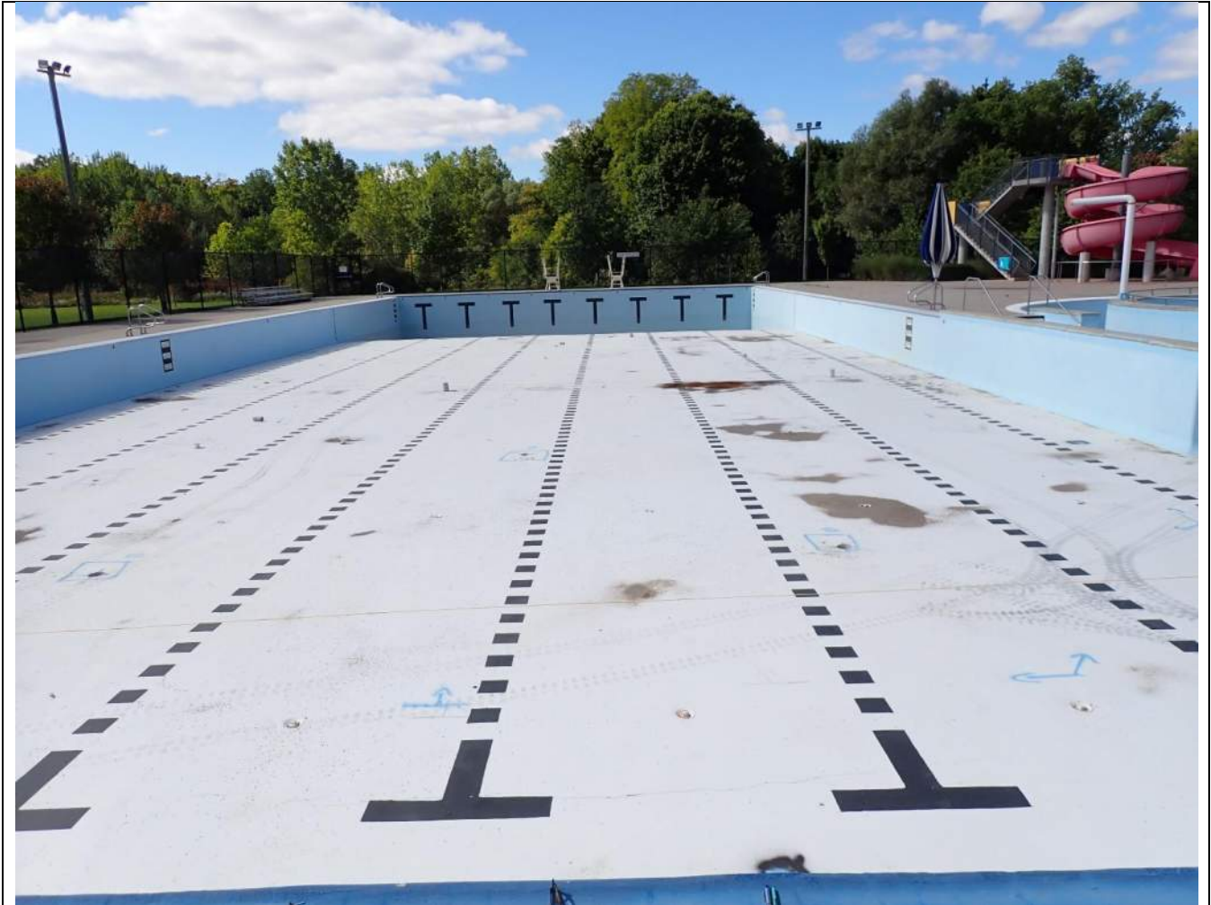
PHOTOGRAPH 1: Overview of Eight(8) Lane Lap Pool
