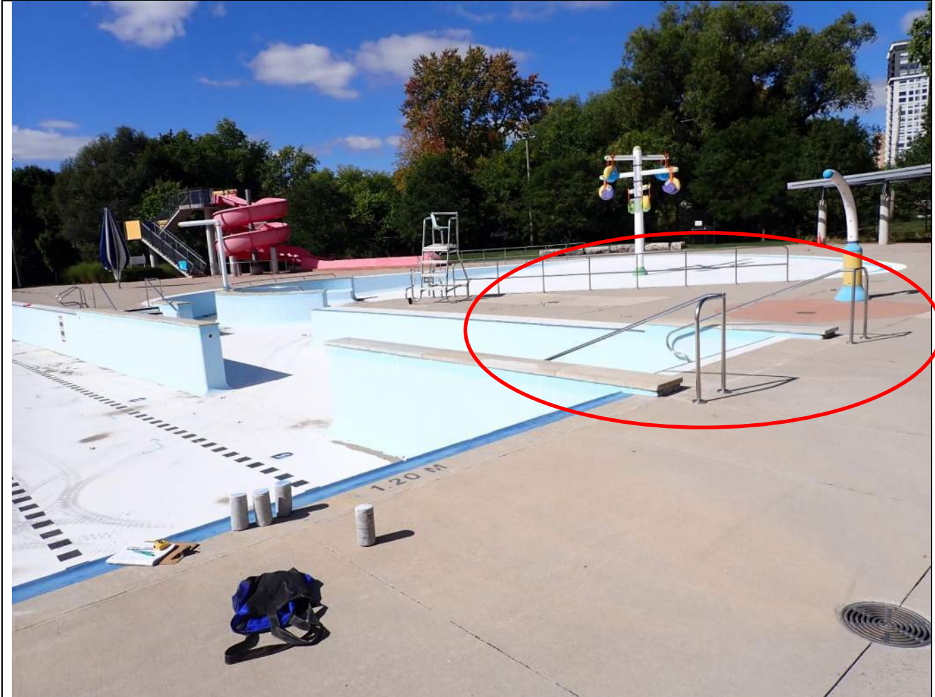
PHOTOGRAPH 5: Stainless Steel railing appears sound
