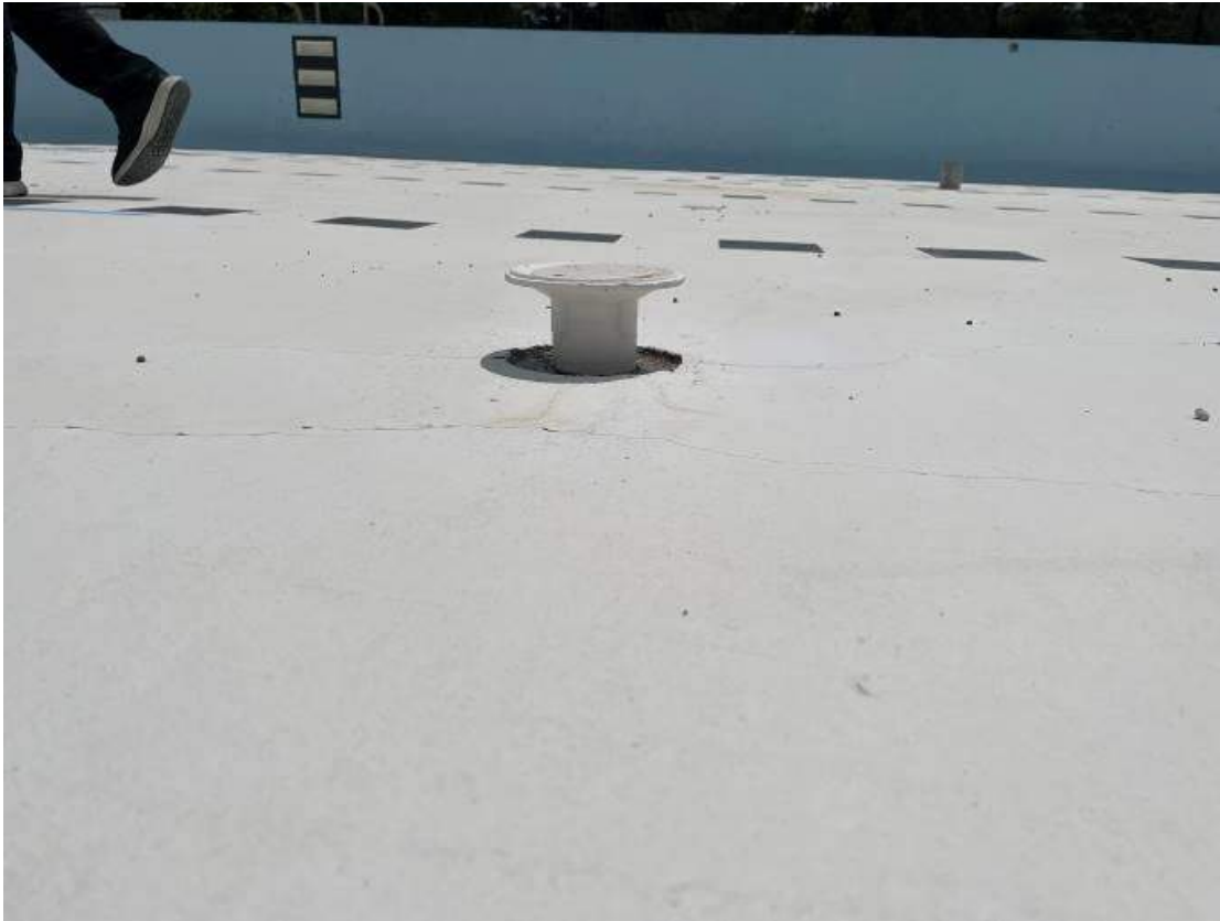
Figure 7, Report I – Preliminary Review – Floor return protruding from pool floor, June 2022
