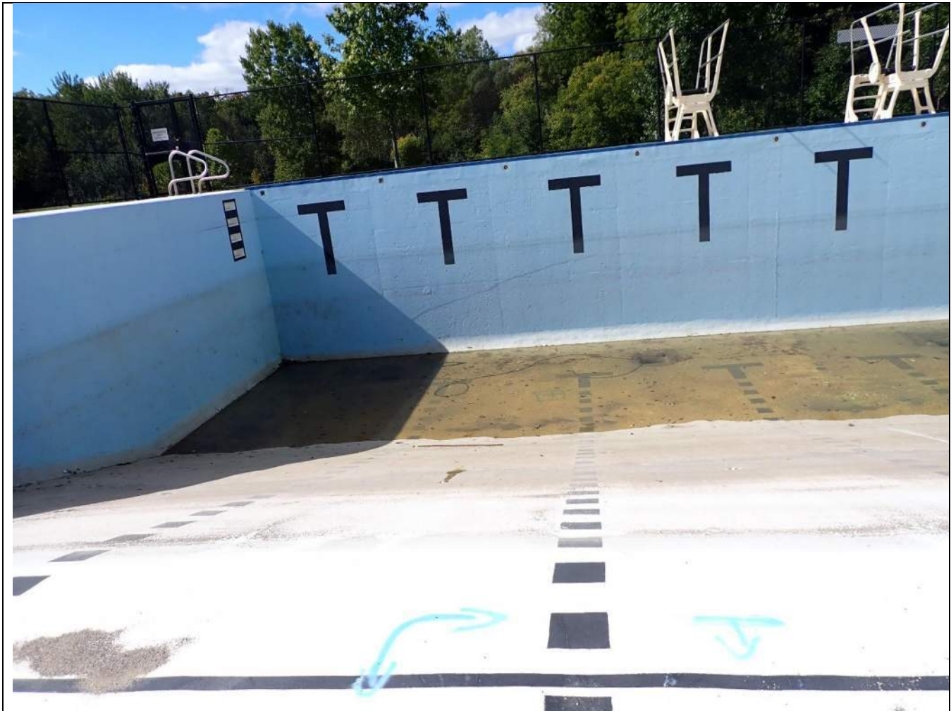
PHOTOGRAPH 2: Closeup of deep end of Lap Pool
